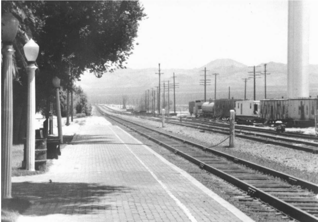
History #7: Brick station platform, looking east. (PGSO, Collection of Art Francis, ca. 1960)
