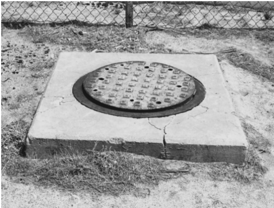
Small Scale Features #7: Concrete shaft with manhole cover. (PGSO, CLI negative #MOJA-N-0005-25, 1999)
