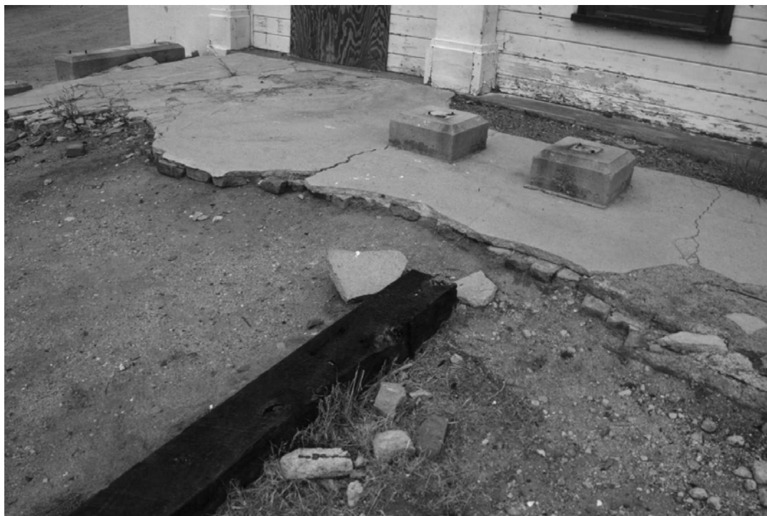
Circulation #8: Concrete walkway, west side of depot, looking east. (PGSO, CLI slide #MOJA-S-0002-22, 1999)
