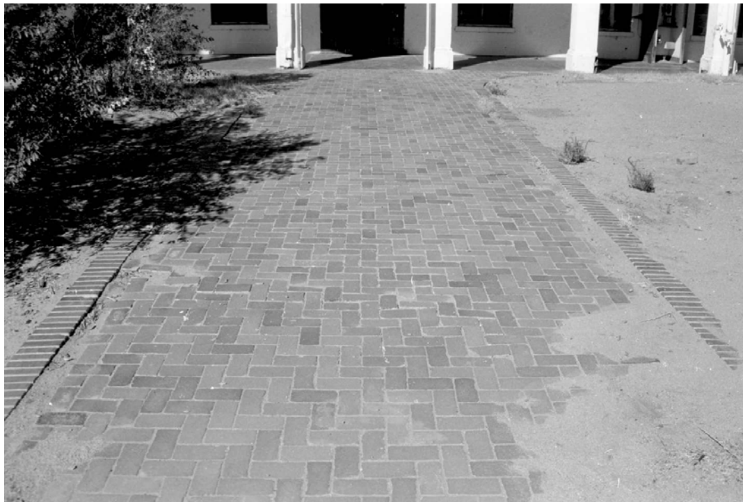
Circulation #4: Herringbone pattern on brick walkway, looking north. (PGSO, CLI negative #MOJA-N-0010-22, 1999)
