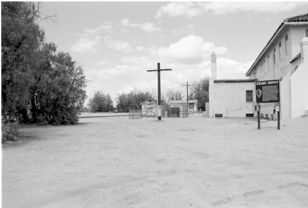
Small Scale Features #8: Utility poles, looking east. (PGSO, CLI negative #MOJA-N-0001-8, 1999)
