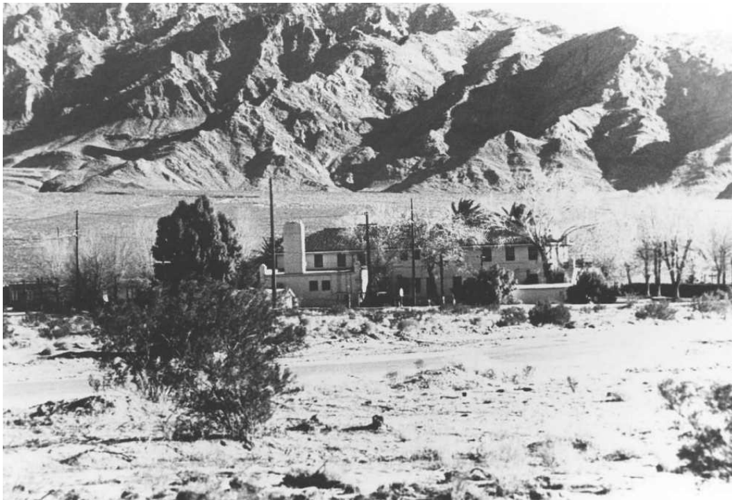
Views and Vistas #1: Rear of depot with Providence Mountains in the background. (PGSO, Parks and Snyder, 1975)
