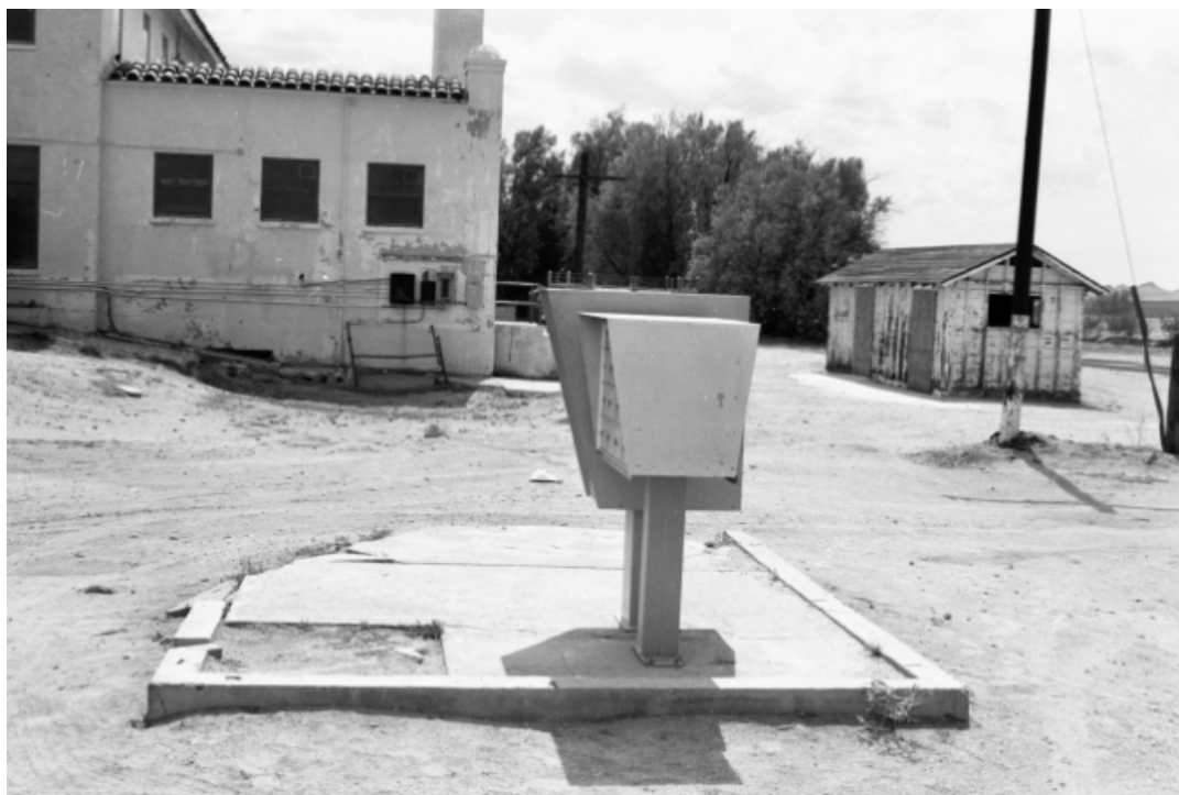
Archeology #3: Shower building foundation, looking west. (PGSO, CLI negative #MOJA-N-0007-5, 1999)
