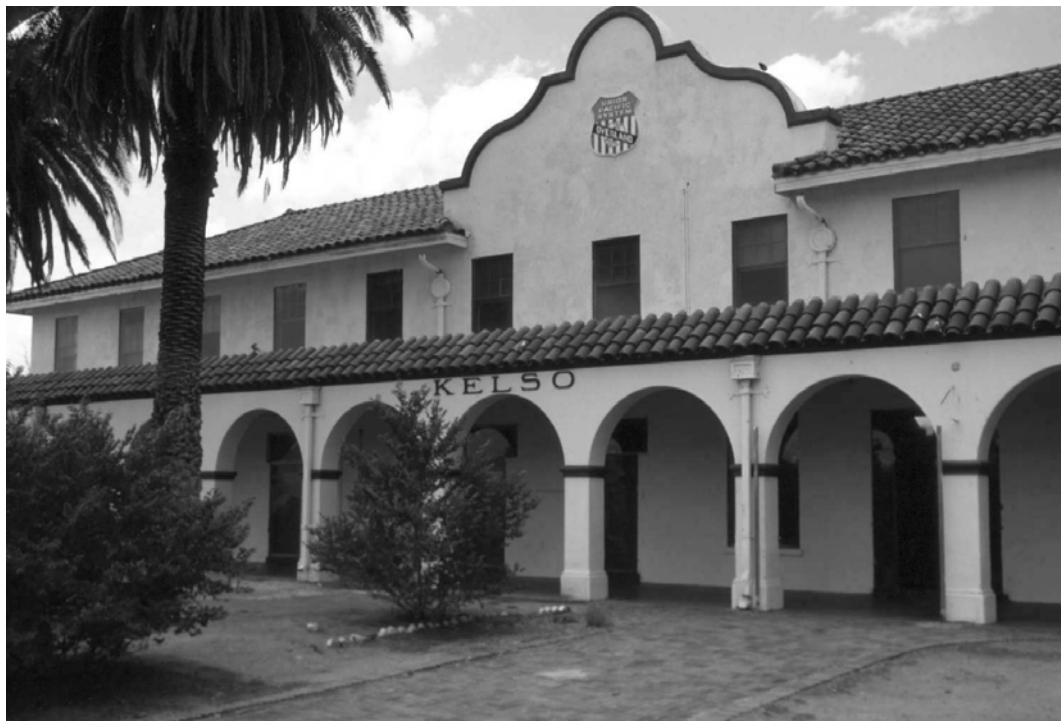
Circulation #2: Kelso Depot arcade and brick walkway, looking north. (PGSO, CLI slide #MOJA-S-0002-18, 1999)
