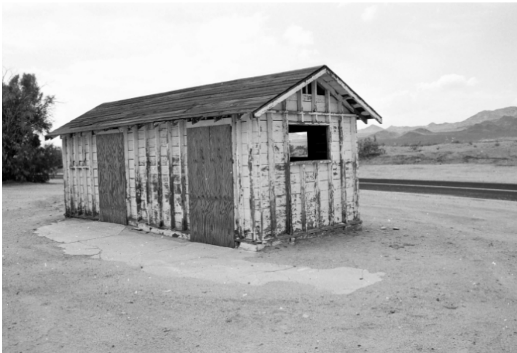
Buildings and Structures #3: Coal Shed and concrete walkway, looking west. (PGSO, CLI negative #MOJA-N-0005-21, 1999)
