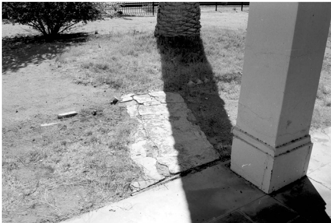
Circulation #7: Concrete walkway, looking south. (PGSO, CLI negative #MOJA-N-0009-05, 1999)
