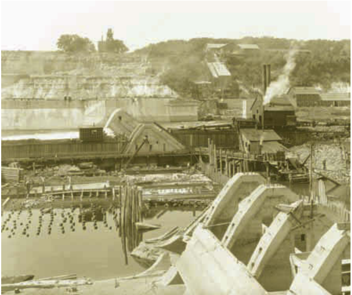
Lock and Dam No. 1, showing innovative prefabricated design that allowed for cold-weather construction, nearing completion, 1916
