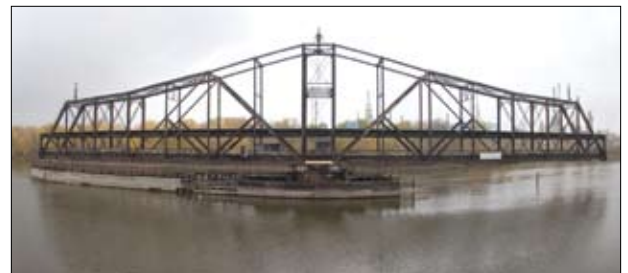
The Rock Island Swing Bridge carried rail and vehicular traffic between Inver Grove Heights and St. Paul Park. (NPS)
