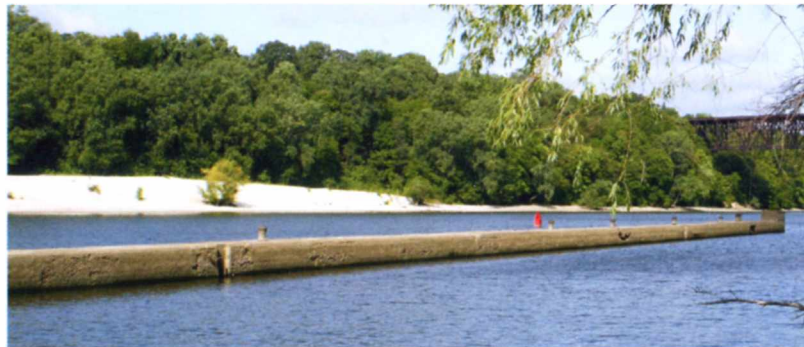
Meeker Island lock wall. (NPS)
