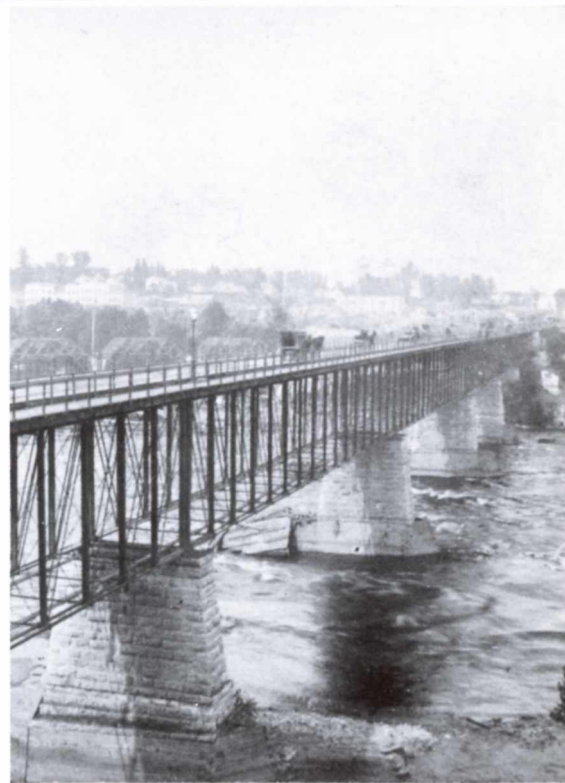
Tenth Avenue Bridge Across the Mississippi, circa 1885. (Minnesota Historical Society)
