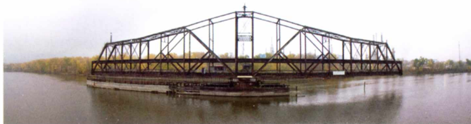
Rock Island Swing Bridge. (NPS)
