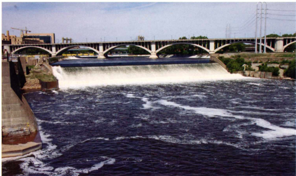
St. Anthony Falls, Minneapolis. (NPS)
