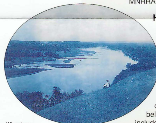
Wingdams Below Nininger, Minn., 1891, by Henry Bosse, U.S. Army Corps of Engineers. Through his cyanotype photographs, Bosse captured the early reshaping of the river's natural landscape by the Corps of Engineers. (Photo courtesy U.S. Army Corps of Engineers)
