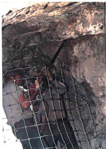
CABLE NET AT STATE OF TEXAS MINE IN CORONADO NM. CONSTRUCTED AND IN- STALLED BY DEATH VALLEY NM STAFF. COST AVERAGES $1,250 PER NET.
