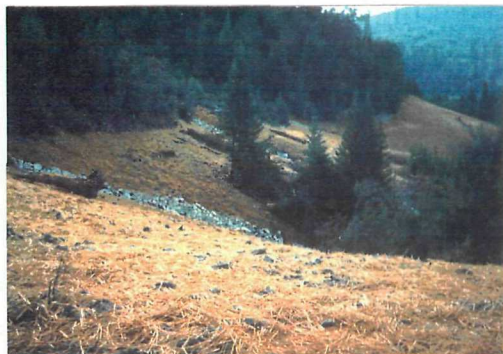
RECLAIMED TIMBER HAULAGE AND QUARRY ACCESS ROAD IN REDWOOD NP. RECLAMA- TION OF THIS ROAD COST $189,000/MI. SMALLER ROADS COST AS LITTLE AS $11,000/MI.
