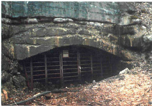
BAT GATE IN NEW RIVER GORGE NR DESIGNED TO ADMIT RARE BATS
