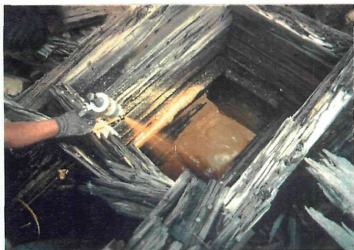
INSTALLING A POLYURETHANE FOAM PLUG. COSTS VARY FROM $1,000 TO $31,000 DEPENDING ON SIZE, ACCESS AND SITE CONDITIONS.
