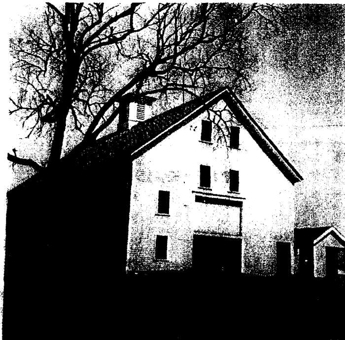
Figure 5 Front and west elevations of the barn, April 1963.
