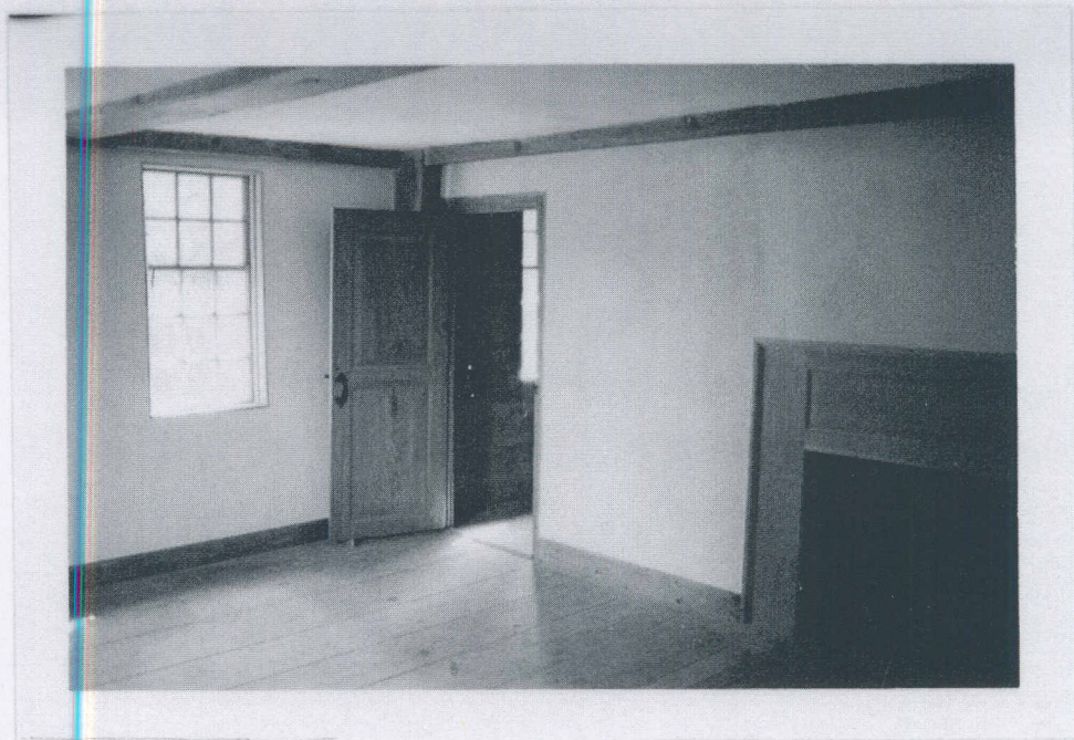
Southwest corner of the East Chamber with an original two paneled door and thumb latch. Mantelpiece is a reconstruction.
