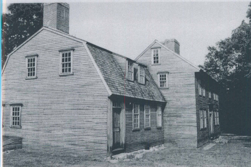
View of Hartwell Tavern looking northeast at restored exterior completed in 1981-82. Window frames and doorway in south wall of c. 1783 gambrel addition are original.
