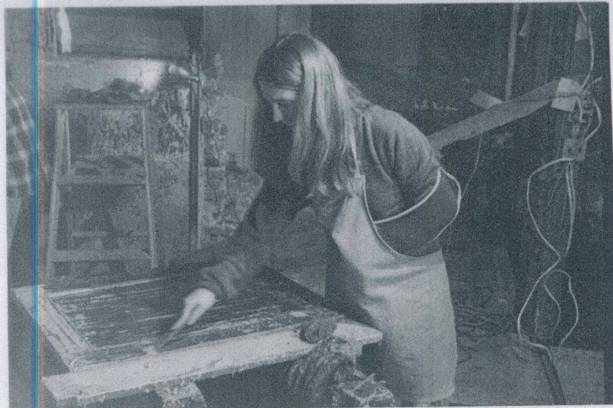
Kathy Thompson removing paint from a cupboard door in the West Parlor. In order to give the public the effect of an unpainted tavern room in 1775, paint was removed from later additions to the West Parlor, such as this cupboard door added in ca. 1830.
