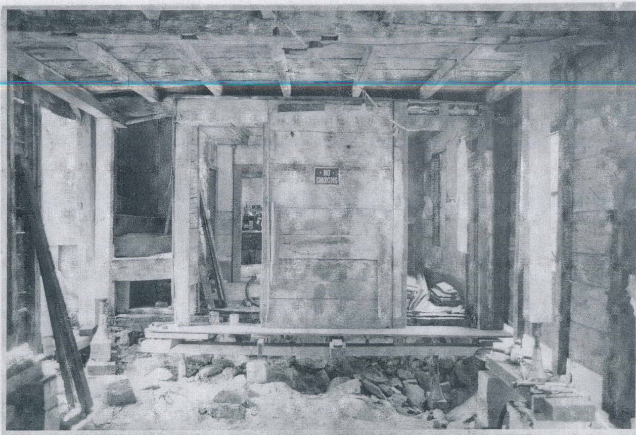
Interior view of the shed during rehabilitation work on the floors and stairway. View looking south with gambrel addition beyond.
