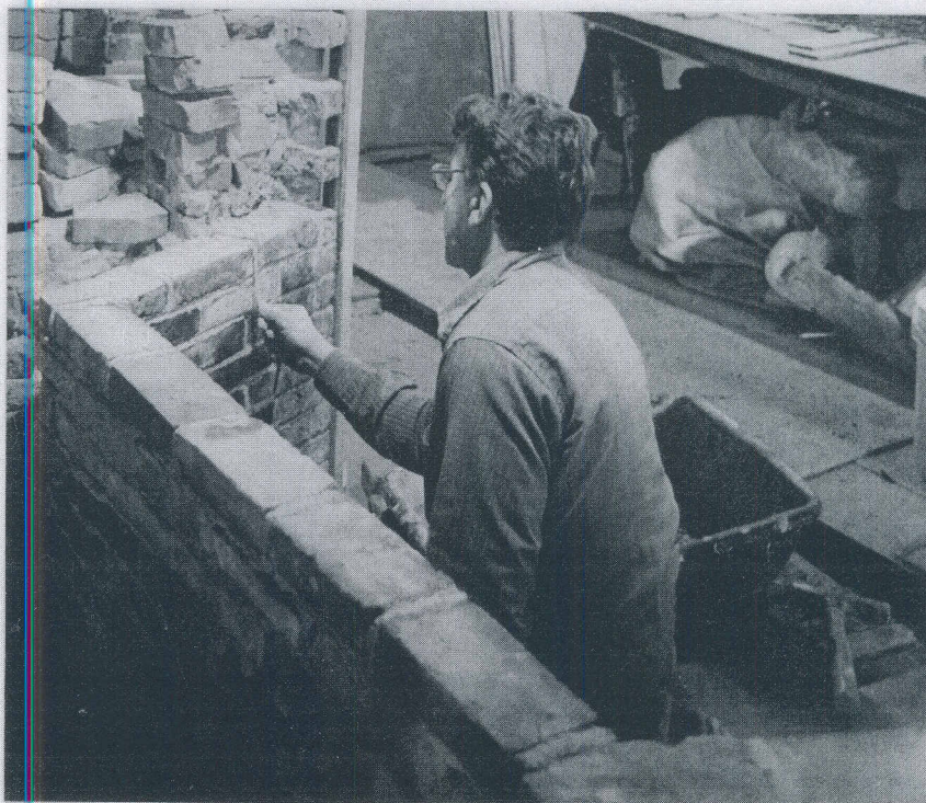
R. Boucher shown rebuilding the fireback and jambs for the fireplace in the Kitchen of the lean-to.
