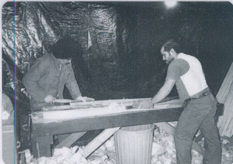
Pablo Cuevas and Pedro Deleon are shown smoothing the rough clapboard stock into clapboards. The use of a long-handled slick proved to be a more efficient way of removing the excess wood than the traditional use of a draw knife.
