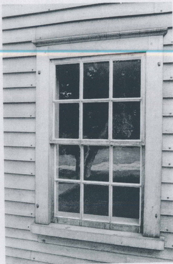
Reconstructed window frame and sash c. 1830 period.
