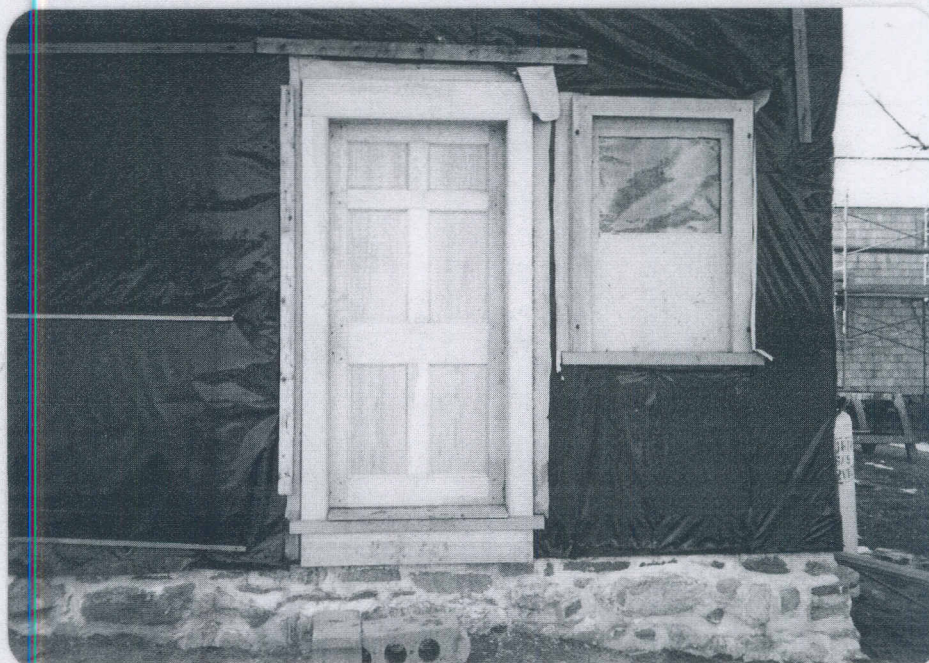
East wall of the kitchen lean-to showing the recently installed door frame and door along with a new adjoining window frame. These members represent one of several architectural styles in use during the first half of the 19th century.
