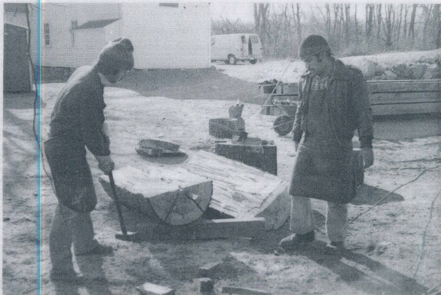
Michael Smith and Pedro Deleon split five feet long white pine logs into clapboard bolts. Photo: NPS, M. Fortin, February 1980
