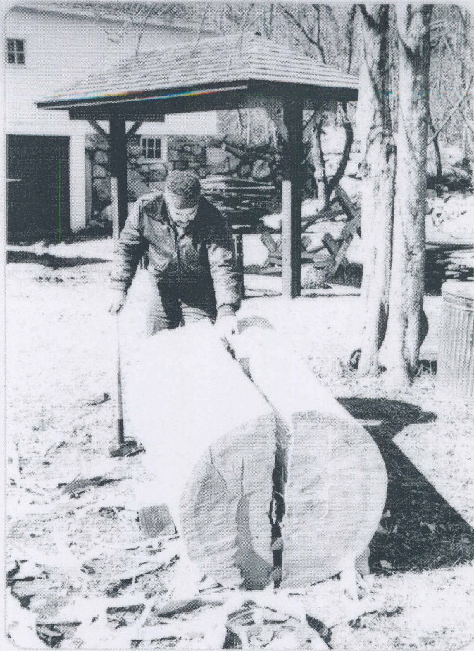
Pedro Deleon debarks and splits a white pine log on the first step toward making clapboards. Photo: NPS, M. Fortin, March 1981
