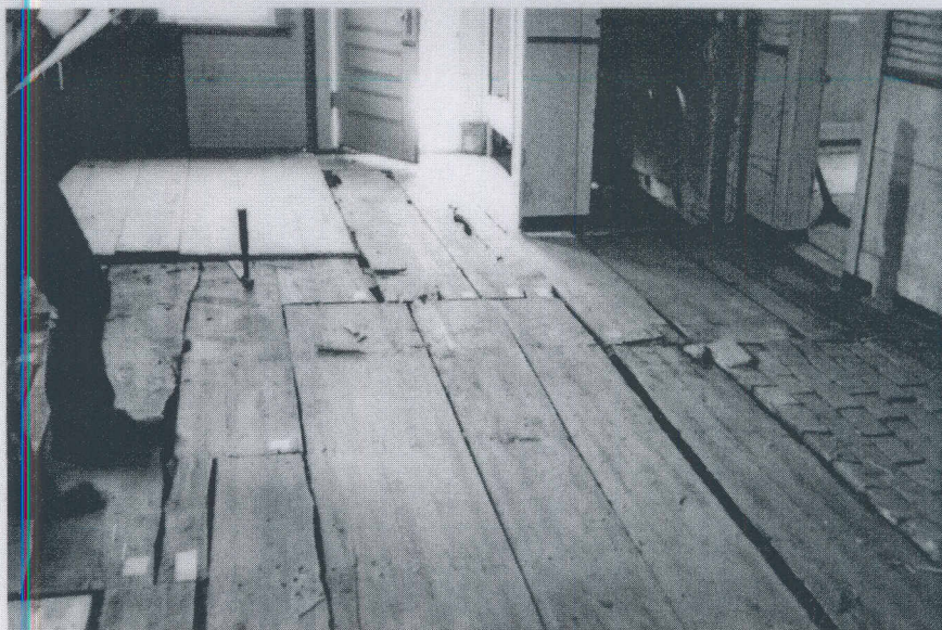
Original floor boards in the Kitchen lean-to. The six finish floor boards seen in the upper left hand corner are original to a small room once located here. The remaining boards are from the original sub-floor of ca. 1830. Kitchen hearth dates from c. 1830 and was taken up and relaid in 1981.
