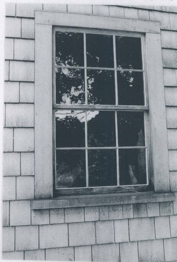
Window frame representing the 1865 period when the first exterior changes were made to shed of c. 1830.
