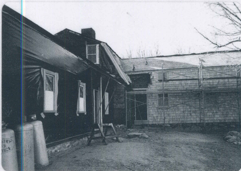
By early winter of 1981, the roofs had been shingled, exterior window and door frames installed and work on the shed addition nearly completed. View at rear of Hartwell Tavern.
