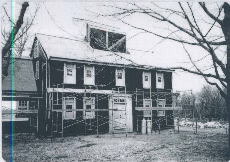
South wall of the Hartwell Tavern after the reproduction (1733) window frames and fronticepiece for the central doorway had been installed. The temporary tent structure seen on the roof provided protection to the brick mason while the central chimney was being built.
