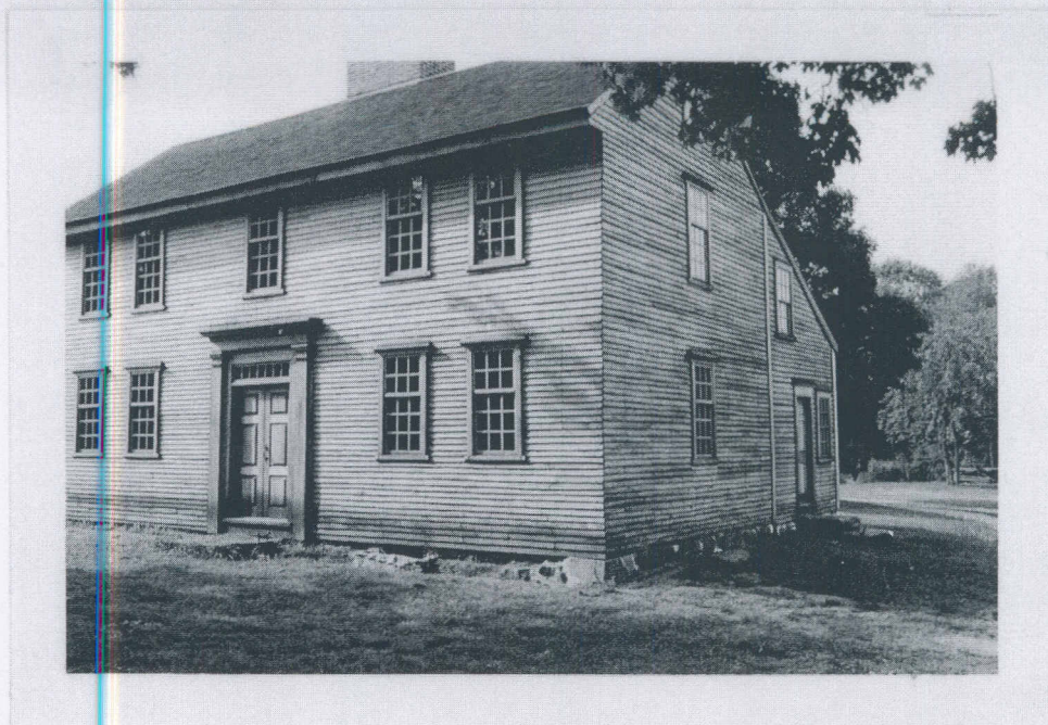
Exterior view of 1733 house as restored in 1981-82. All woodwork replaced was reproduced from white pine.
