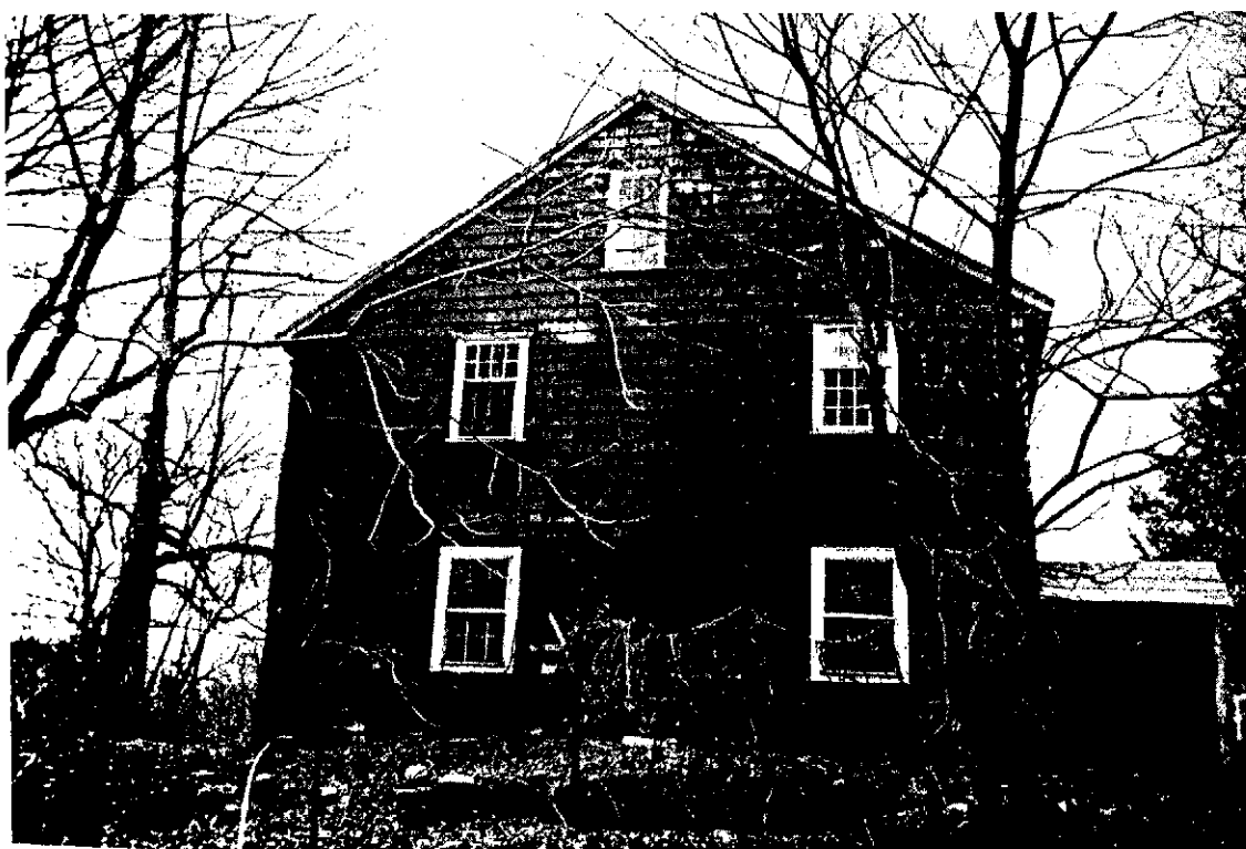
Figure 17. East elevation, April 2002.
