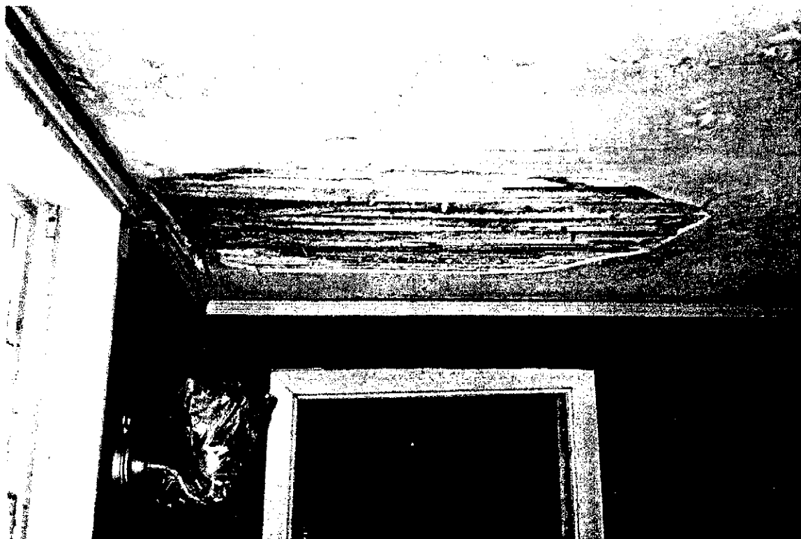
Figure F-2. Missing/damaged plaster ceiling, upper hall (Room 202).
