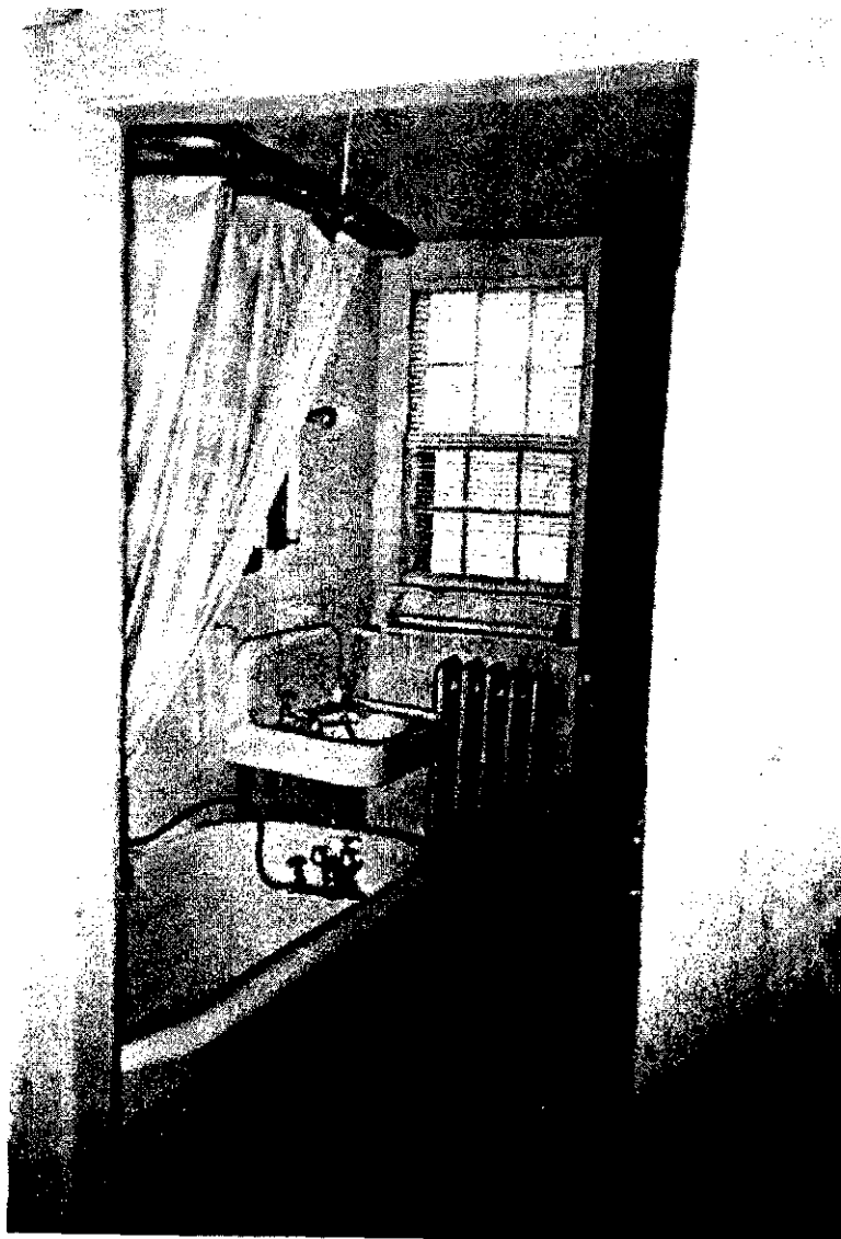
Figure 44. Bathroom (Room 205): view looking northwest, April 2002.
