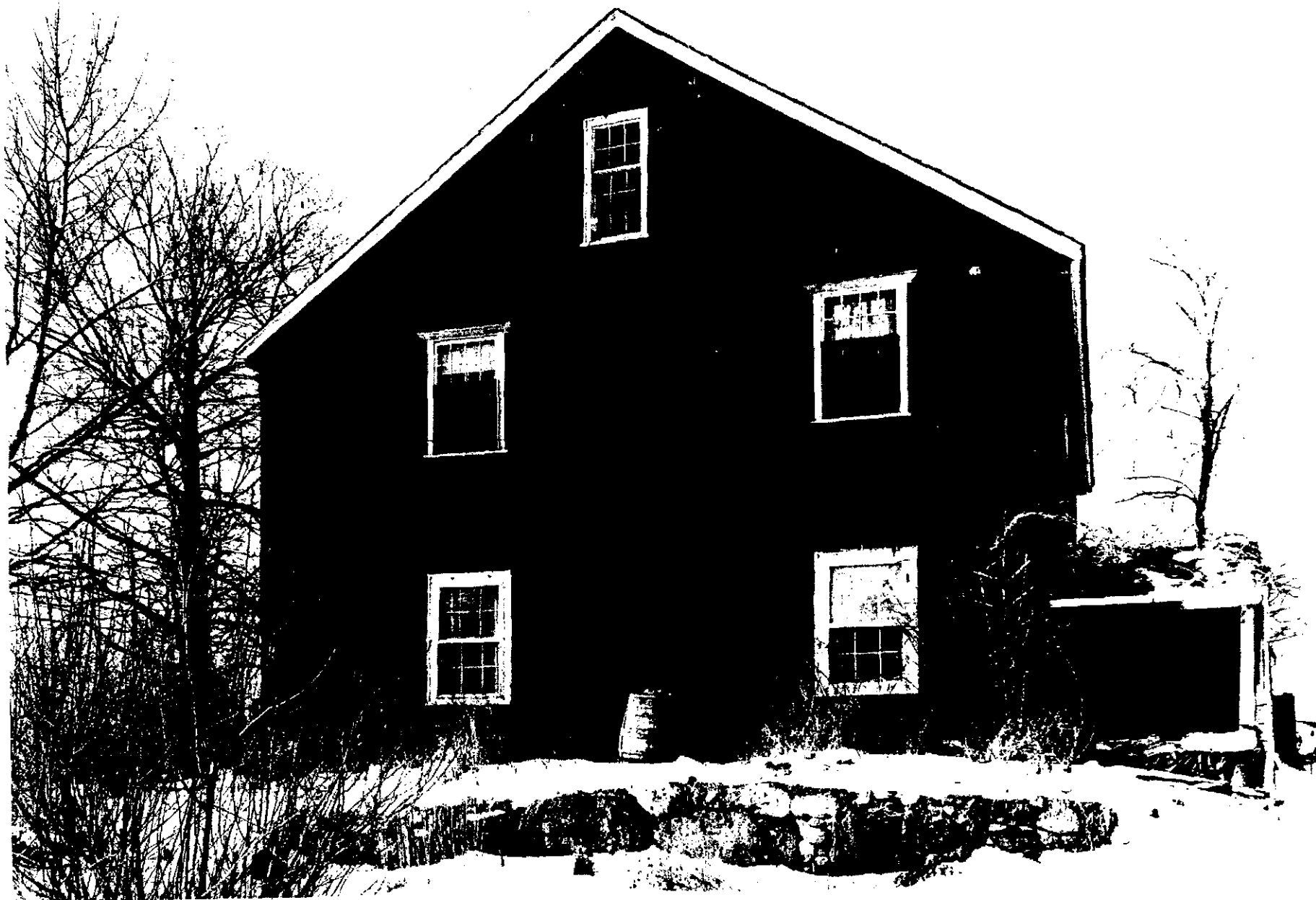
Figure 7. Olive Stow House: east elevation, February 1963.
