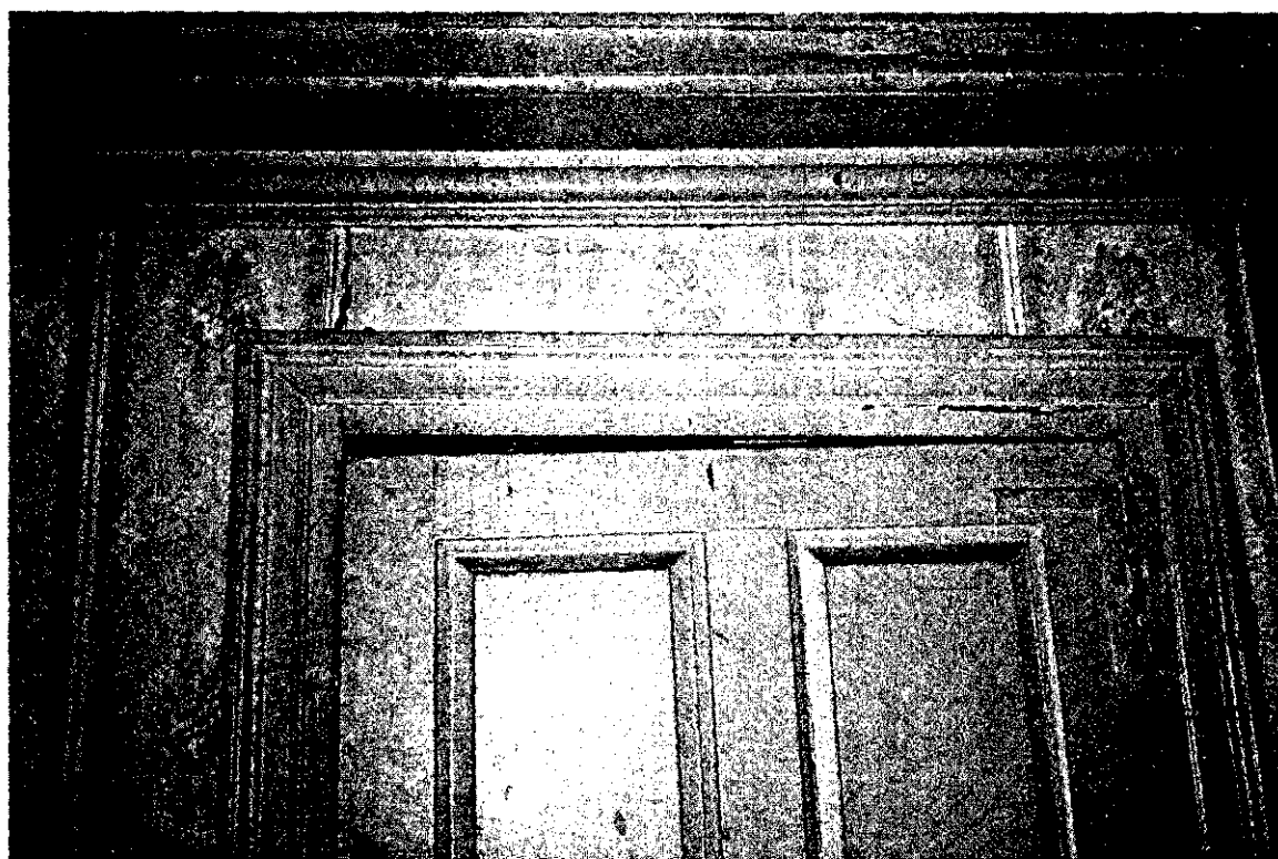
Figure F-9. Out-of-level door frame, east doorway of the southwest room (Room 101).
