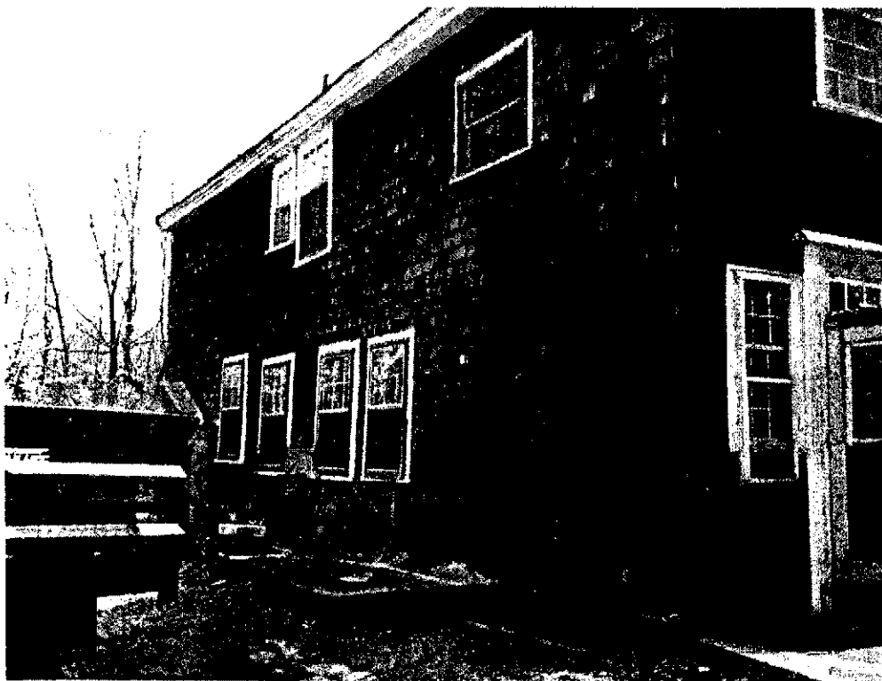
Figure 16. Rear (north) elevation, April 2002.
