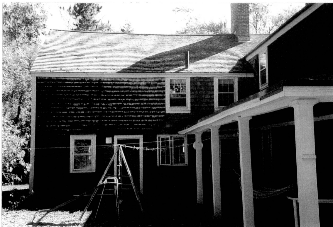
Figure 39. Gowing-Clark House – Ell, West Wall (1999).
