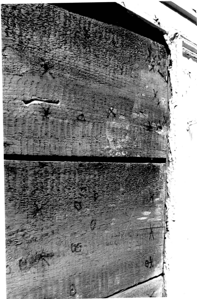
Figure 13. Gowing-Clark House – South Façade, West End, Detail Showing Original Mill-Sawn Sheathing (1999).
