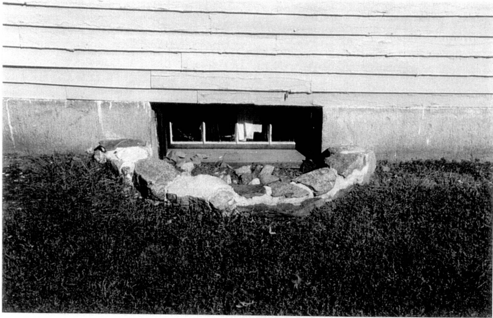
Figure 51. Gowing-Clark House – Main House South Façade, Window W001 (1999).
