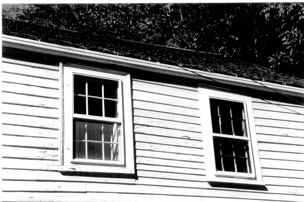
Figure 56. Gowing-Clark House – Ell East Wall, Windows W208 & W209 (1999).
