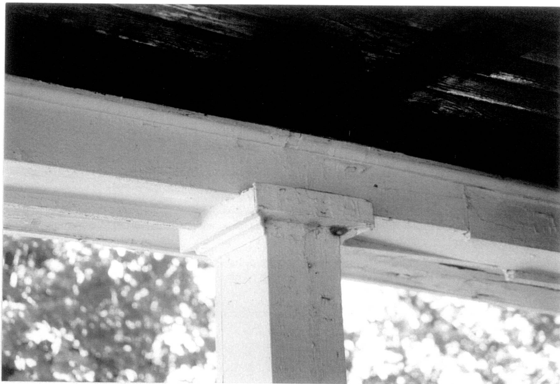
Figure 68. Gowing-Clark House – West Porch, Post Cornice Detail (1999).
