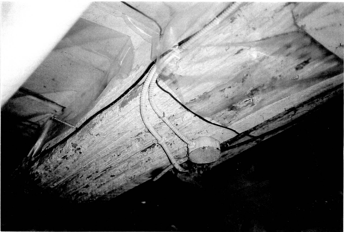
Figure 18. Gowing-Clark House – Ell Cellar, Reused Timber as North/South Girt (2000).
