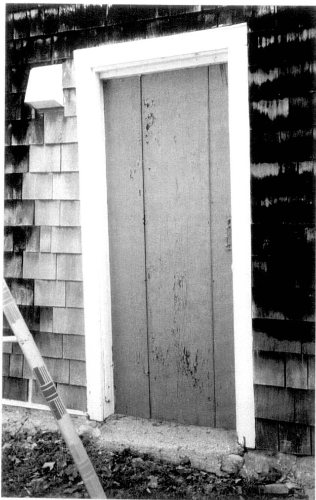
Figure 47. Gowing-Clark House – Ell West Wall, Doorway D104 (1999).
