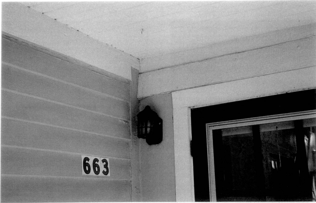
Figure 41. Gowing-Clark House – Junction of Ell South Wall with Main House East Wall (1999).
