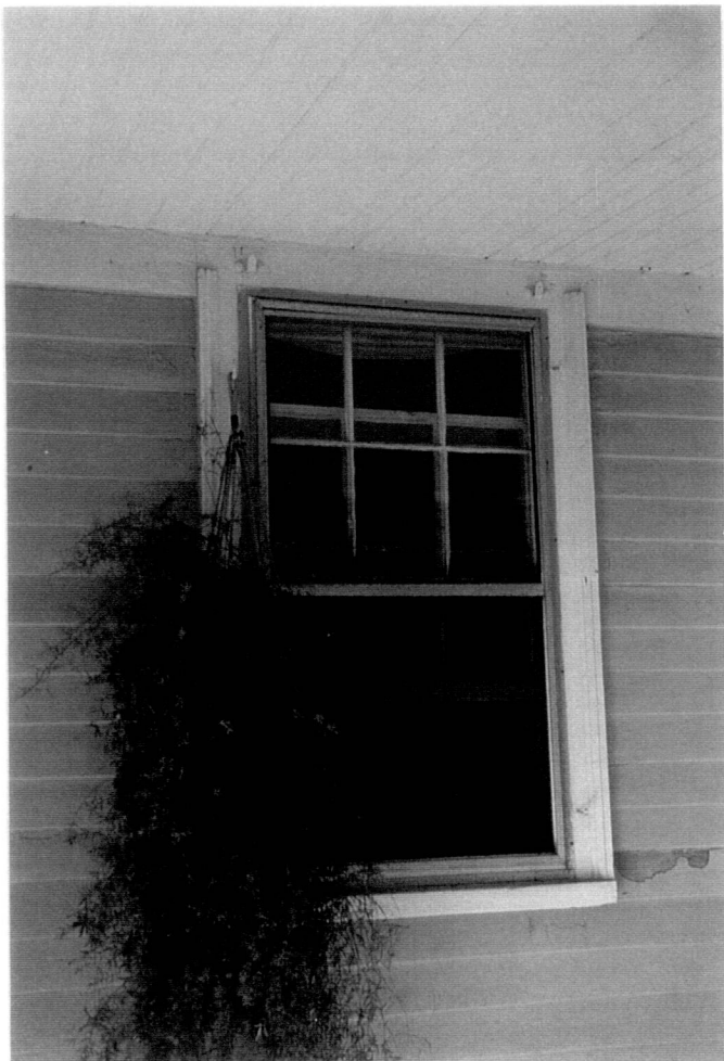
Figure 54. Gowing-Clark House – Main House East Wall, Window W105 (1999).
