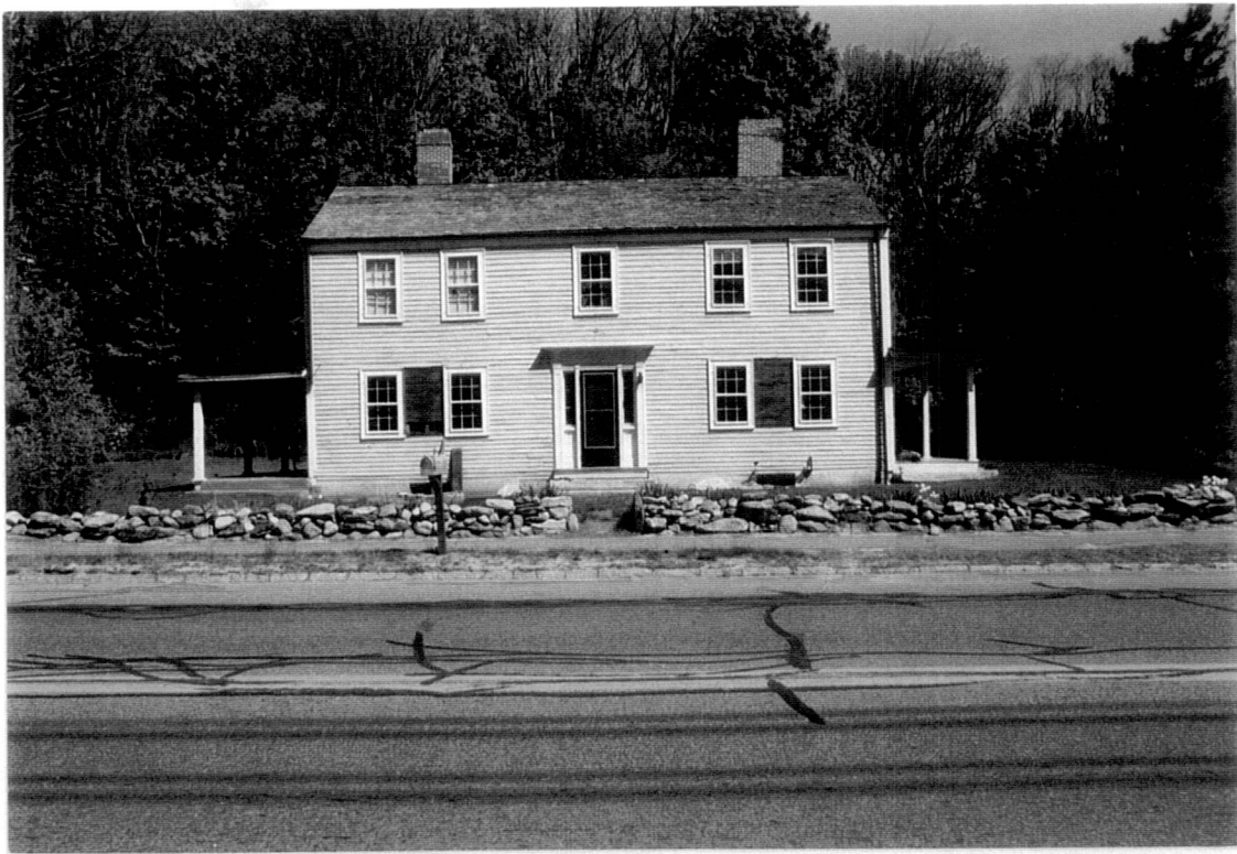
Figure 31. Gowling-Clark House – South Façade (1999).
