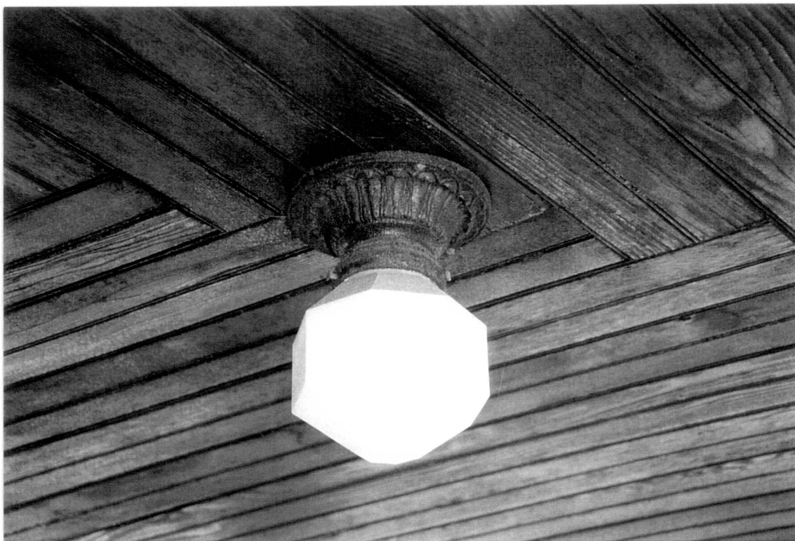
Figure 69. Gowing-Clark House – West Porch, Ceiling and Light Fixture Detail (1999).
