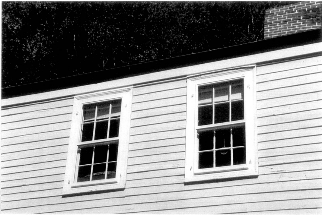
Figure 53. Gowing-Clark House – Main House South Façade, Windows W203 & W204 (1999).
