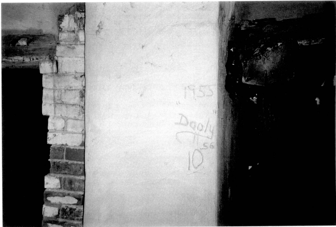
Figure 30. Gowing-Clark House – Ell Cellar, North Side of Center Chimney-Base Pier (2000).
