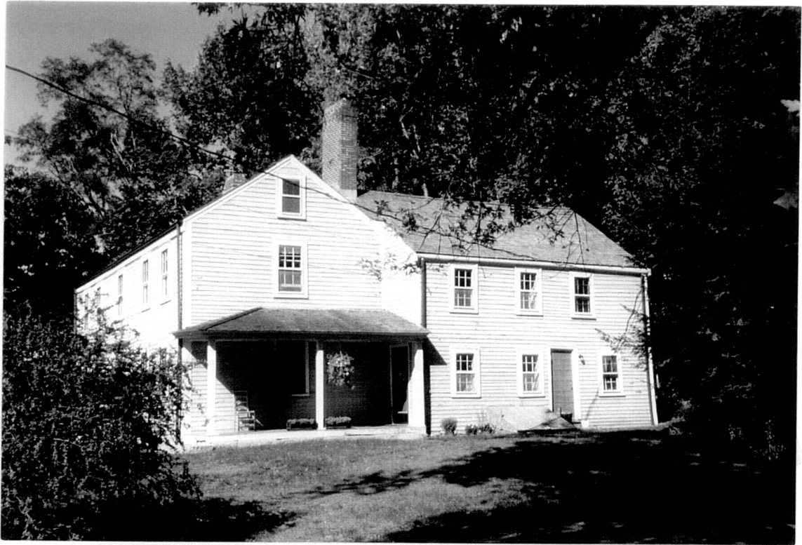
Figure 33. Gowling-Clark House – East Elevation (1999).
