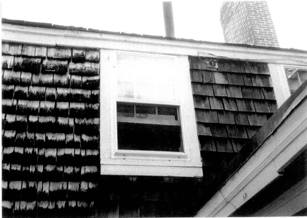
Figure 62. Gowing-Clark House – Ell West Wall, Window W211 (1999).
