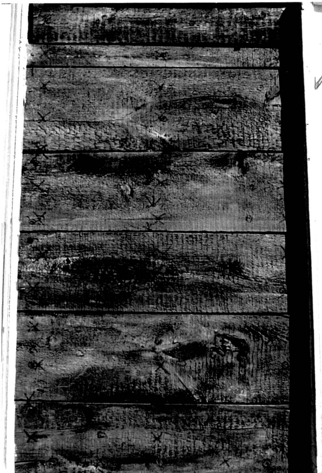
Figure 15. Gowing-Clark House – South Façade, East End, Detail Showing Original Mill-Sawn Sheathing (1999).
