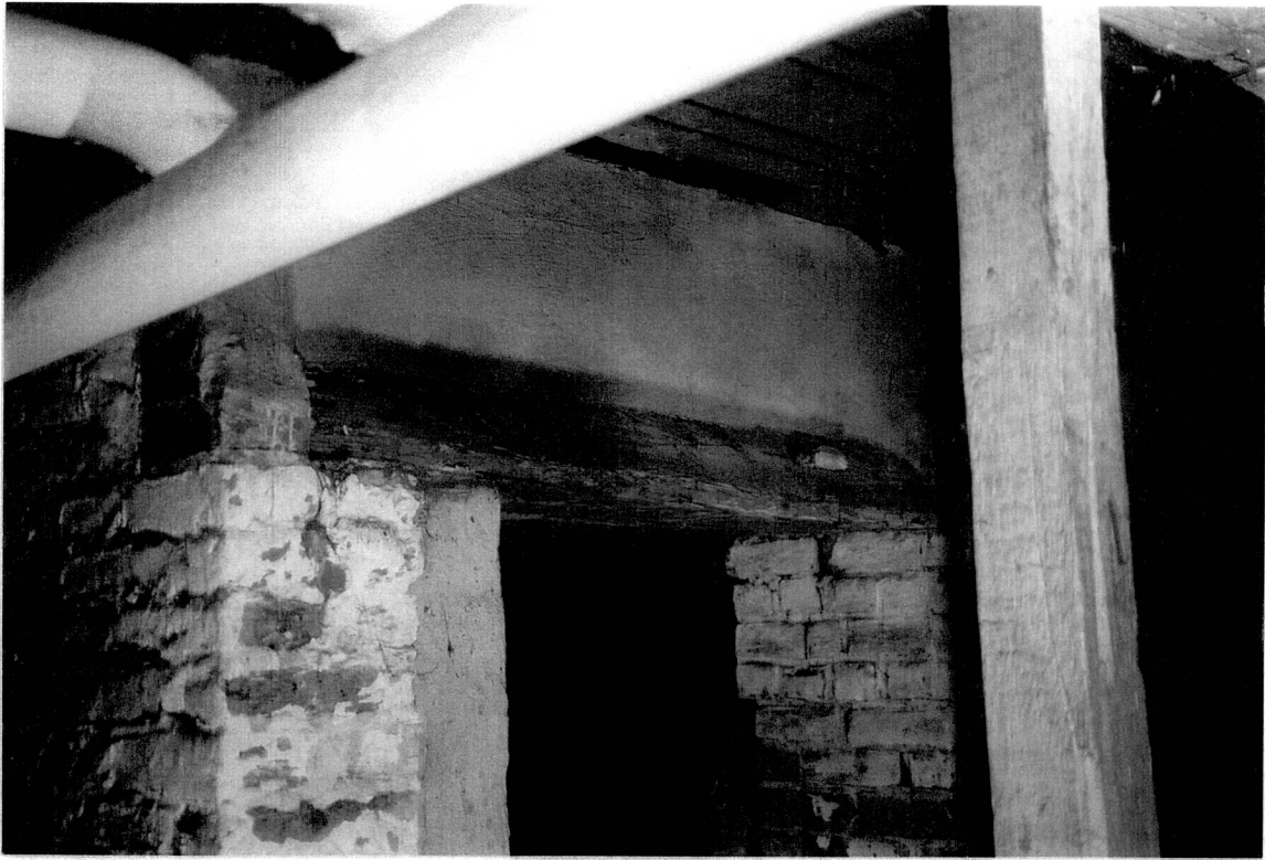
Figure 17. Gowing-Clark House – Ell Cellar, North Side of East Chimney Base (2000).
