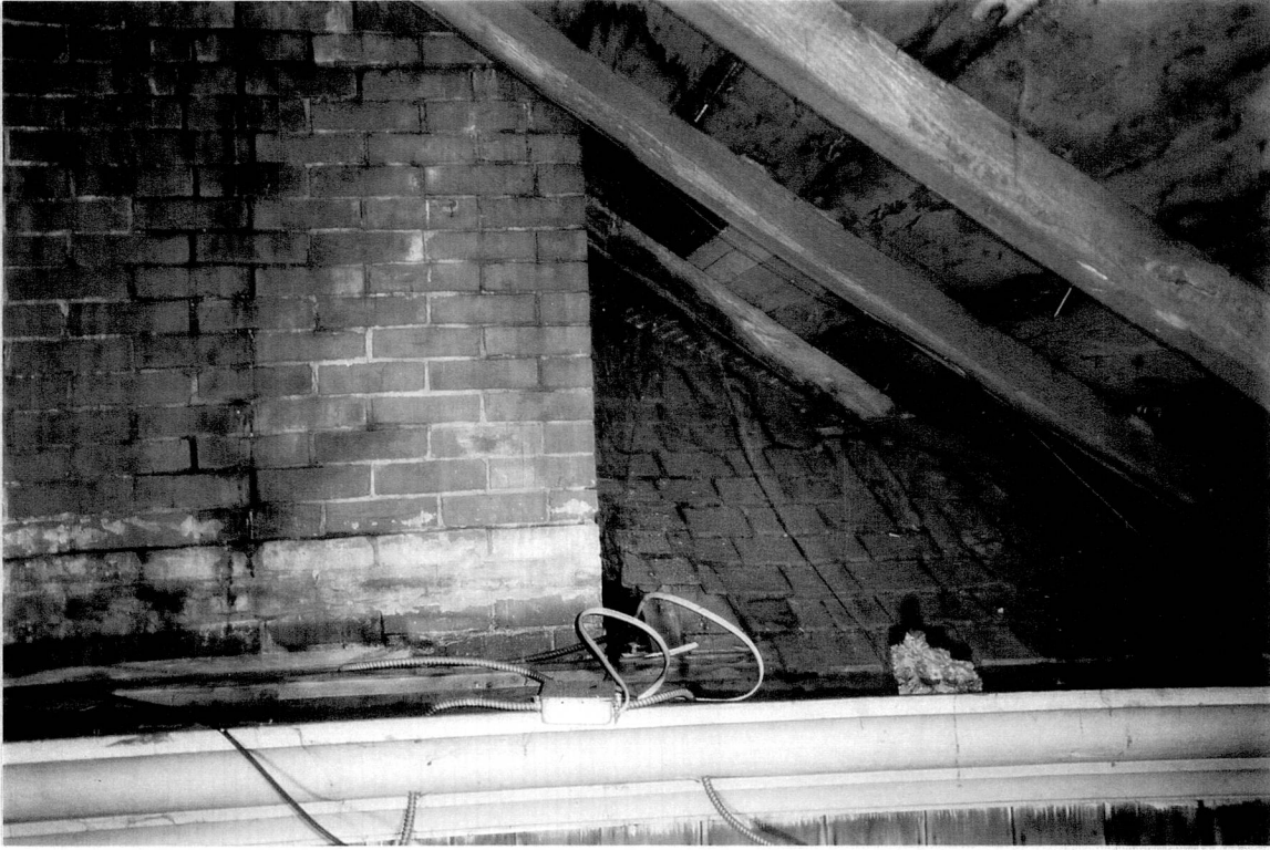
Figure 19. Gowling-Clark House – Ell Attic Looking South, Formerly-Exposed Original Roofing on North Slope of Main-House Roof (2000).
