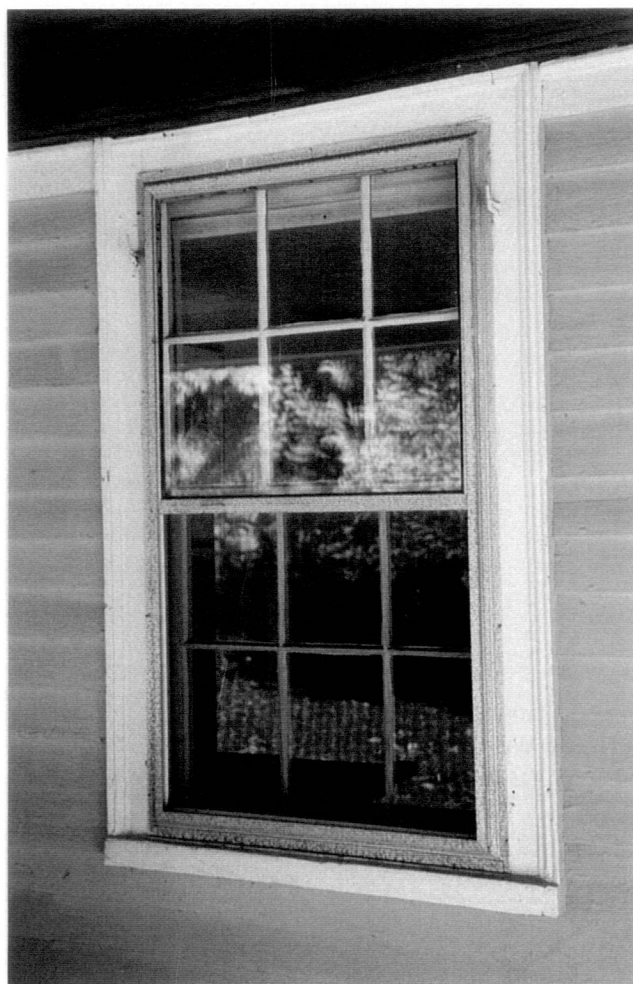
Figure 61. Gowing-Clark House – Main House West Wall, Window W113 (1999).
