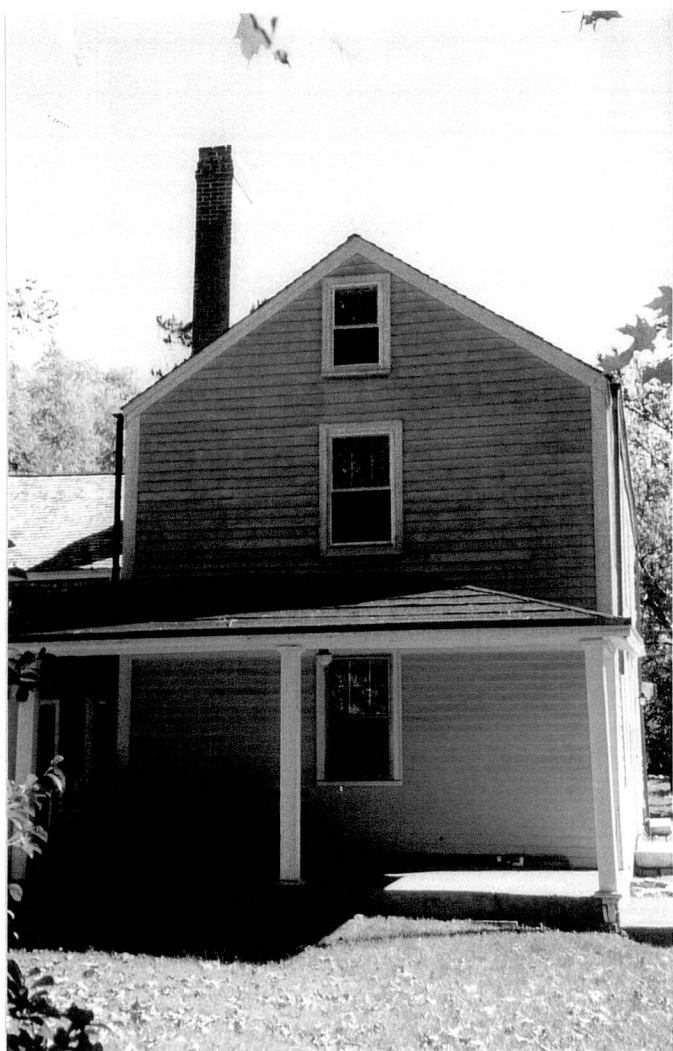
Figure 35. Gowing-Clark House – Main House West Wall (1999).
