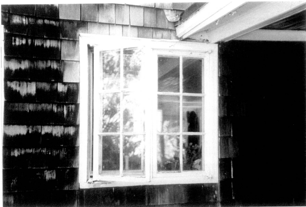
Figure 60. Gowing-Clark House – Ell West Wall, Window W111 (1999).
