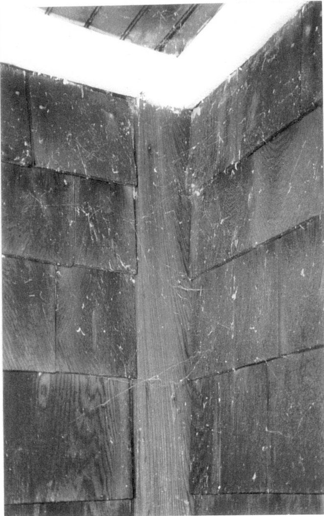
Figure 42. Gowing-Clark House – Junction of Ell West Wall with Main House North Wall (1999).
