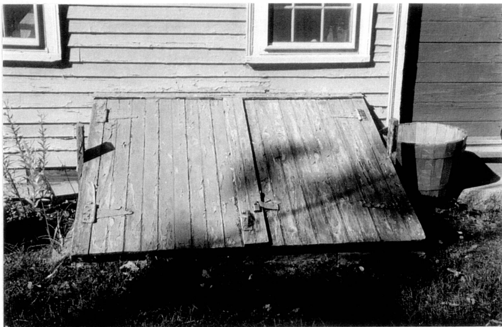
Figure 50. Gowing-Clark House – Ell East Wall, Bulkhead Doorway D001 (1999).
