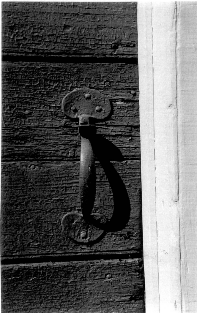
Figure 46. Gowing-Clark House – Ell East Wall, Doorway D103 Suffolk Latch (1999).
