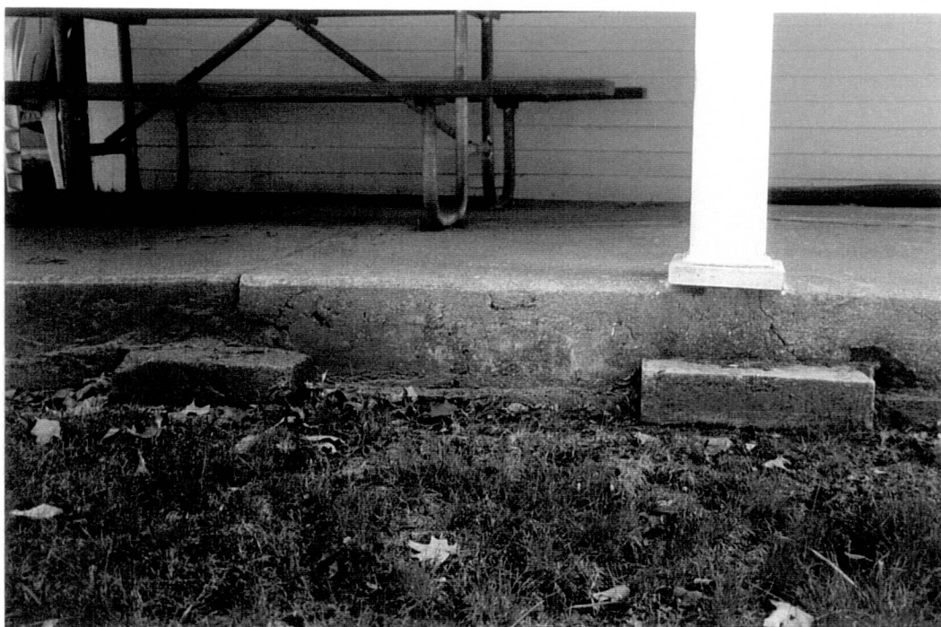
Figure 67. Gowing-Clark House – West Porch, Concrete Decking and Post Base Detail (1999).
