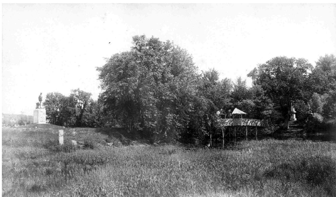
Figure 5. View northeast of The Minute Man (left), Minute Man enclosure fence. 1874 commemorative North Bridge and Battle Monument (right), c. 1880s. Concord River and wetland are in foreground. (MIMA Archives, Box 12, #34306)
