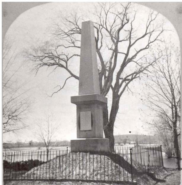
Figure 4. Stereoscopic view west of the Battle Monument. Note the Concord River in the background, the great elm behind the monument, and the iron fence enclosing the monument base. (Photograph Files, Concord Free Public Library)
