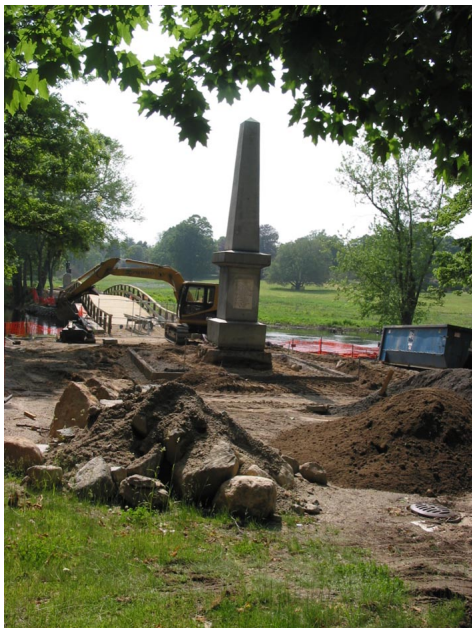
Figure 13. View west of the Battle Monument during re-grading of the avenue leading to the North Bridge and rehabilitation of the monument base, June 2005. (OCLP)
