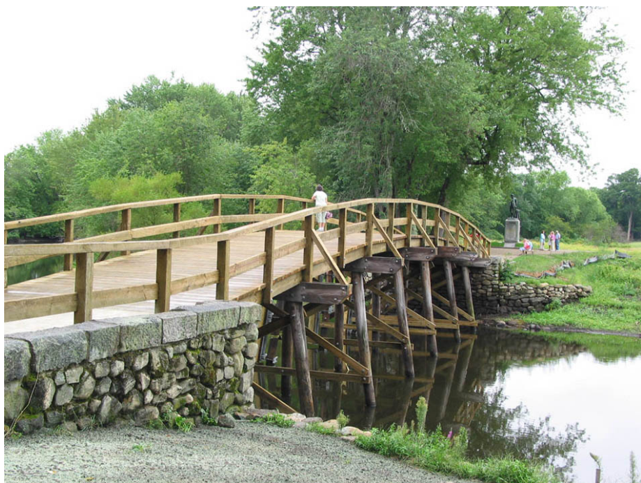
View southwest of the 1956 commemorative North Bridge, after restoration in 2005. (OCLP)
