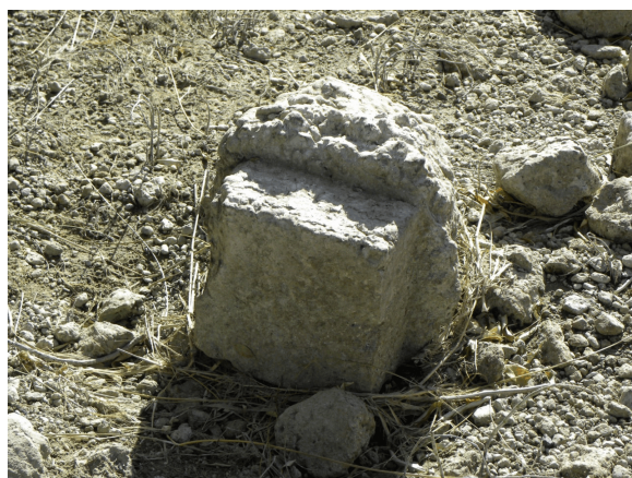
Figure 10. Small concrete footer, Robeson Property Feature 44.
