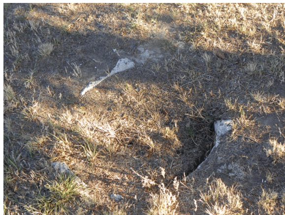
Figure 8. In situ relocation center manhole, Robeson Property Feature 1.14.
