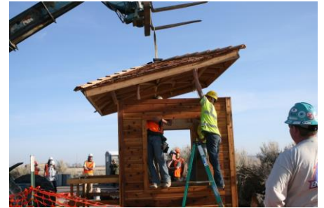
Boise State University students setting the roof onto the Guard Tower structure.
