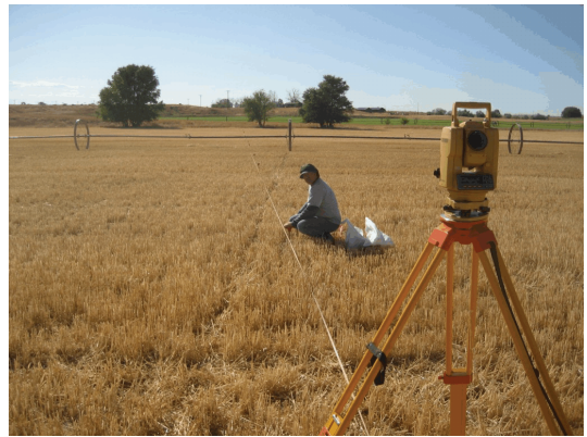
Figure 2. Laying out and staking barracks corners.
