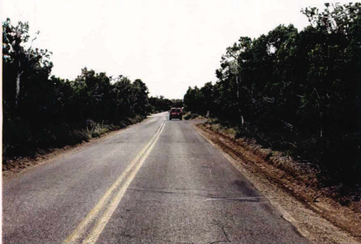
Photograph #34 - is looking north approaching the south intersection of the three-way.
