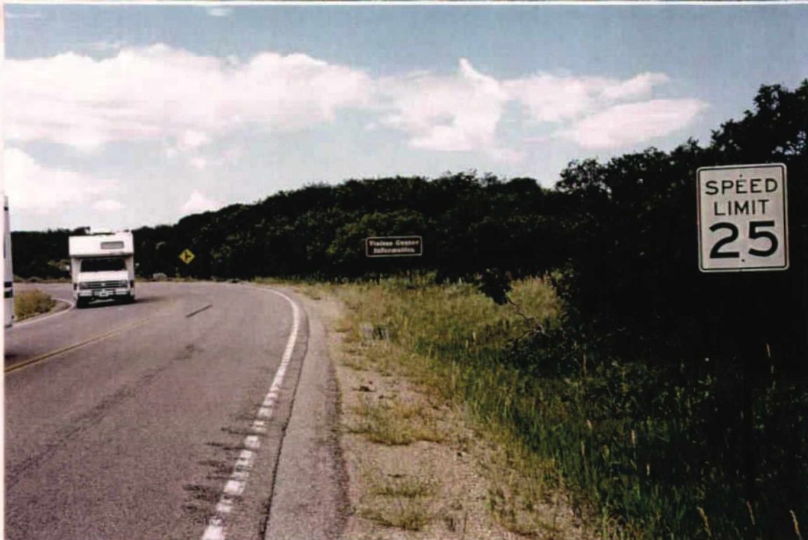
Photograph #1 - southbound at the entrance road at Mesa Verde approaching the Farview Visitor Center. The sign "Visitor Center Information" is on the right and perhaps should say next right or have a right arrow rather than just having the sign since the visitor center is on the left and the parking lot is on the right. There may be a better sign than the T-intersection warning sign that shows the variety of driveways or it may be that the sign is not necessary. If the sign is necessary, it should be replaced. It does not appear to be in very good shape and is probably not reflective.
