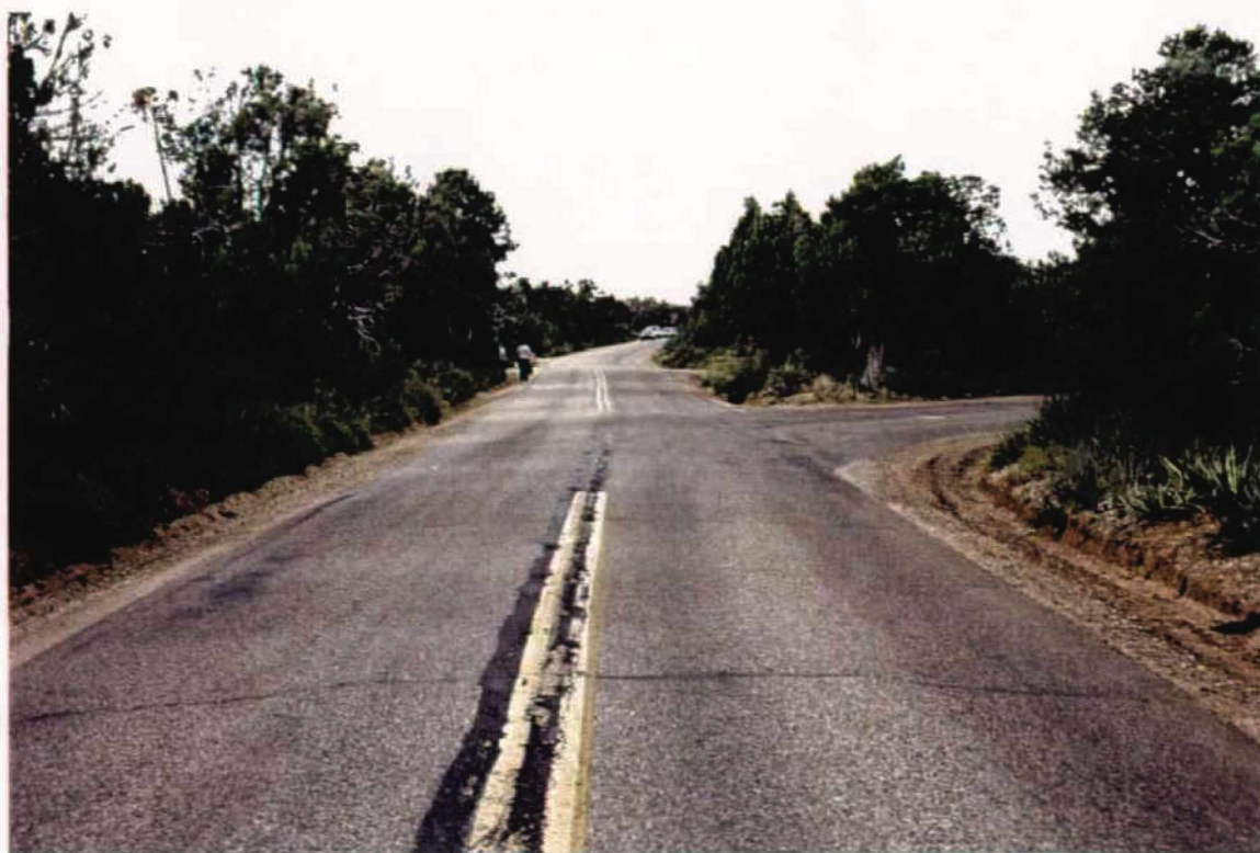
Photograph #35 - is looking north from just south of the south intersection.
