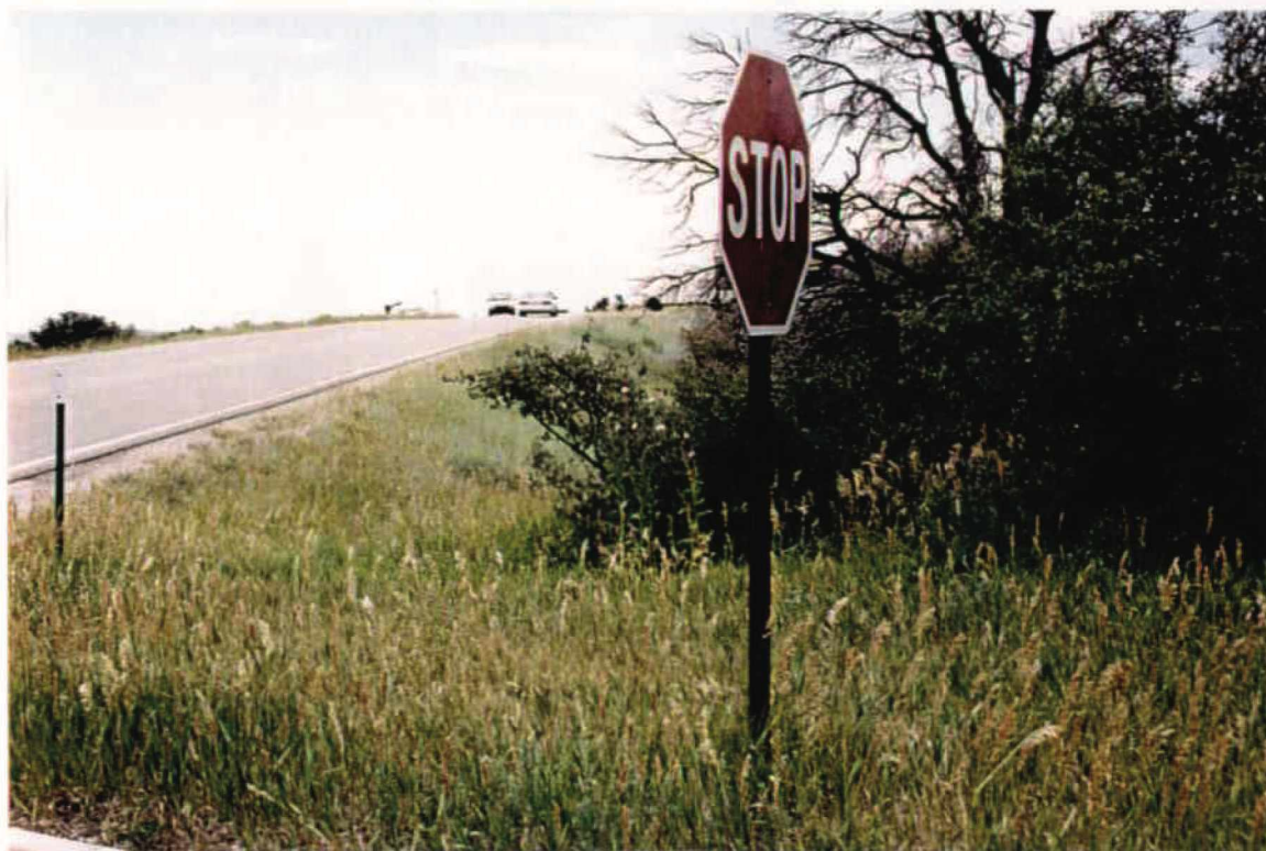
Photograph #11 - is looking in a southerly direction from the stop line. Shrubbery on the southwest corner of the driveway intersection should be trimmed to improve sight distance.
