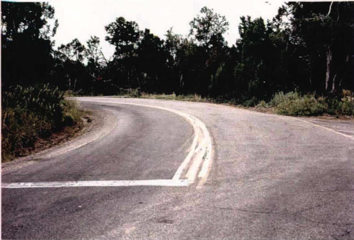
Photograph #24 - is looking southeasterly from the north intersection.
