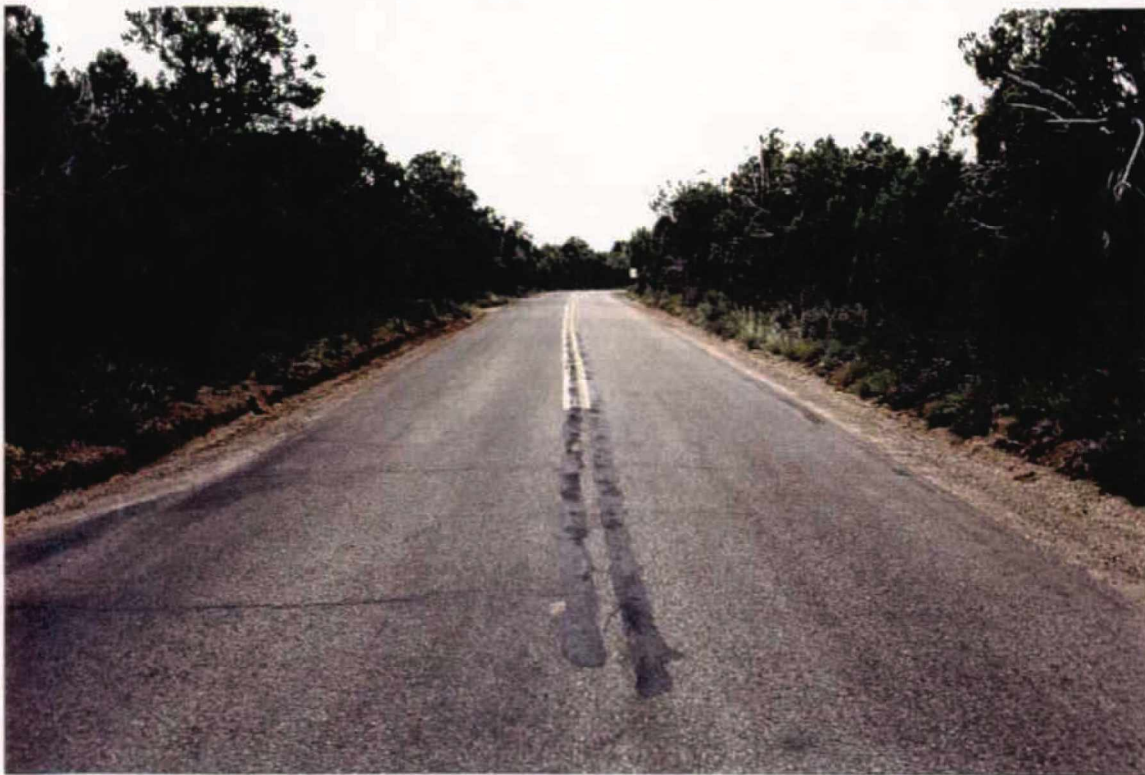
Photograph #25 - is looking south from the south intersection.
