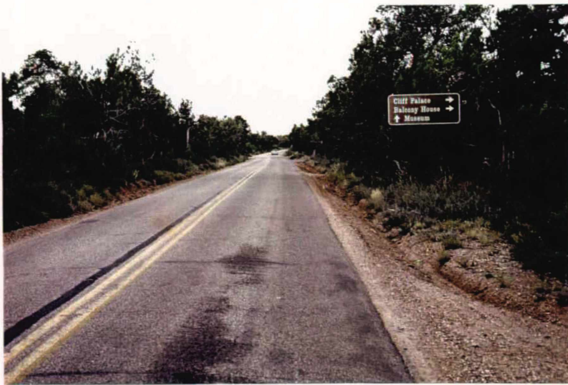
Photograph #33 - is looking north approaching the three-way.
