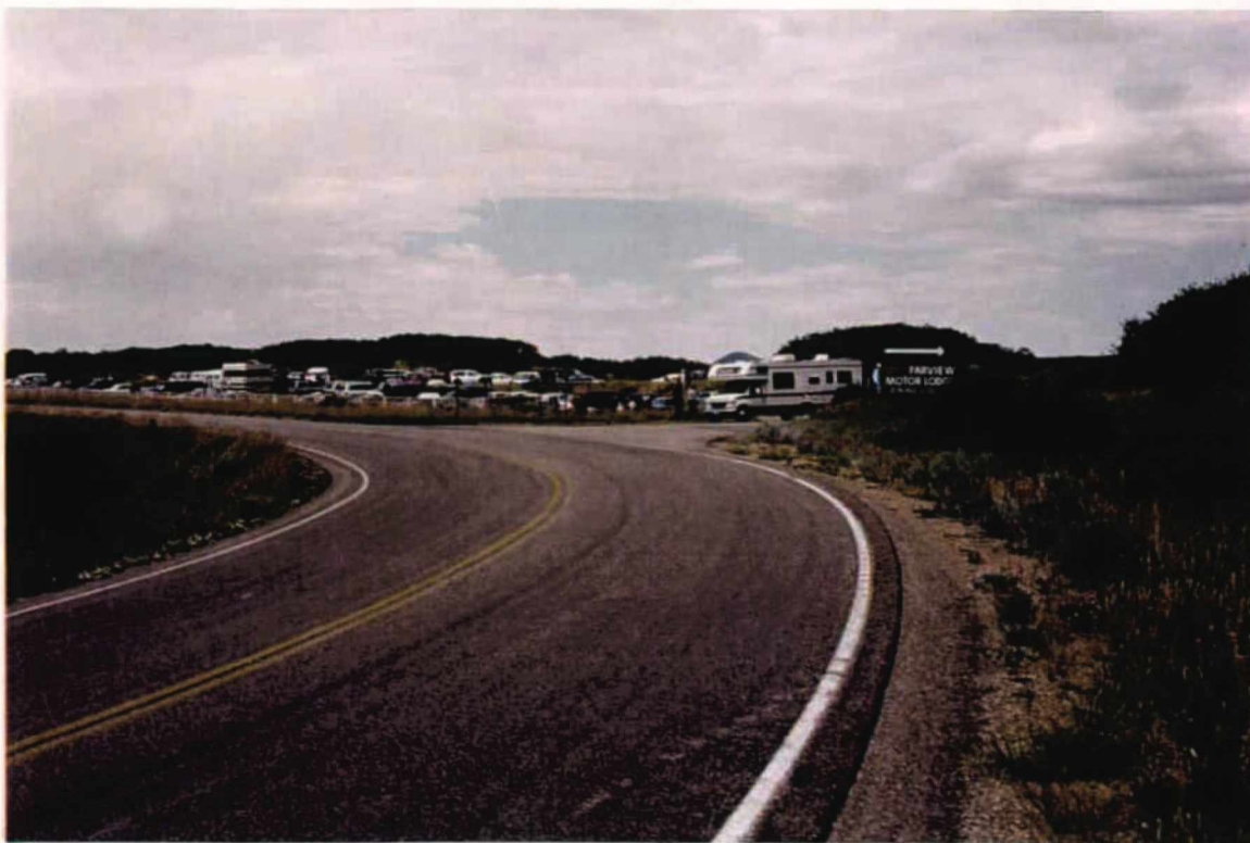
Photograph #2 - shows the driveway entrance and the road that is also the lodge entrance. Again, the visitor center parking perhaps would be more clear if there were an arrow to the right.
