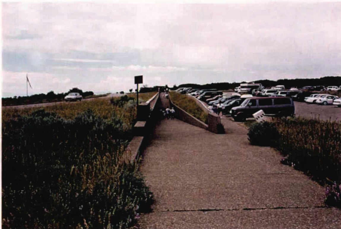
Photograph #5 - shows the ramp to the tunnel which goes under the road to the visitor center which seems to work quite well. Where the lodge road and the parking lot come together there seems to be some confusion because of the different directions people are going. A lot of movements are happening right in that area which is shown in Photograph #6 .
