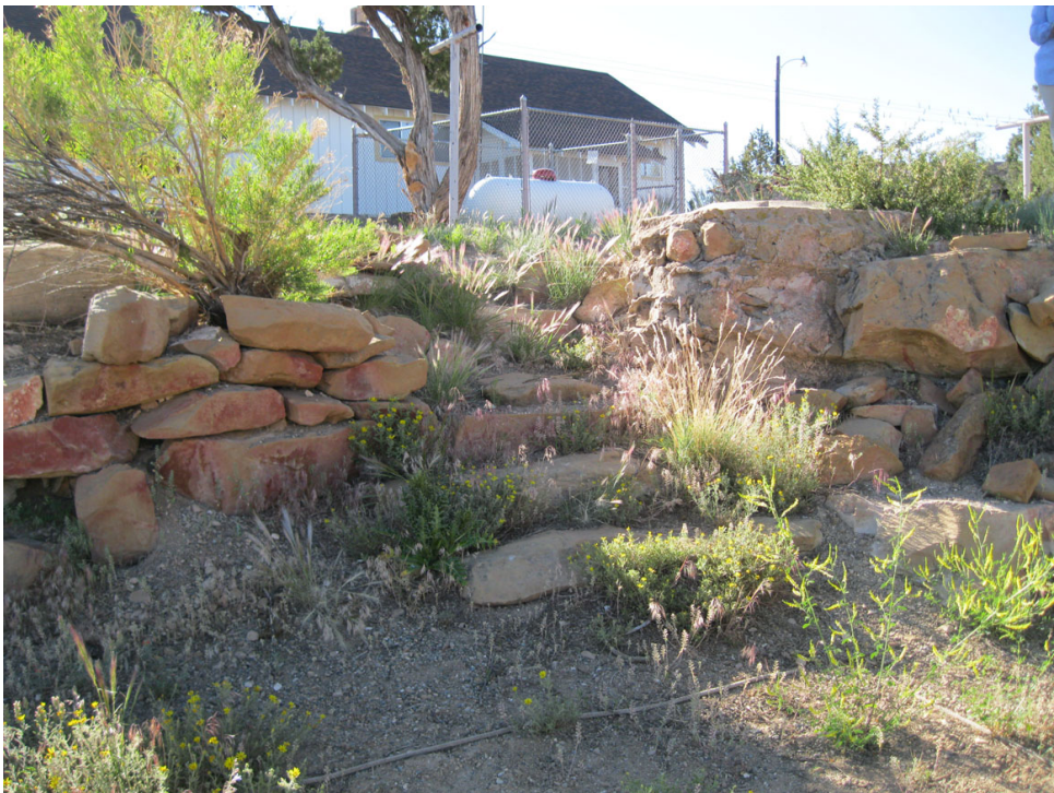
Stone steps, retaining walls, chainlink fences, and propane tanks are common small-scale features throughout the housing area, June 2010. Source: K. Miller, National Park Service.
