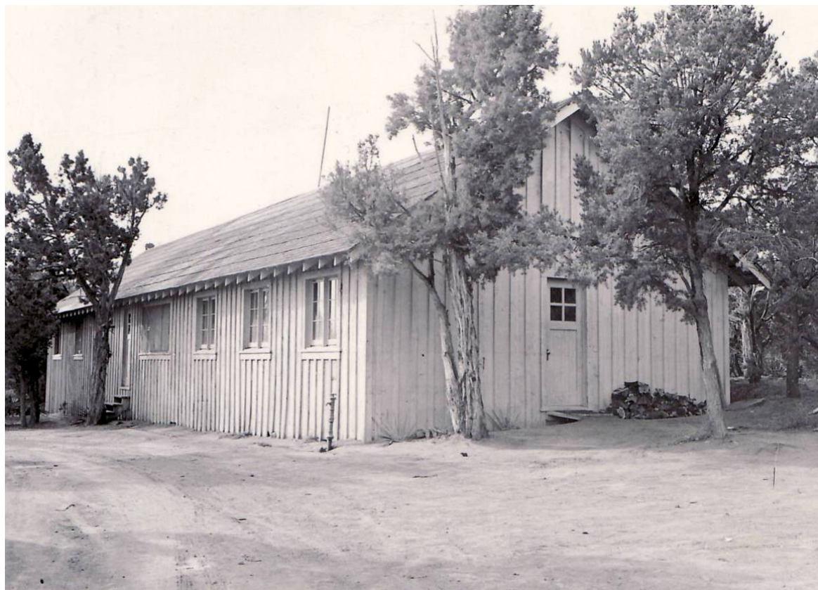
Bunkhouse/duplex (no. 16), October 1932. Source: Markley, Mesa Verde Archives, 9031.
