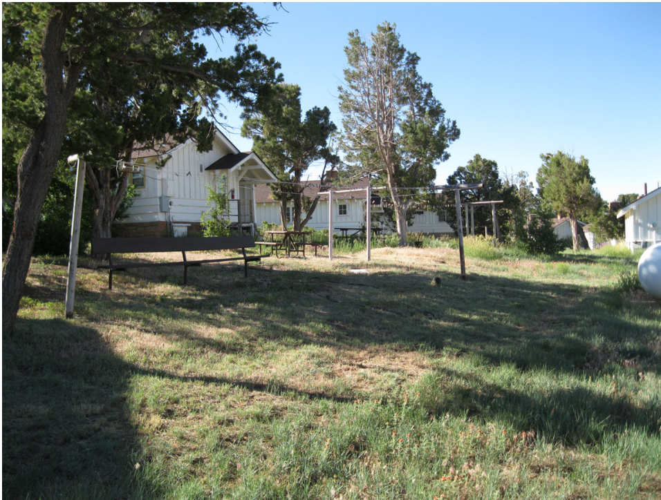
Residences along the drive within the Utility Housing Area, looking south, June 2010. Source: K. Miller, National Park Service.
