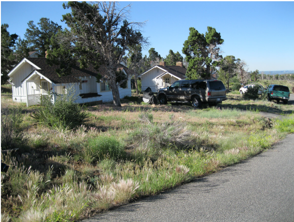
Cluster of Residences within the Utility Housing Area, June 2010. Source: K. Miller, National Park Service.
