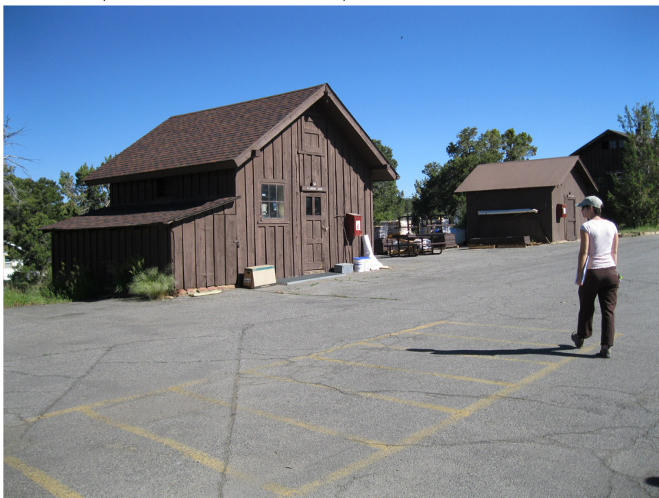
Plumbing Shop within the Maintenance Yard, constructed in 1929 in the NPS Rustic Style, June 2010. Source: K. Miller, National Park Service.
