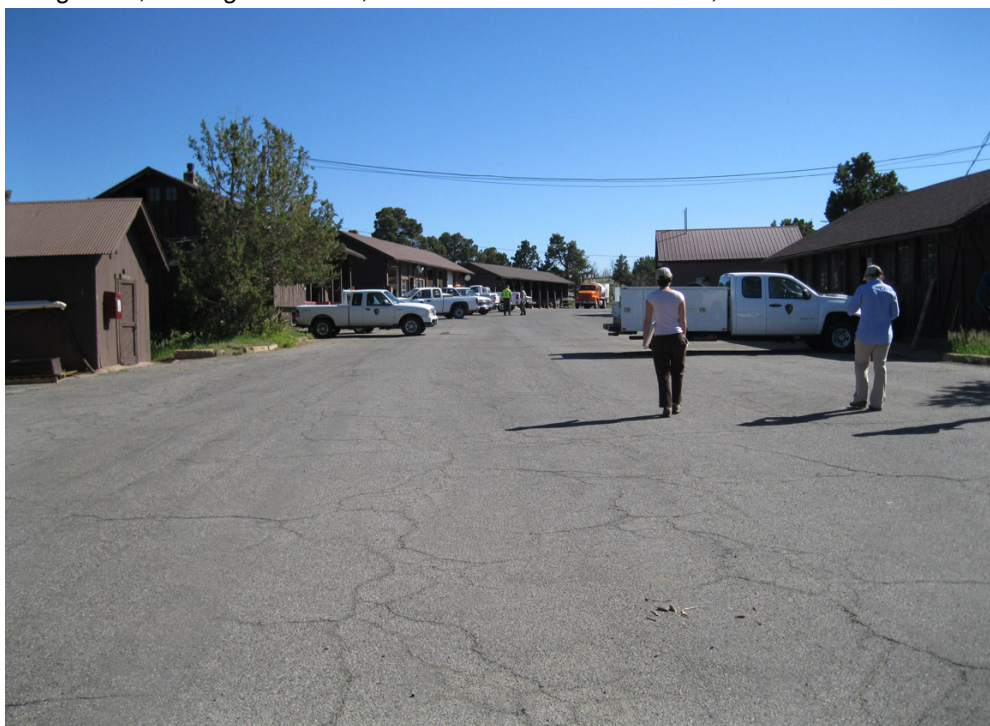
Cluster of buildings along the cross of the “T” formation within the Maintenance Yard, June 2010. Source: K. Miller, National Park Service.
