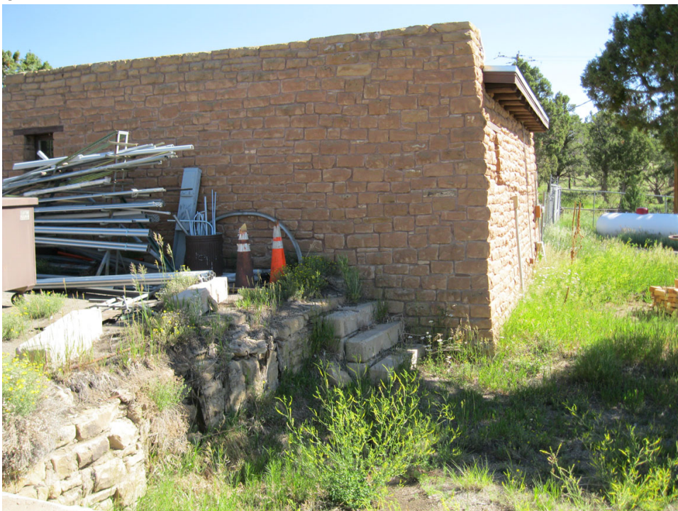
A 4-foot tall stone retaining wall and stockpile area at the southeast corner (rear) of the fire cache, June 2010. Source: K. Miller, National Park Service.
