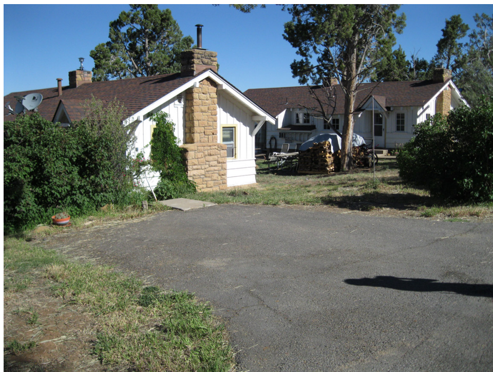
The Utility Area Housing remains to be used for its original purpose – seasonal and permanent employee housing, June 2010. Source: K. Miller, National Park Service.
