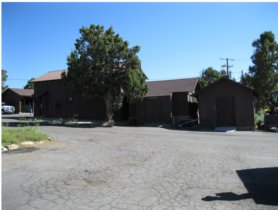
From L to R: The Snow Blast Shed, Blacksmith Shop, and Oil House, June 2010. Source: K. Miller, National Park Service.
