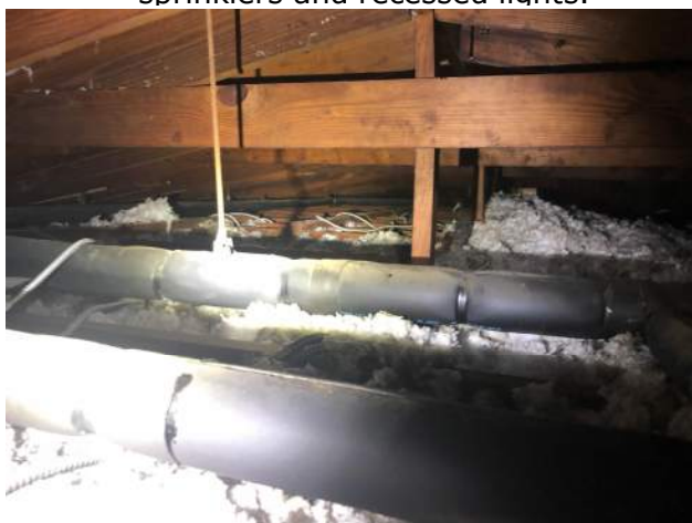
Photo 3 – View of attic.
