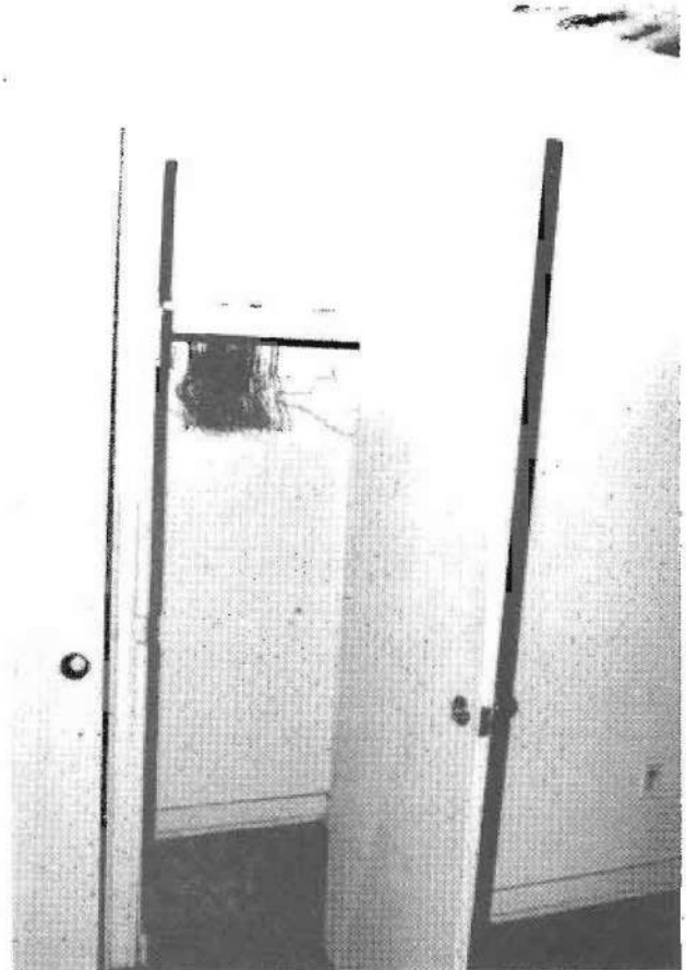
Figure 30. This photograph shows the back wall of the mechanical closet that extends into the closet opening in Bedroom 3. The mechanical closet encloses area that was once a part of the bedroom closet.
