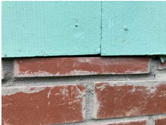
Figure 39. Transition from siding to brick.
