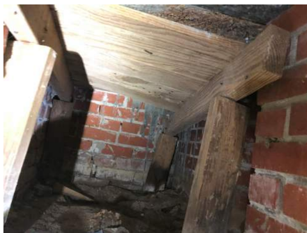
Photo 18 – Formwork left in place.
