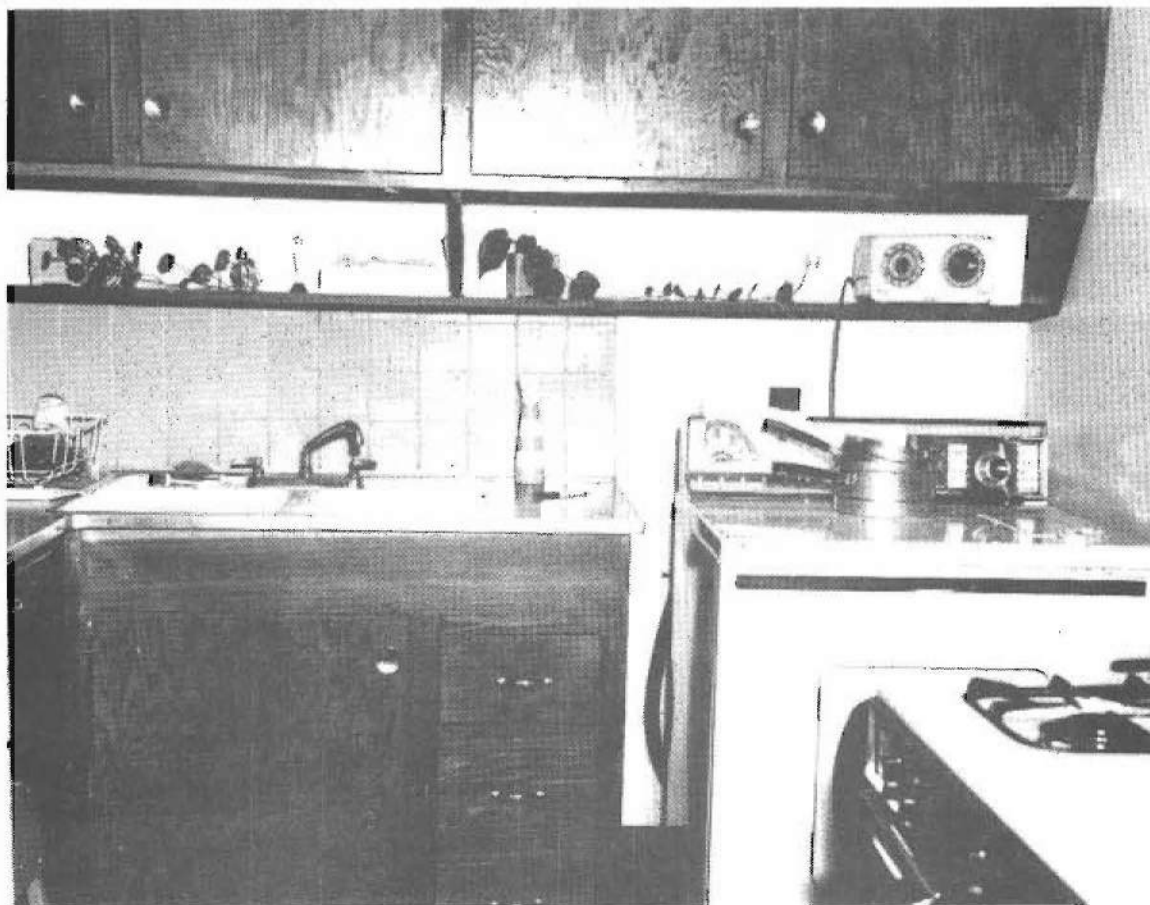
Figure 24. District Attorney's Office photograph taken the night of the assassination. The stained wood cabinets shown still exist in the same form, but they were painted some time after 1963. The countertop and sink also exist in the same form, but the sink faucet has been replaced. The washer shown is no longer in the house. Some of the drawer pulls shown remain, but none of the round door hardware remains.
