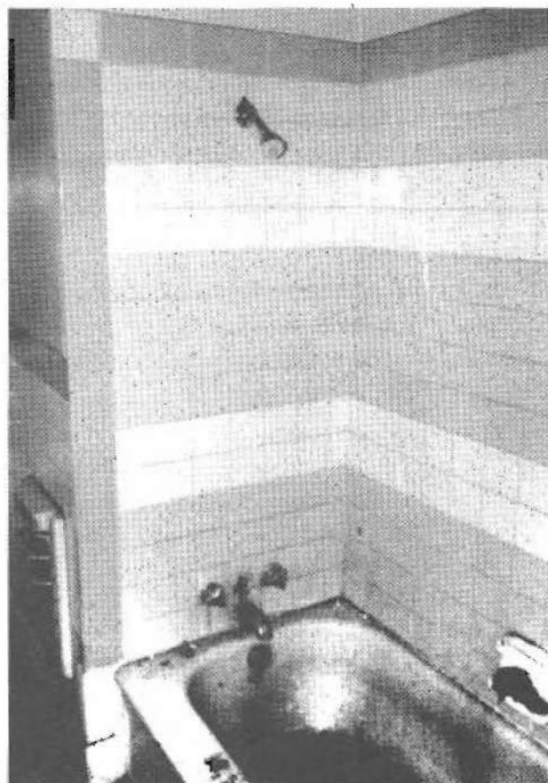
Figure 32. 1994 photograph of tub and tub surround.
