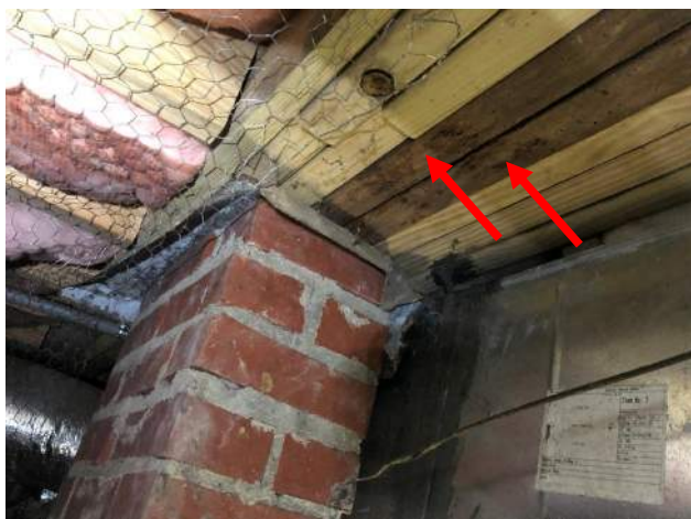
Photo 13 – Foundation pier and reinforced center beam.
