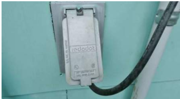
Figure 49. Weatherproof receptacle, when closed.
