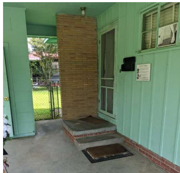
Figure 4. Main entry door within Carport.
