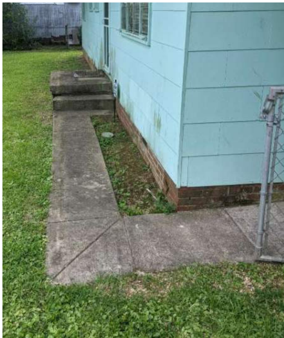
Figure 21. Existing rear sidewalk.
