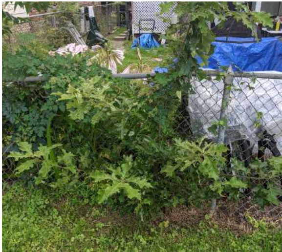
Figure 17. Overgrown existing fence.
