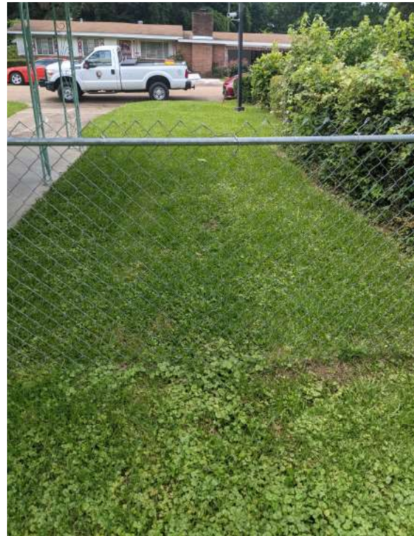
Figure 29. Sink hole where tree has been removed.
