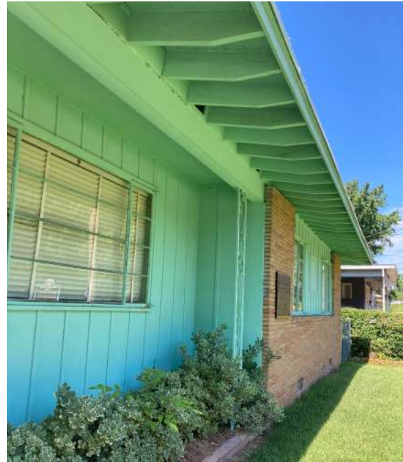
Figure 2. Front overhang and veneer materials.
