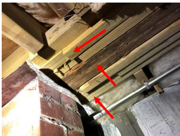
Photo 14 – Fit up of reinforced beam.
