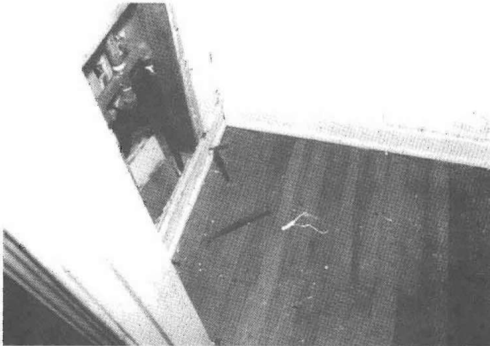
Figure 26. Photograph taken in 1994 of the bathtub plumbing access located in the closet of Bedroom 1.
