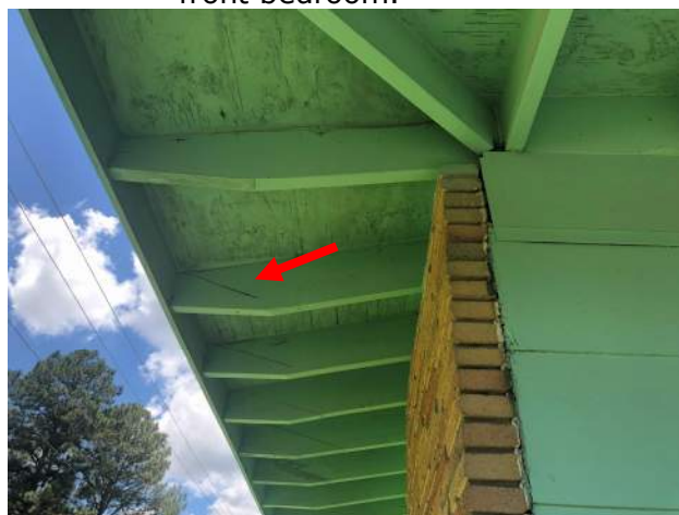
Photo 6 – Typical repair of rafter tails.
