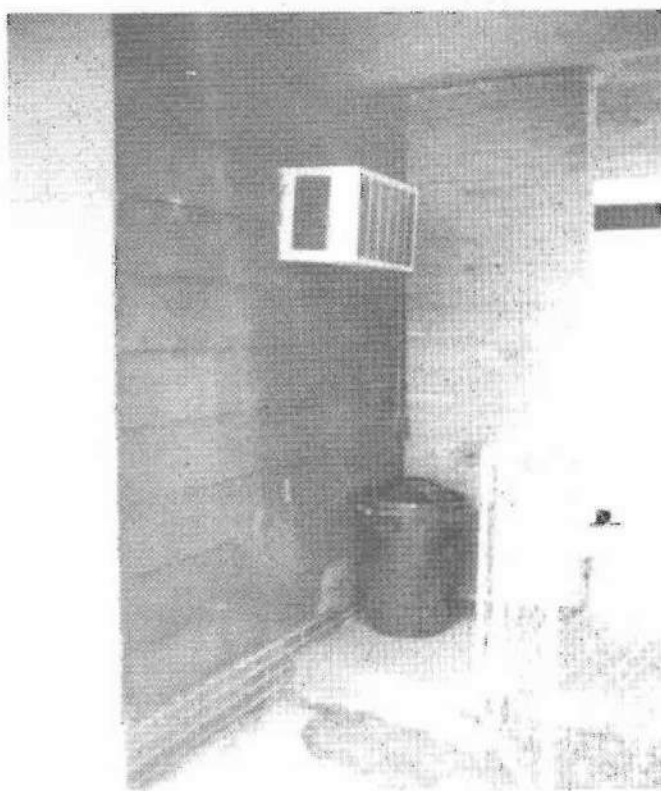
Figure 17. A view of the rear of the carport showing the brick wing wall behind the entry door and an air conditioner that appears in 1963 photographs.
