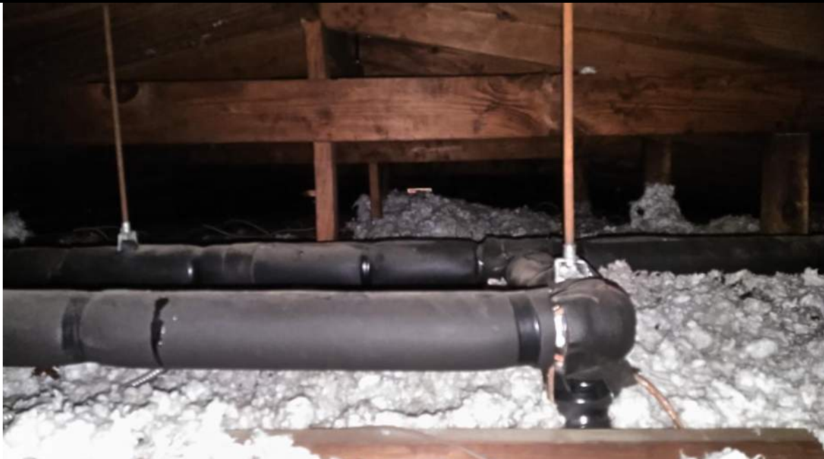
Photo 4: Attic Insulation (PSI HSM 04)
