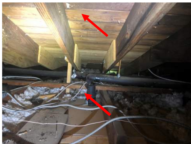
Photo 4 – Repair of rafters and roof sheathing.
