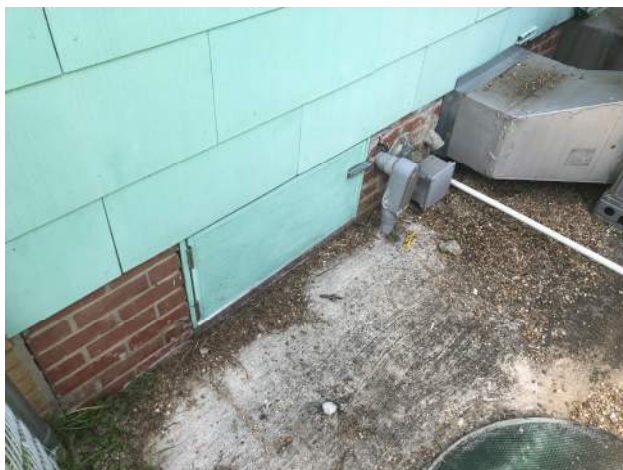
Photo 9 – Typical foundation wall, face brick and access to crawlspace on east side.
