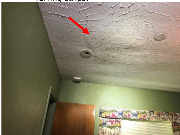
Photo 2 – Patches in ceiling for installation of sprinklers and recessed lights.
