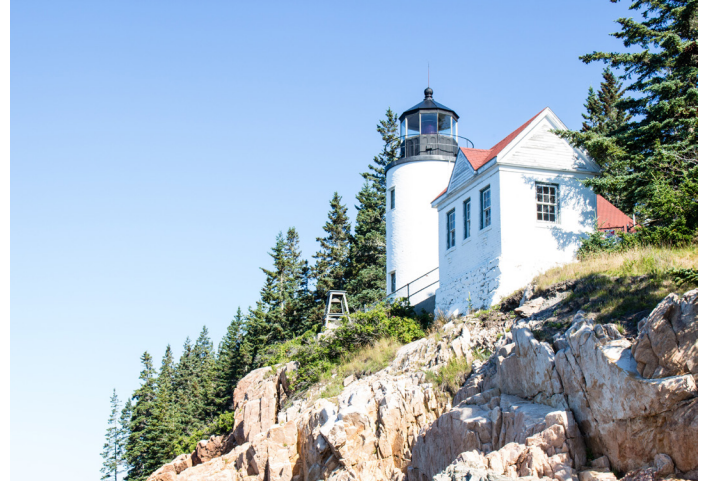
Bass Harbor Light Station, Bass Harbor, Maine
