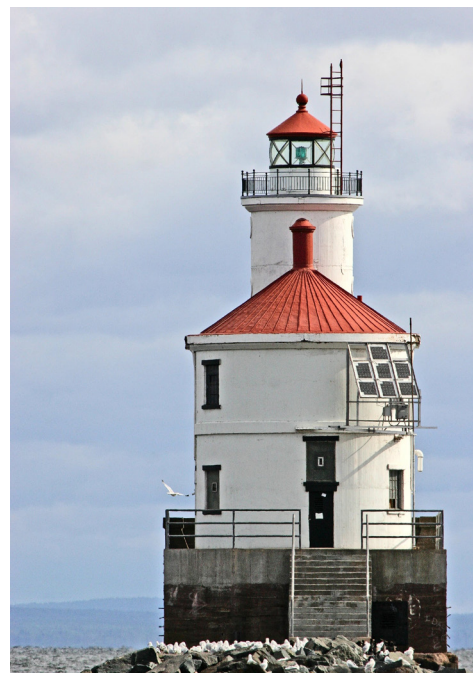
Superior Entry Lighthouse
