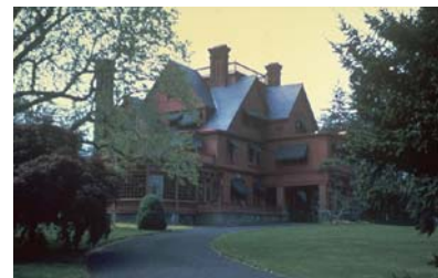
Edison National Historic Site
