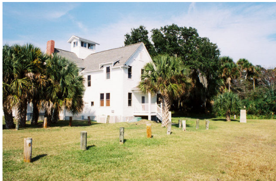
Eldora State House at Canaveral National Seashore
