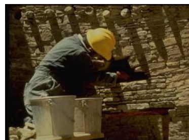
Mason repairs prehistoric stone walls, Chaco Culture NHP.
