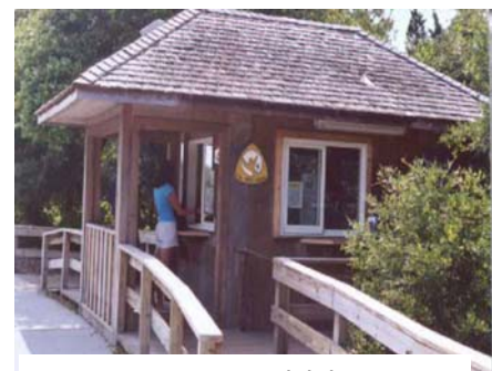
Cape Hatteras Lighthouse Entrance Station
