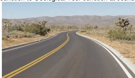
Keys View Junction to Geological Tour Junction at Joshua Tree NP
