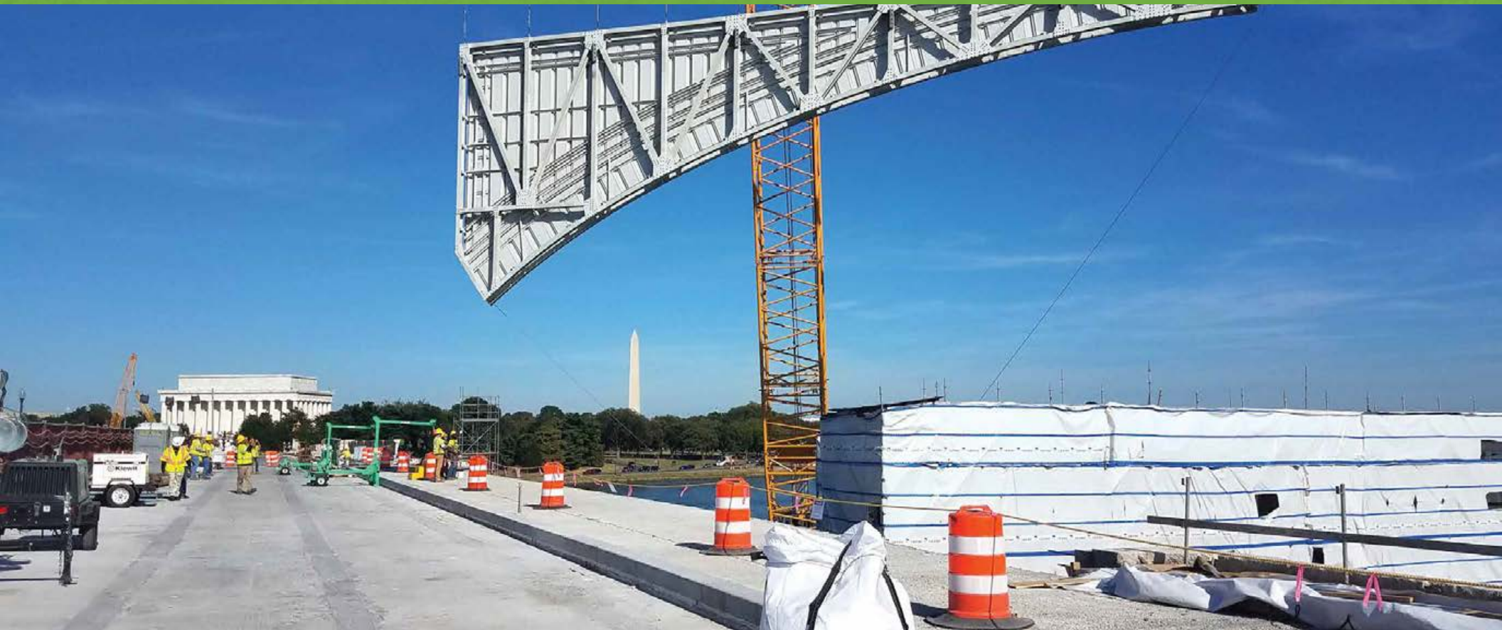
Crews lift and secure the restored metal bascule fascia back into place for the Arlington Memorial Bridge in Washington, DC.
