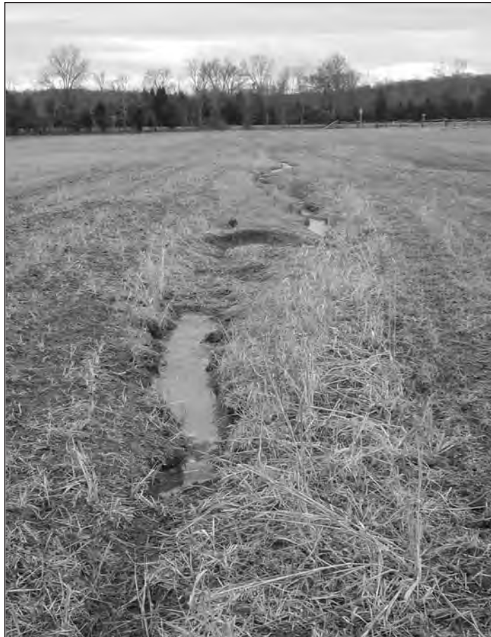
Figure 17. The drainage swale feeding into Young's Branch. The swale is located in the field occupying the southeast corner of the site. (2001; NCR CLP digital photo)
