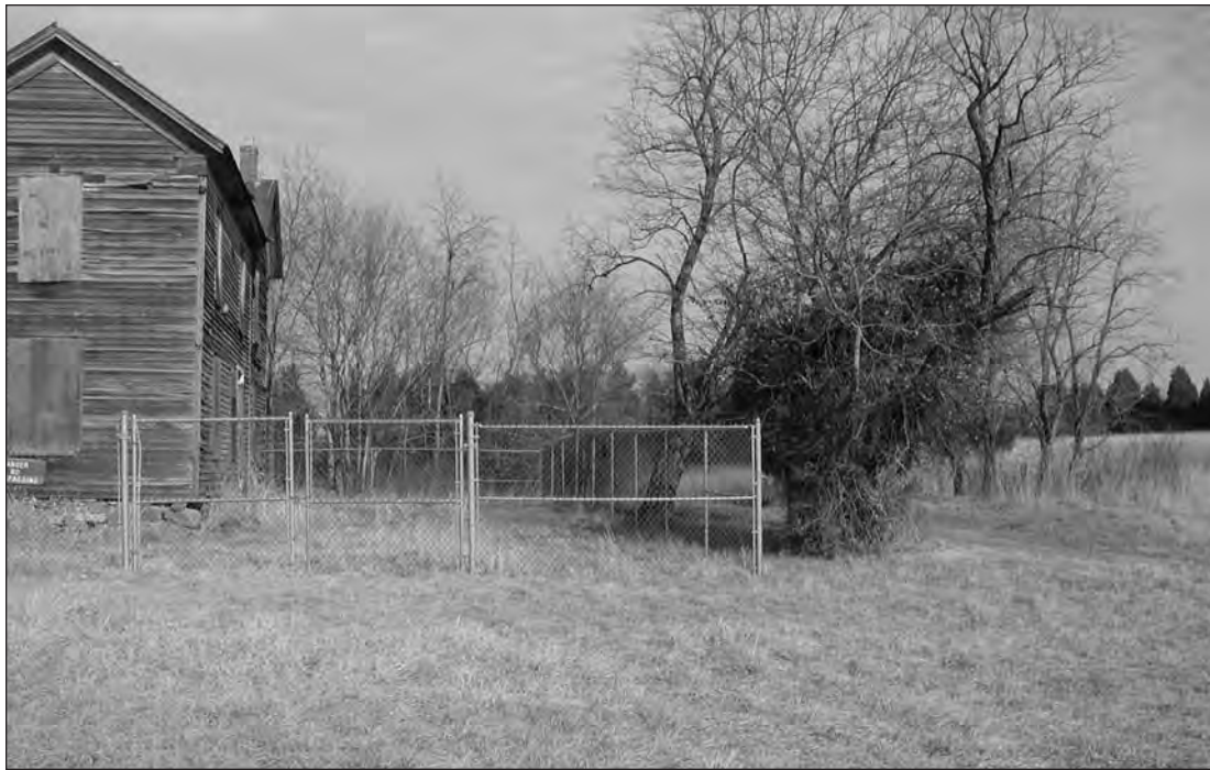
Figure 43. After the 1904/1905 enlargement of the house, the façade faced east towards the farm road. The trace of this road is visible on the right. (2002; NCR CLP digital photo)
