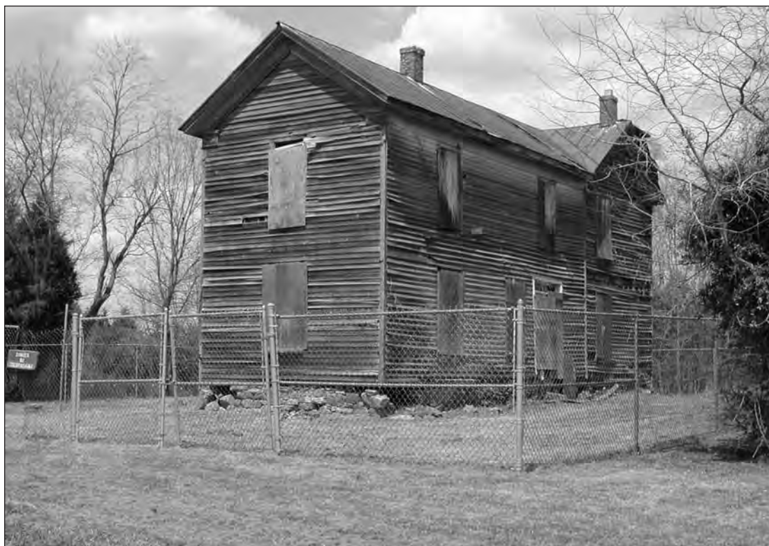
Figure 40. The existing farmhouse, oblique view of the south and east elevations. (2001; NCR CLP digital photo)
