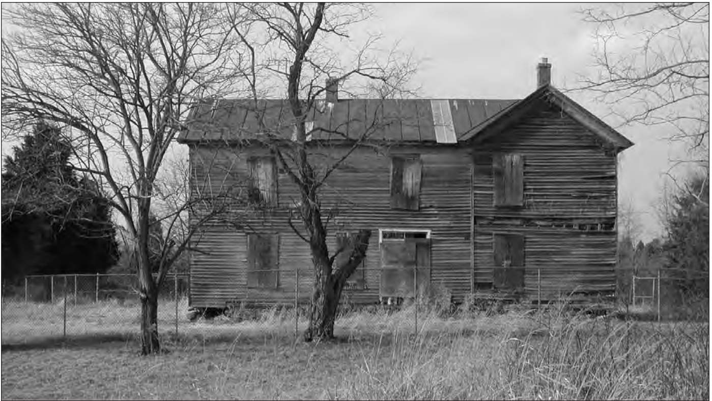
Figure 42. The house's north block, to the right, seen from across the historic road trace, incorporates a late-eighteenth or early-nineteenth-century structure that was probably moved to this site at some time between 1862 and 1904. (2002; NCR CLP digital photo)
