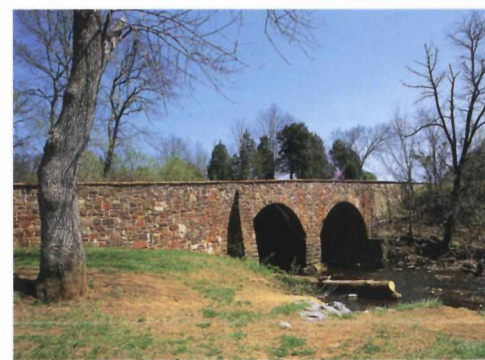
Stone Bridge, tour stop 11
