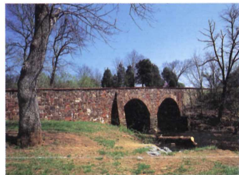
Stone Bridge, tour stop 11
