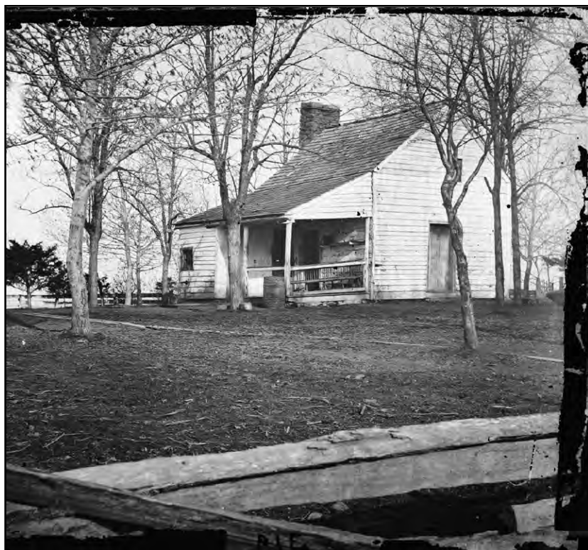
FIGURE 48: The James Robinson House in 1862 (Barnard 1862a)
