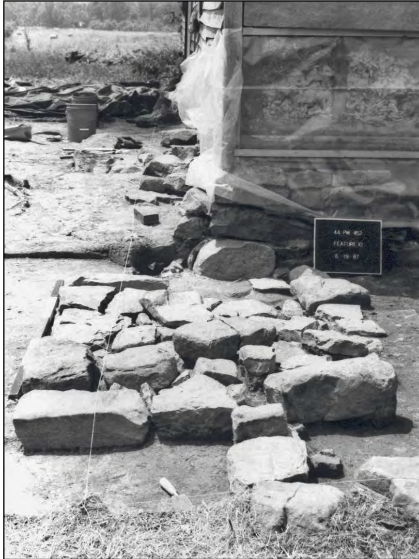
FIGURE 7: Chimney Base of Old House in 1987 (Parker 1989)
