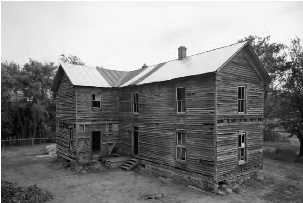
FIGURE 5: The Brawner Farmhouse Before Rehabilitation, 2006 to 2007, Facing Northeast (HABS 1933a)
