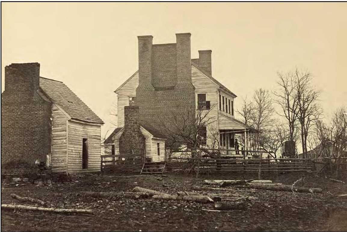
FIGURE 36: Portici in 1862, Facing North (NPS)
