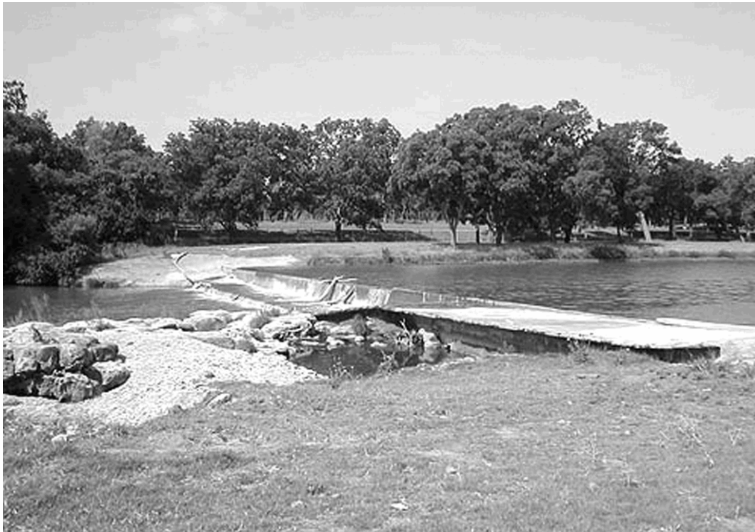
Johnson Dam & Low-Water Crossing (HB-050): One of the first improvements made to the ranch after its purchase. Water from the Pedernales was diverted for irrigation and the pond created by the dam provided a swimming hole."Photo by LYJO.
