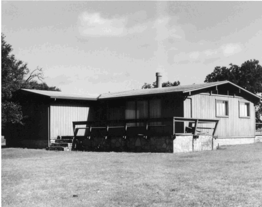
Cedar Guest House (HB-83): LBJ erected this house during his presidency as housing for high administrative officials. Photo by E. Degutis, 1993.
