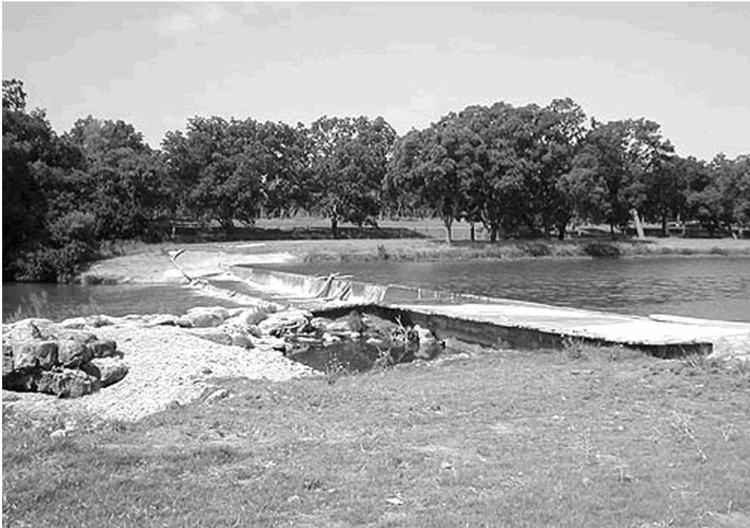
Johnson Dam and River Crossing. Photo by LYJO.
