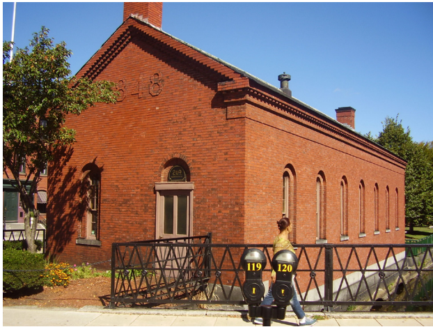
Moody Street Feeder Gatehouse-Information Center on Merrimack Street.
