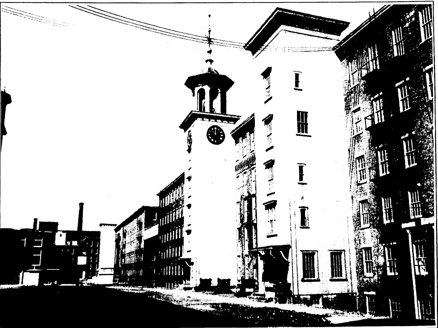
Figure 21. View of Boot Cotton Mills looking west, by John Coolidge. Circa 1930s. Source: Museum of American Textile History. Note the sidewalk along Mills No. 1 and 2 and traces of the paths across the Mill Yard.
