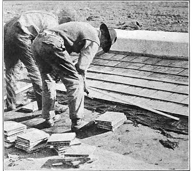
Laying Cement Tile
