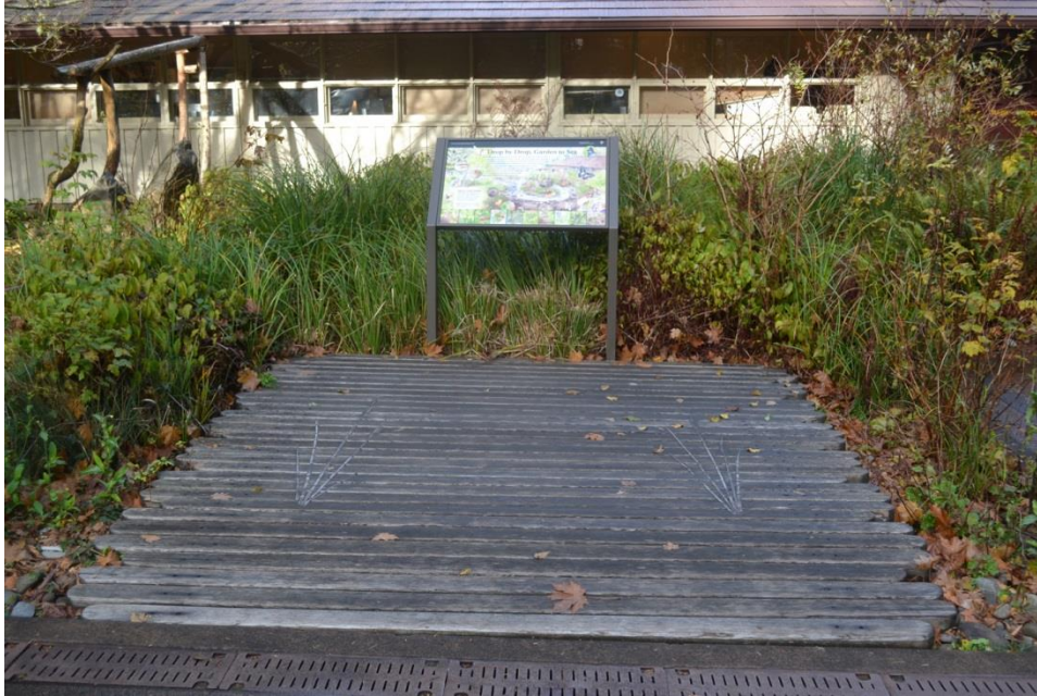
View of the rain garden and wayside exhibit in front of the visitor center. (WJE/LSHLA)
