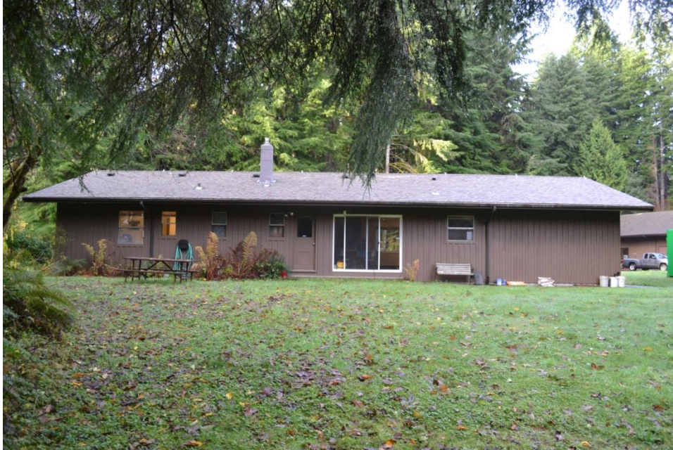
View west of the rear facade of the resources building. (WJE/LSHLA)
