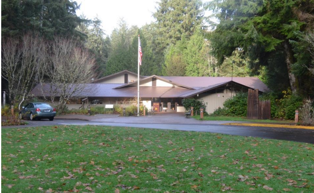
View north toward the visitor center, principal facade. (WJE/LSHLA)
