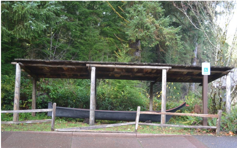
View of the canoe shelter in front of the visitor center. (WJE/LSHLA)
