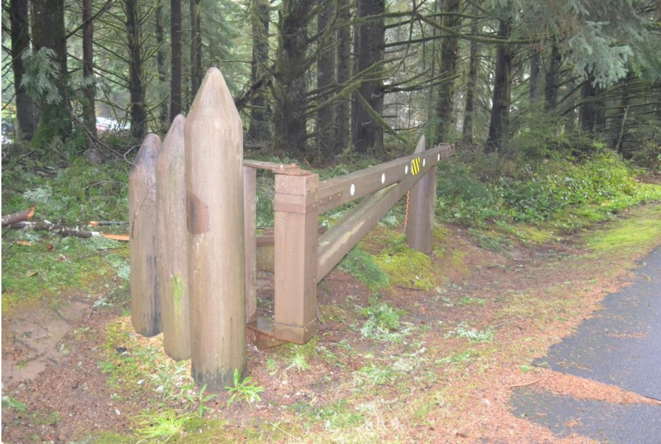
View of the gate at the visitor center access road. (WJE/LSHLA)
