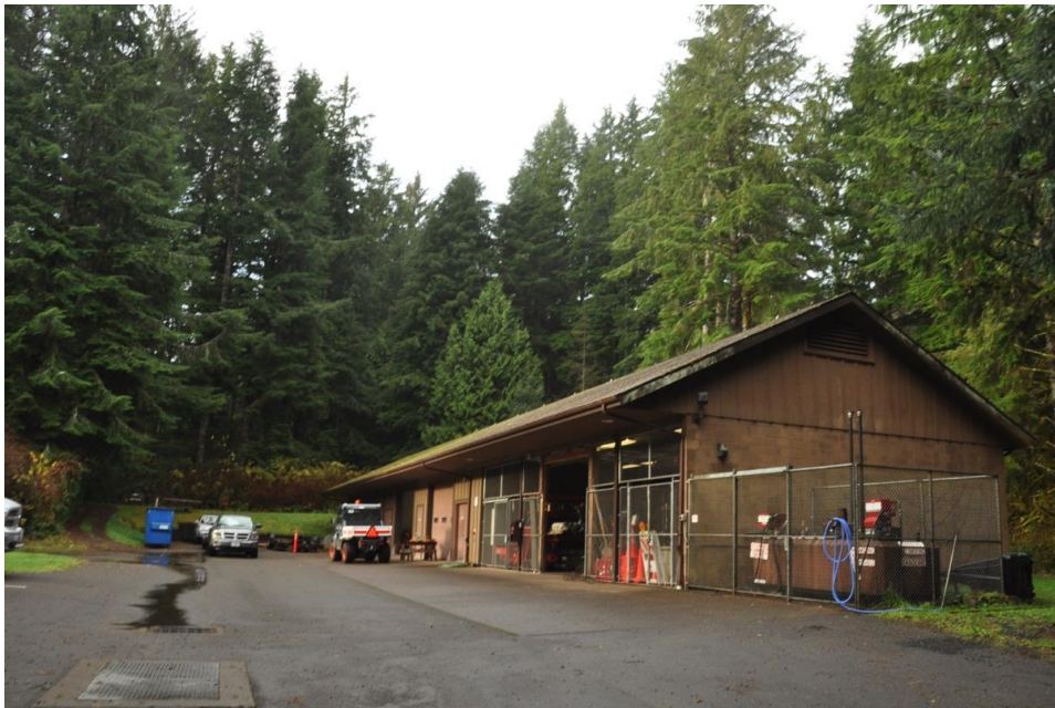
View southwest toward the maintenance shop access road and associated parking. (WJE/LSHLA)
