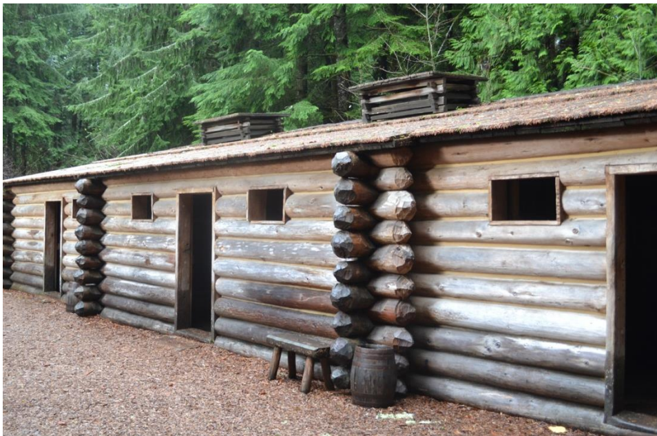
View northeast of a bench and barrel used to interpret historic furnishings associated with the fort during the winter encampment of the Corps of Discovery in 1805–1806. (LSHLA)
