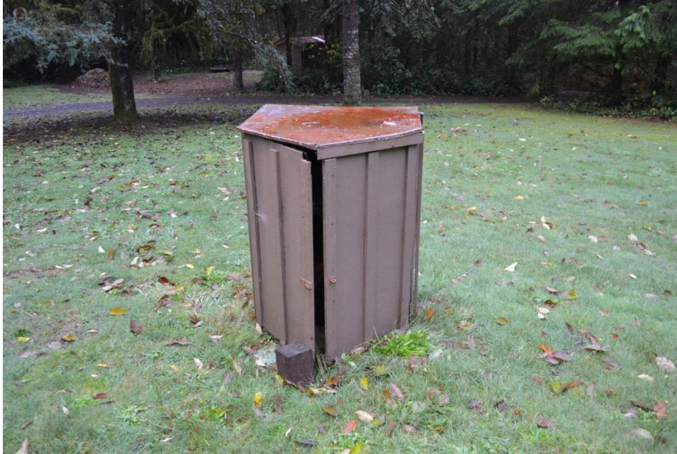
View of the stand pipe cover structure. (WJE/LSHLA)
