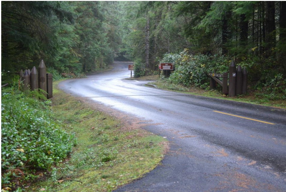
View looking southwest along the park entrance road. (WJE/LSHLA)
