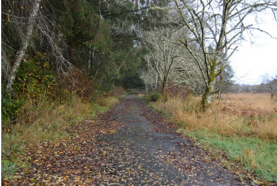
View north along the surviving section of the vacated county road. (WJE/LSHLA)
