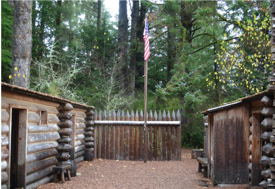
View northeast of the flagpole within the Fort Clatsop replica. (LSHLA)
