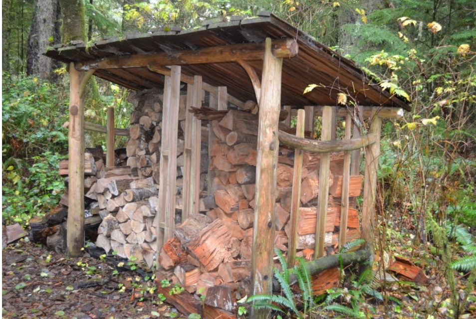
View of the firewood box. (WJE/LSHLA)
