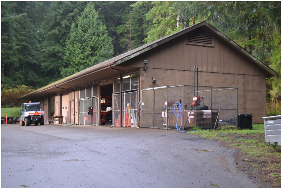
View southwest of the principal and side facades of the maintenance shop. (WJE/LSHLA)
