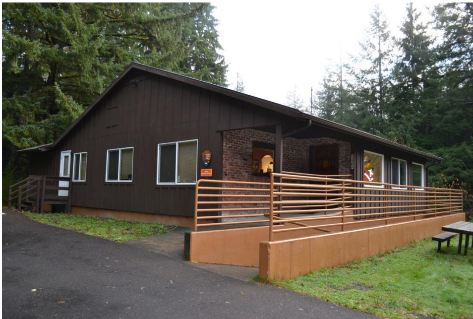
View east toward the principal and side facades of the administrative headquarters building. (WJE/LSHLA)
