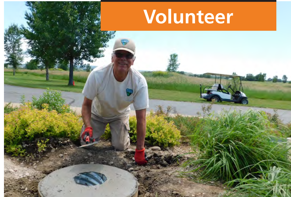
Long-term volunteer Dave Lefevre finishes foundation for new flag pole at Pompeys Pillar National Monument, MT. Photo by Bureau of Land Management.
