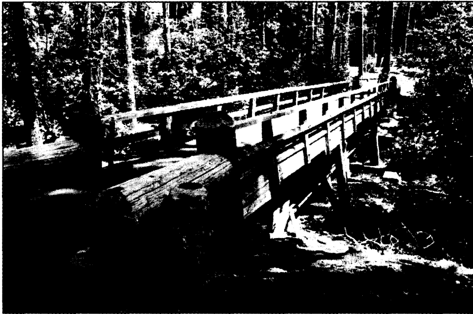
Photo 14: Bridge over Manzanita Creek.
