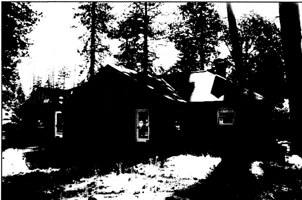
Photo 7: Loomis Residence and Studio, West Elevation
