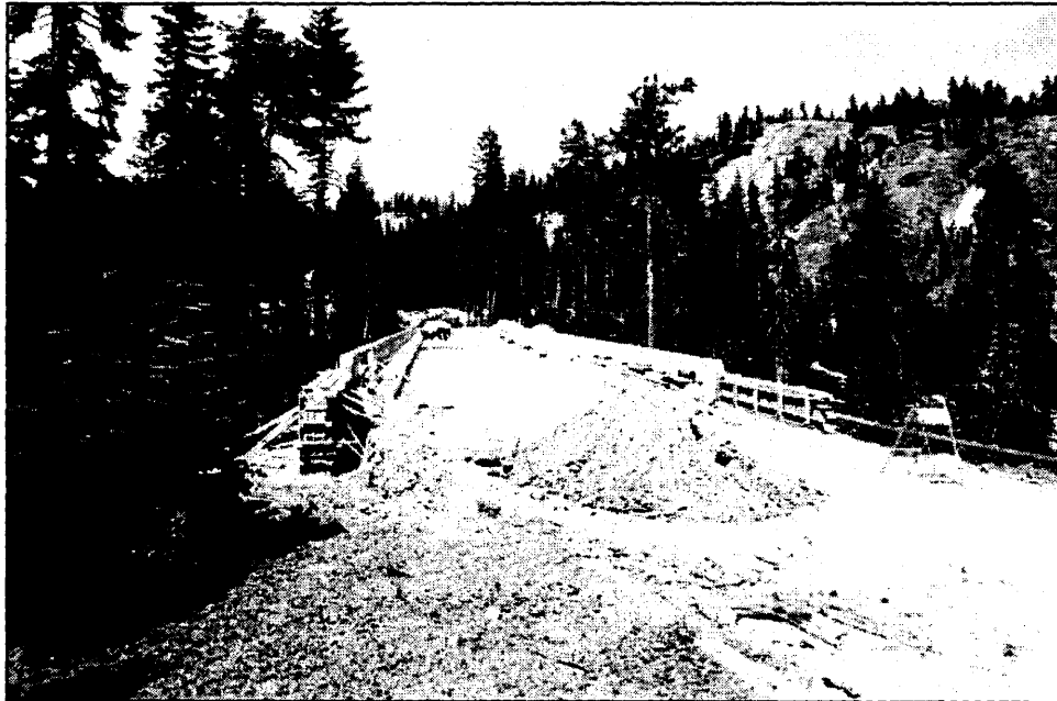
Photo 14: Concrete bridge deck, view to NW.
