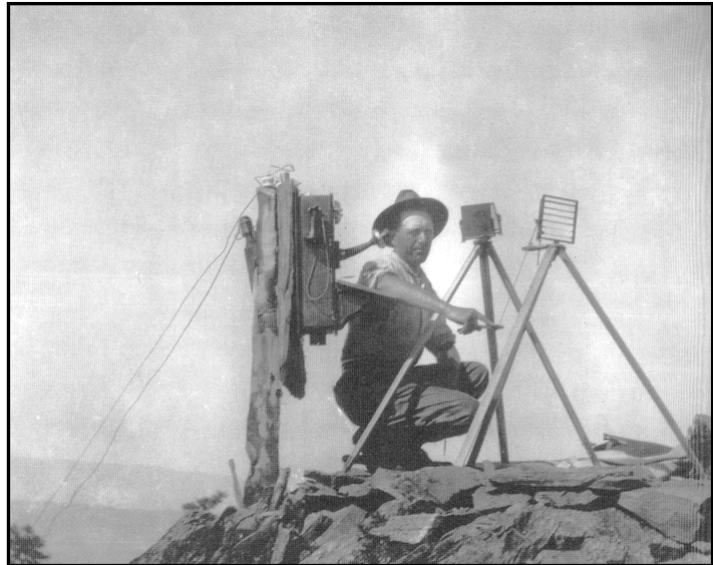
Ranger with heliograph, a communication device that used mirrors and the sun’s rays, 1912. (Source: USDA Forest Service, USDA Forest Service: The First Century , Washington, DC: Government Printing Office, 2000, p. 50.)
