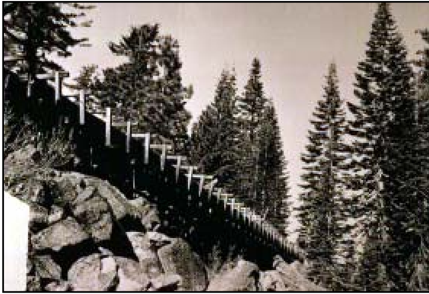
Flume near Sunflower Flat, 1933. (Source: Negative #162.1, Historic Photograph Collection, LAVO).
