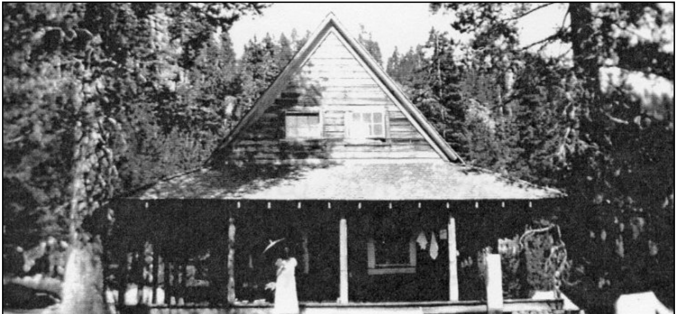
Another view of the improved South Porch and the West Porch addition on the left
