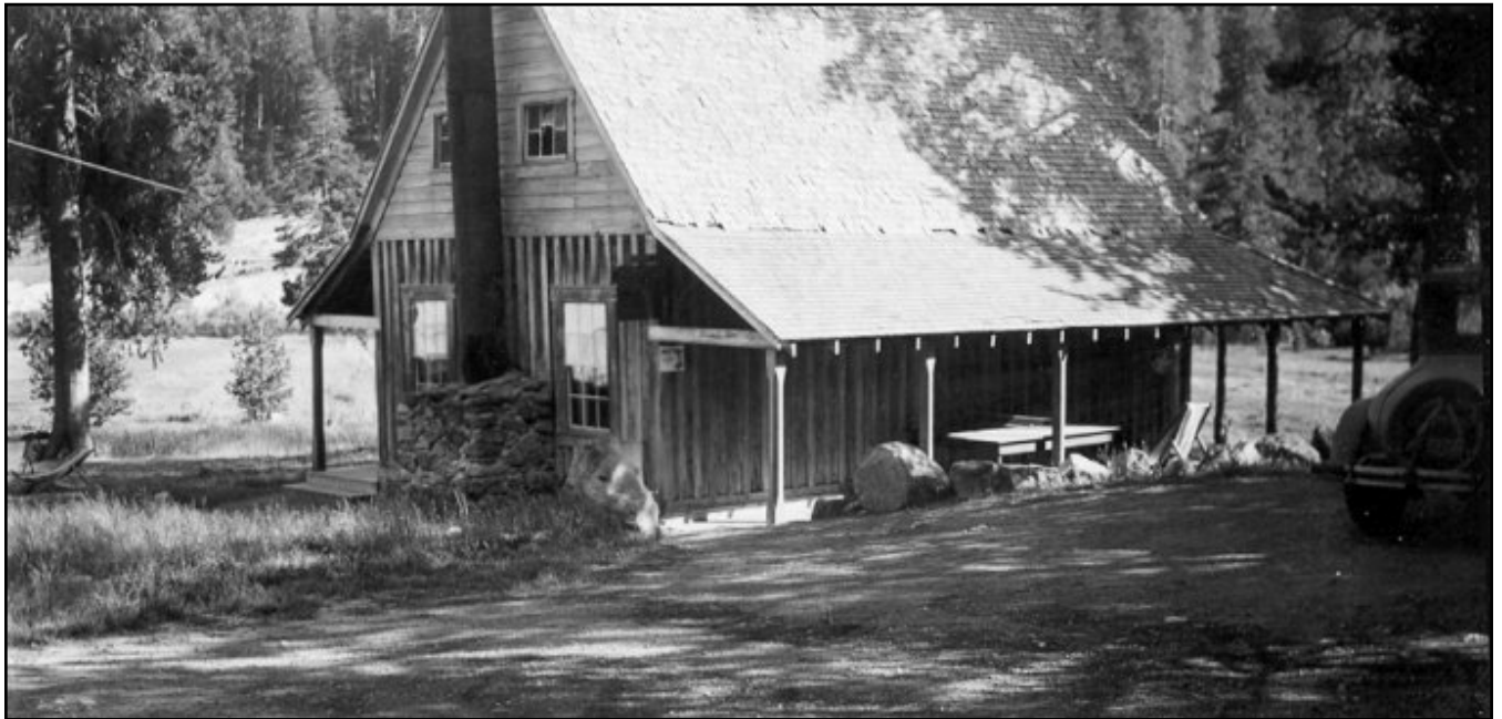
1931 Clearer View of the Earthen Bank at the Rear of the Lodge. (Photograph courtesy of Susan Watson)
