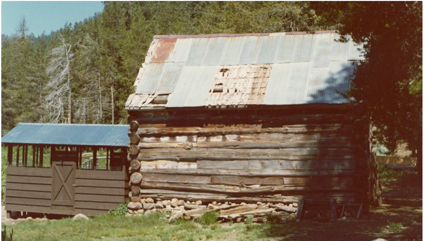
1975--Log barn with old shed replaced by a modern structure
