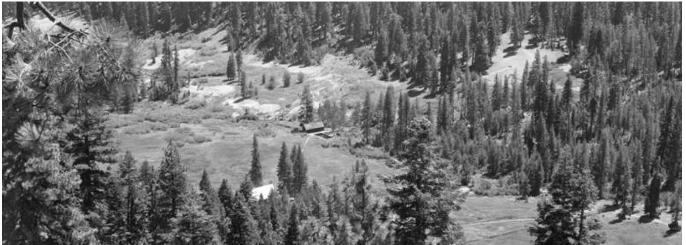
Sifford bath house and the rock and concrete plunge in 1938
