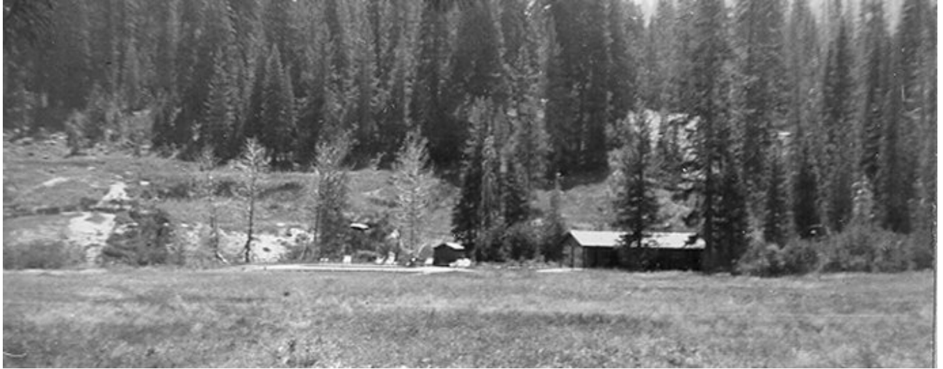
1963--Construction of new bath house completed and old Sifford bath house removed (Photograph courtesy of Susan Watson)
