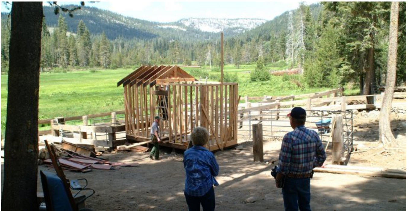
Rebuilding the Tack Shed in June 2003
