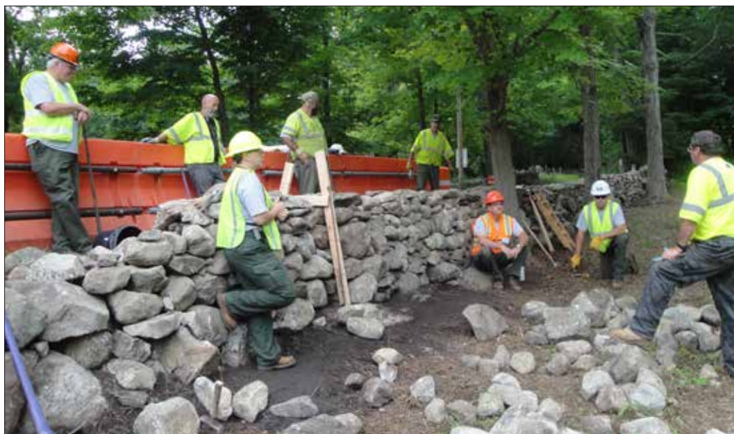
Participants learning about historic stone wall construction, repair and maintenance during a workshop held at Weir Farm National Historic Site. (OCLP)
