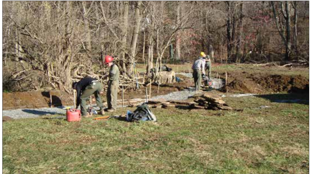
Rehabilitating a historic trail at Valley Forge National Historical Park. (OCLP)
