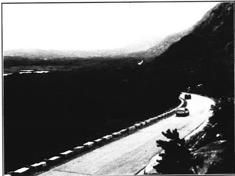
Historic Motor Road, Acadia National Park. The Olmsted Center has prepared a number of studies for the Motor Road including design guidelines for Federal Highways Administration rehabilitation work.
