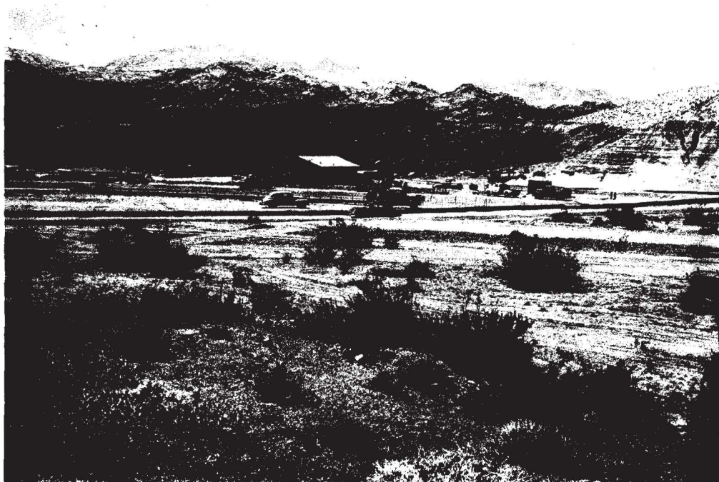
Plate 12 (Lower)--View of Parking Area and Road Construction at Katherine. Concessioner cafe shown during construction
