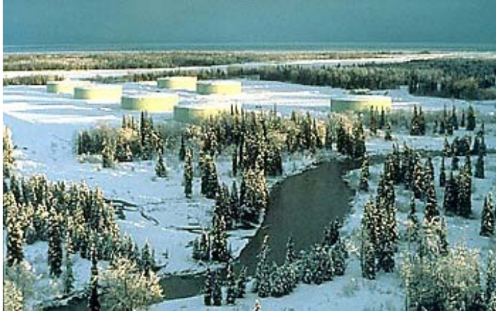
Figure 43. The oil storage tanks of the Drift River oil storage facility located along the banks of the Drift River. Photograph by J. Major in 1990 (USGS Volcano Hazards Program, http://volcanoes.usgs.gov/Images/Jpg/Redoubt/30210600_023_large.jpg )
