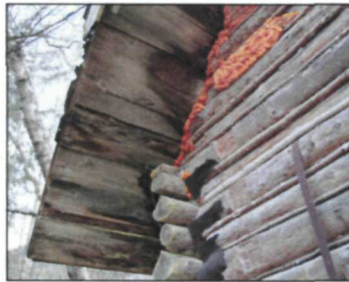
Figure 88. Biological growth, north elevation, photographed by Kathleen Wackrow, NPS, April 2016 (NPS, AKRO, Historic Architecture, Patterson Cabin Digital Files).
