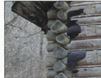
Figure 57. Remnants of former shed roofed kitchen addition, north elevation, photographed by Kathleen Wackrow, NPS, April 2016 (NPS, AKRO, Historic Architecture, Patterson Cabin Digital Files).
