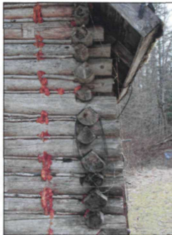
Figure 59. Utility wire, north elevation, photographed by Kathleen Wackrow, NPS, April 2016 (NPS, AKRO, Historic Architecture, Patterson Cabin Digital Files).
