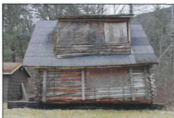
Figure 61. West elevation, photographed by Kathleen Wackrow, NPS, April 2016 (NPS, AKRO, Historic Architecture, Patterson Cabin Digital Files).
