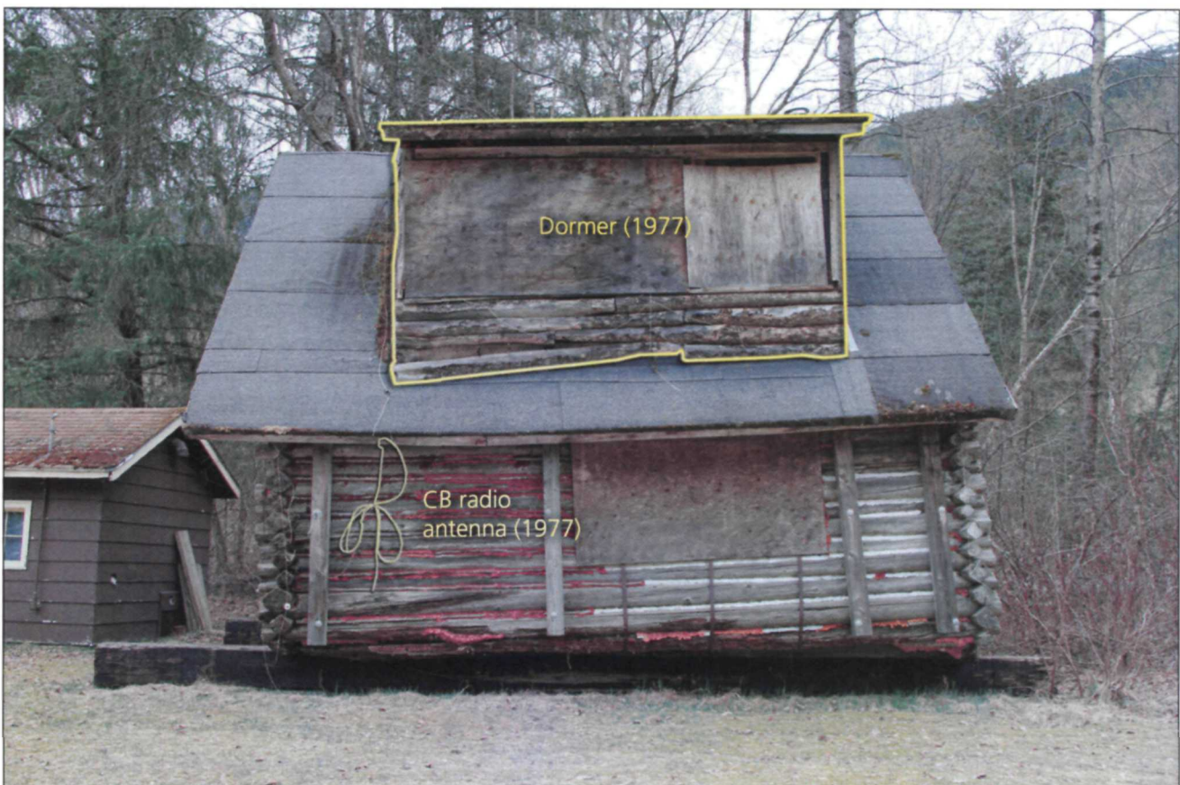
McDermott Era Modifications, West Elevation.
