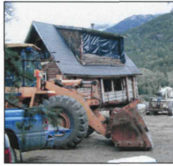
Figure 43. Patterson Cabin relocation from McDermott property to NPS property, unknown photographer, September 2002 (NPS, AKRO, Historic Architecture, Patterson Cabin Digital Files).
