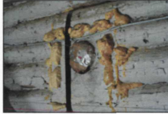
Figure 71. Wall thimble, south wall, photographed by Kathleen Wackrow, NPS, April 2016 (NPS, AKRO, Historic Architecture, Patterson Cabin Digital Files).
