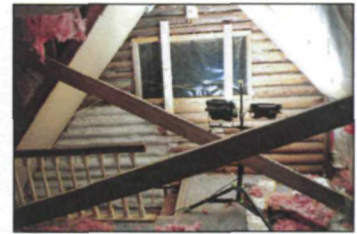
Figure 81. Second floor (attic), photographed by Kathleen Wackrow NPS, April 2016 (NPS, AKRO, Historic Architecture, Patterson Cabin Digital Files).
