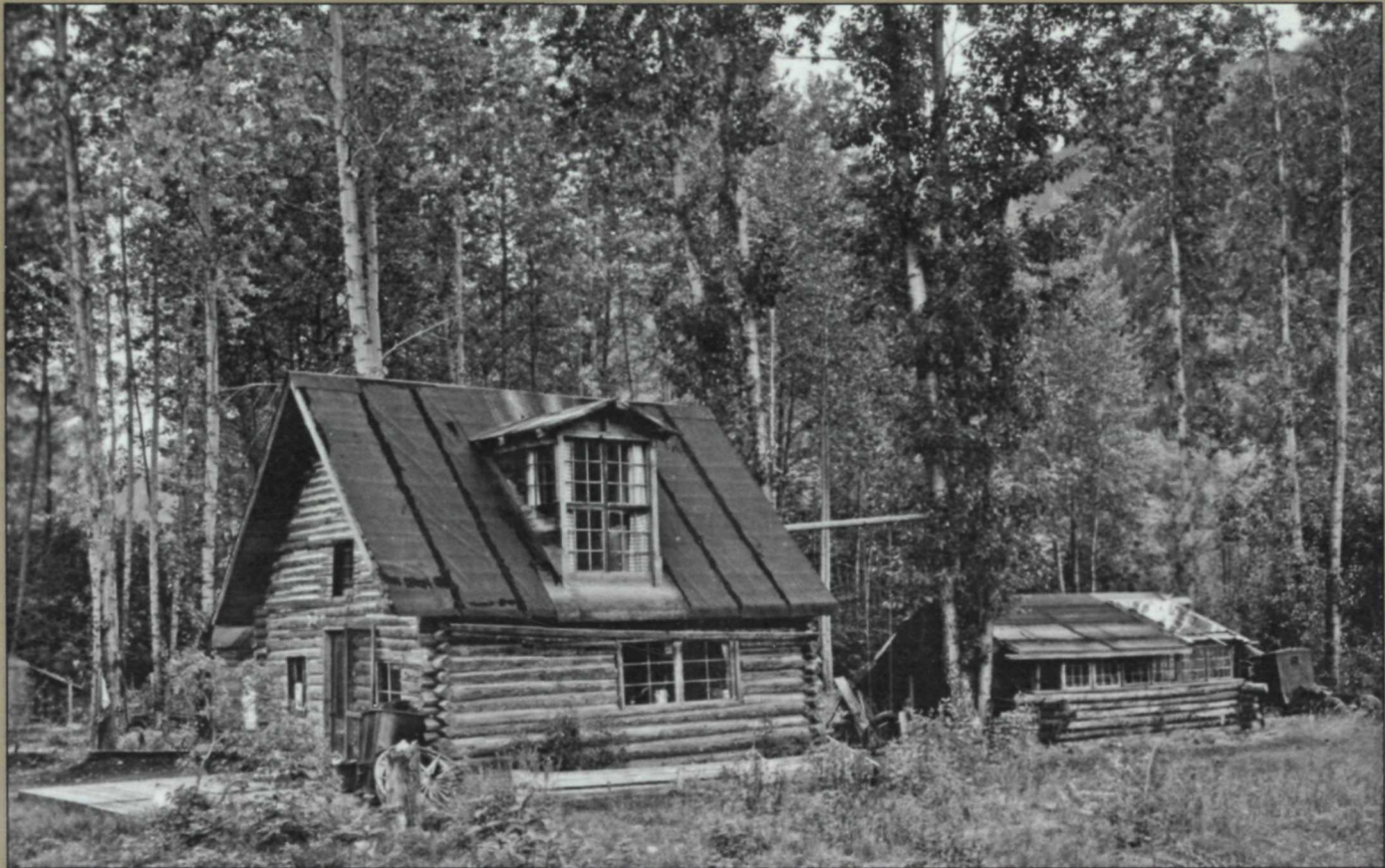
Patterson Cabin, north and east elevations (586-85), photographed by Hunter Gruening, September 1952 (NPS, KLGO, Steve Hites Collection).
