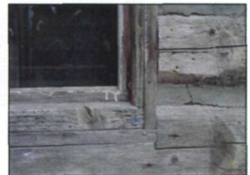
Figure 48. Hewn ends of logs abutting fenestration, photographed by Kathleen Wackrow, NPS, April 2016 (NPS, AKRO, Historic Architecture, Patterson Cabin Digital Files).
