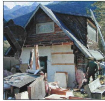
Figure 41. Patterson Cabin relocation from McDermott property to NPS property, unknown photographer, September 2002 (NPS, AKRO, Historic Architecture, Patterson Cabin Digital Files).
