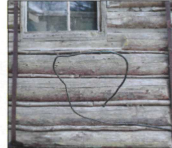
Figure 60. Copper Propane Pipe, north elevation, photographed by Kathleen Wackrow, NPS, April 2016 (NPS, AKRO, Historic Architecture, Patterson Cabin Digital Files).
