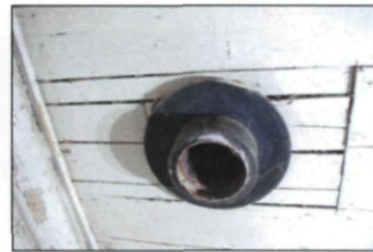
Figure 72. Wall thimble, southwest corner of ceiling, photographed by Kathleen Wackrow, NPS, April 2016 (NPS, AKRO, Historic Architecture, Patterson Cabin Digital Files).
