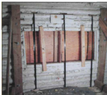
Figure 73. East wall, photographed by Kathleen Wackrow, NPS, April 2016 (NPS, AKRO, Historic Architecture, Patterson Cabin Digital Files).
