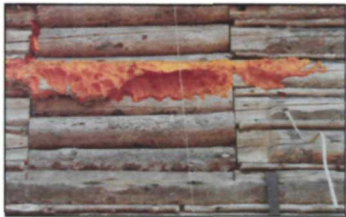
Figure 55. Barked and peeled logs, north elevation, photographed by Kathleen Wackrow, NPS, April 2016 (NPS, AKRO, Historic Architecture, Patterson Cabin Digital Files).
