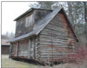
Figure 64. South elevation, photographed by Kathleen Wackrow, NPS, April 2016 (NPS, AKRO, Historic Architecture, Patterson Cabin Digital Files).
