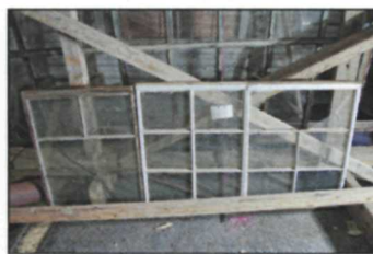
Figure 62. First floor windows, west elevation, photographed by Kathleen Wackrow, NPS, April 2016 (NPS, AKRO, Historic Architecture, Patterson Cabin Digital Files).
