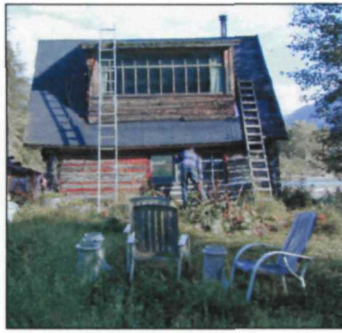
Figure 40. Patterson Cabin relocation from McDermott property to NPS property, unknown photographer, September 2002 (NPS, AKRO, Historic Architecture, Patterson Cabin Digital Files).
