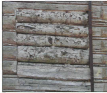
Figure 33. Former first-floor window (to the west), filled-in by McDermotts, north elevation, photographed by Kathleen Wackrow, NPS, April 2016 (NPS, AKRO, Historic Architecture, Patterson Cabin Digital Files).
