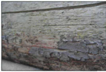
Figure 85. Biological growth, north elevation, photographed by Kathleen Wackrow, NPS, April 2016 (NPS, AKRO, Historic Architecture, Patterson Cabin Digital Files).
