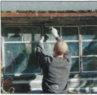
Figure 39. Patterson Cabin relocation from McDermott property to NPS property, unknown photographer, September 2002 (NPS, AKRO, Historic Architecture, Patterson Cabin Digital Files).
