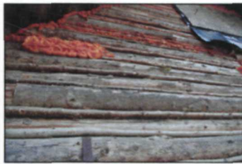
Figure 56. Remnants of former shed roofed kitchen addition, north elevation, photographed by Kathleen Wackrow, NPS, April 2016 (NPS, AKRO, Historic Architecture, Patterson Cabin Digital Files).
