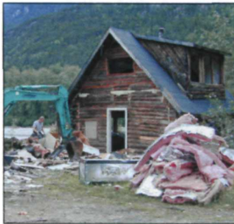
Figure 42. Patterson Cabin relocation from McDermott property to NPS property, unknown photographer, September 2002 (NPS, AKRO, Historic Architecture, Patterson Cabin Digital Files).
