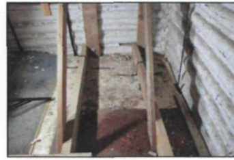
Figure 69. Linoleum flooring, southeast corner, photographed by Kathleen Wackrow, NPS, April 2016 (NPS, AKRO, Historic Architecture, Patterson Cabin Digital Files).
