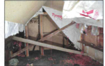
Figure 82. Second floor (attic), photographed by Kathleen Wackrow NPS, April 2016 (NPS, AKRO, Historic Architecture, Patterson Cabin Digital Files).
