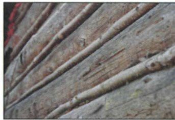
Figure 86. Biological growth, north elevation, photographed by Kathleen Wackrow, NPS, April 2016 (NPS, AKRO, Historic Architecture, Patterson Cabin Digital Files).
