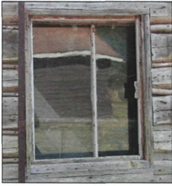
Figure 52. East window, north elevation, photographed by Kathleen Wackrow, NPS, April 2016 (NPS, AKRO, Historic Architecture, Patterson Cabin Digital Files).
