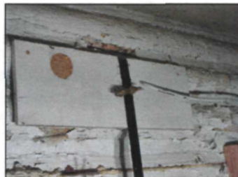
Figure 74. Remnant of propane lighting, photographed by Kathleen Wackrow NPS, April 2016 (NPS, AKRO, Historic Architecture, Patterson Cabin Digital Files).
