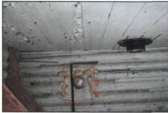
Figure 70. Wall thimbles, southeast corner, photographed by Kathleen Wackrow, NPS, April 2016 (NPS, AKRO, Historic Architecture, Patterson Cabin Digital Files).
