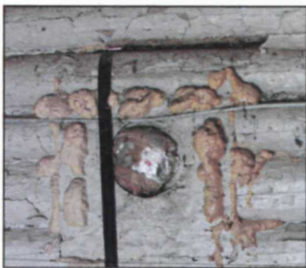
Figure 22. Interior portion of wall thimble, remnant from Patterson era stovepipe, photographed by Kathleen Wackrow, NPS, April 2016 (NPS, AKRO, Historic Architecture, Patterson Cabin Digital Files).
