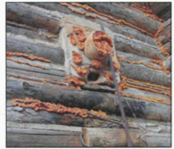
Figure 23. Exterior portion of wall thimble, remnant from Patterson era stovepipe, photographed by Kathleen Kathleen Wackrow, NPS, April 2016 (NPS, AKRO, Historic Architecture, Patterson Cabin Digital Files).
