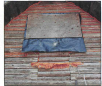
Figure 35. Former second-floor window, filled-in by McDermotts, north elevation, photographed by Kathleen Wackrow, NPS, April 2016 (NPS, AKRO, Historic Architecture, Patterson Cabin Digital Files).
