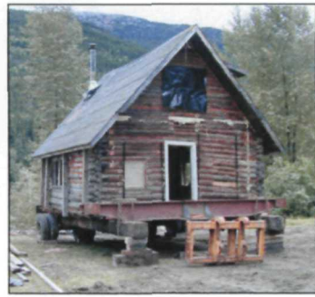
Figure 44. Patterson Cabin relocation from McDermott property to NPS property, unknown photographer, September 2002 (NPS, AKRO, Historic Architecture, Patterson Cabin Digital Files).
