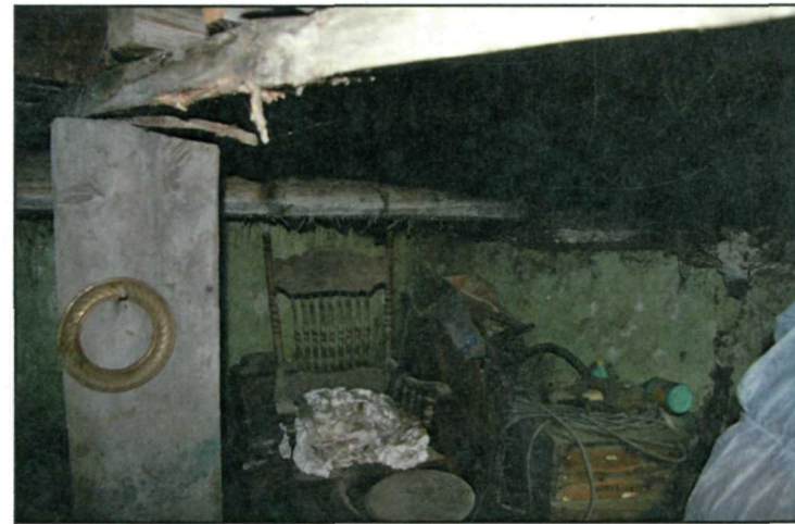
Figure 74: Crawl Space A section A-2 cellar with log sill atop concrete walls. Note central support post in left foreground (NPS July 2008).
