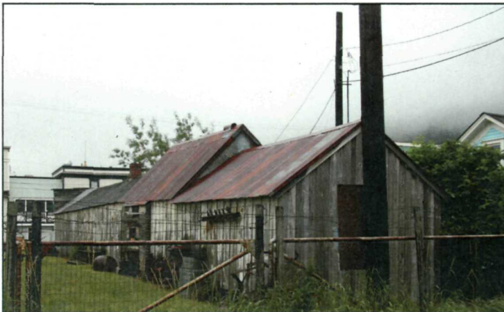
Figure 53: Jeff. Smiths Parlor Museum building, south and west elevations. (NPS July 23, 2008)
