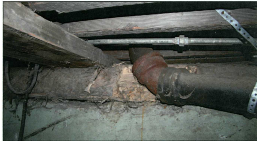
Figure 110: Log foundation along west wall of section A-2 (NPS July 2008).
