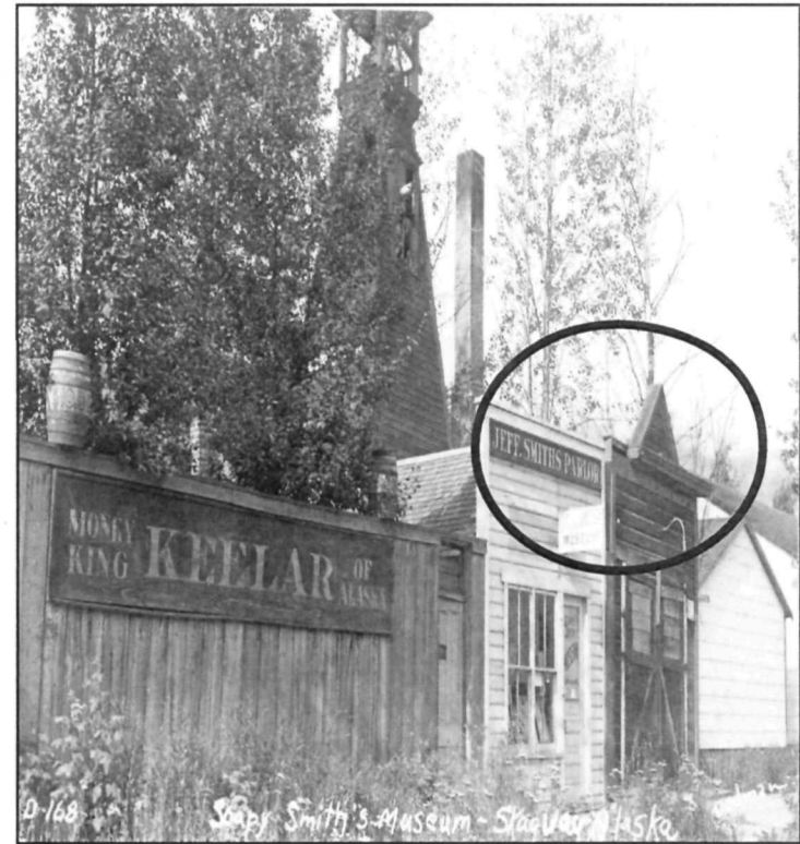
Figure 19: Museum building after 1935 with adjacent Hose House. Circled area highlights the original cut in cornice from when the buildings were located on the north side of Sixth Avenue (Dedman's Photo Shop; KLGO, 6th32-1641).
