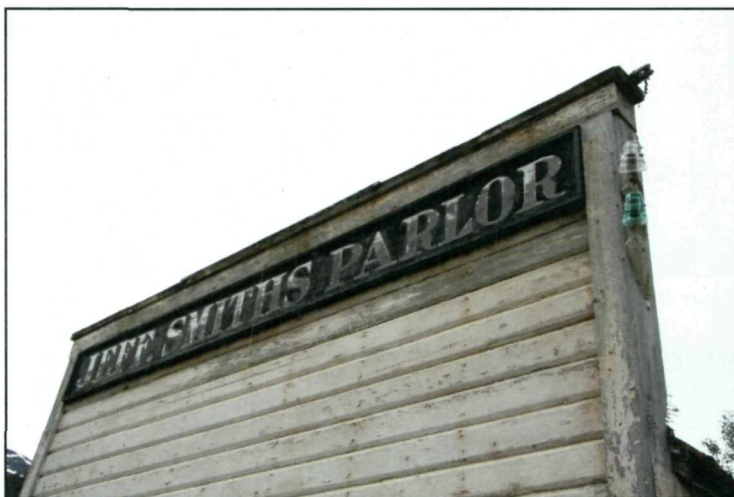
Figure 79: False front with painted sign, north elevation. The green glass insulator probably came from the Chilkoot Trail. (NPS July 2008).
