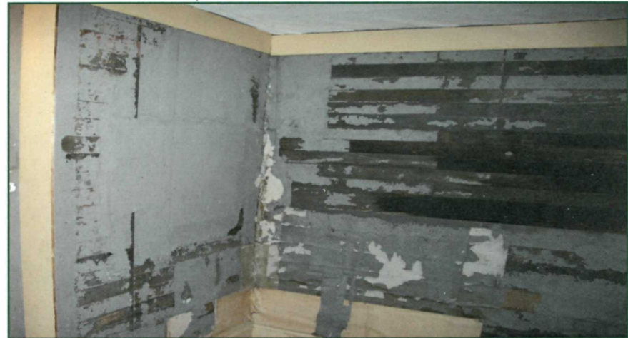
Figure 131: Same corner of A-1 after museum curatorial staff stripped the wall, only felted sheet cardboard remains on walls (NPS July 2009).
