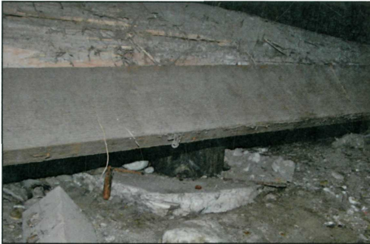
Figure 73: Crawl Space A, section A-1 looking west at log foundation supported by cut log on concrete pier (NPS July 2008).
