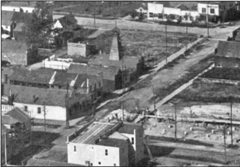
Figure 17: Hose House (note tower) and the Hook and Ladder Company shed on the south side of Sixth Avenue ca. 1916, new Bank of Alaska foundations shown in the lower right hand part of the photograph (Alaska State Library, print # PCA 25-8; KLGO SO-136-5470).
