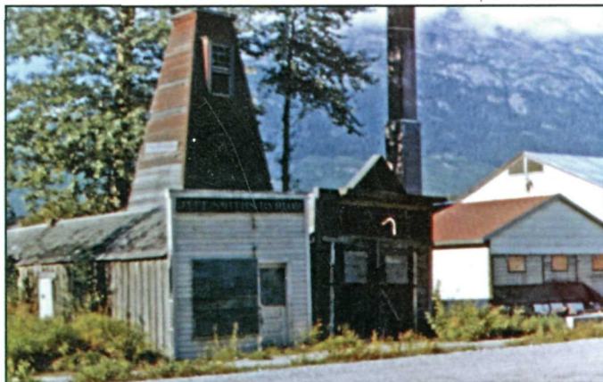
Figure 44: Jeff. Smiths Parlor Museum building, on the south side of 6th Avenue (George and Edna Rapuzzi Collection, Rasmuson Foundation, Klondike Gold Rush National Historical Park print inventory #00074).
