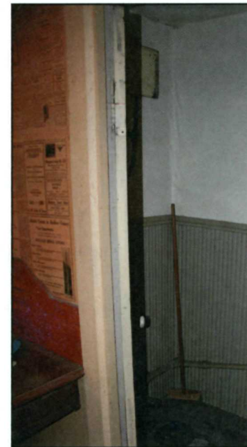
Figure 97: Toilet flange and doorway into bathroom from Room A-1 (NPS July 2008).
