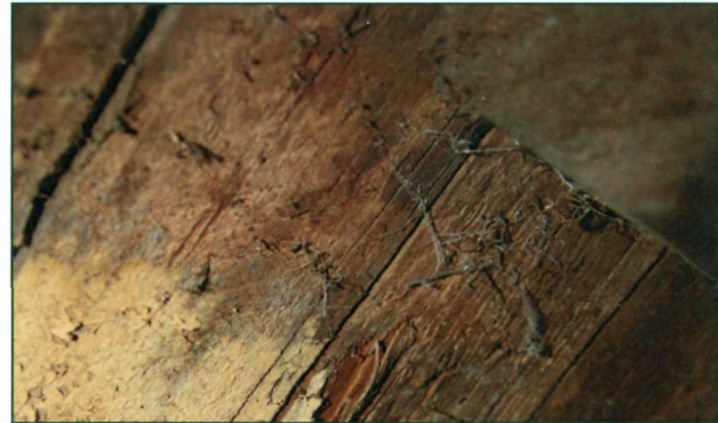
Figure 126: Sub-flooring in A-1 with 3 3/4" x 3/4" boards (NPS July 2009).
