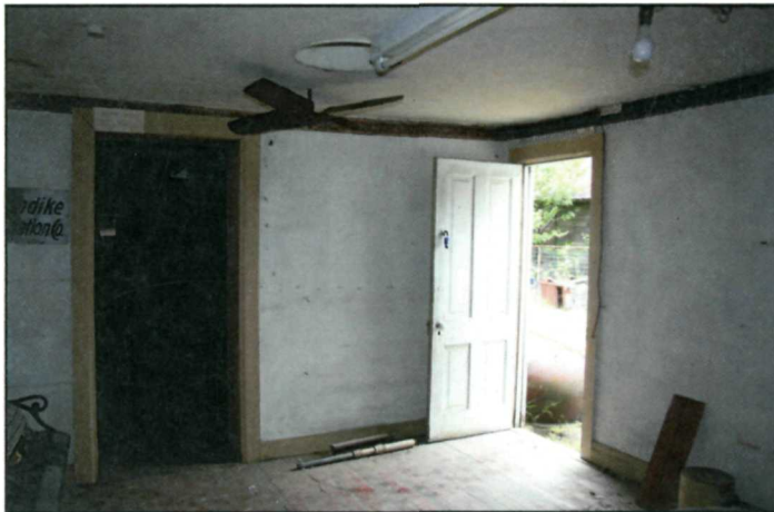
Figure 99: Southwest corner of Room A-2, with felted sheet cardboard still covering walls (NPS July 2008).
