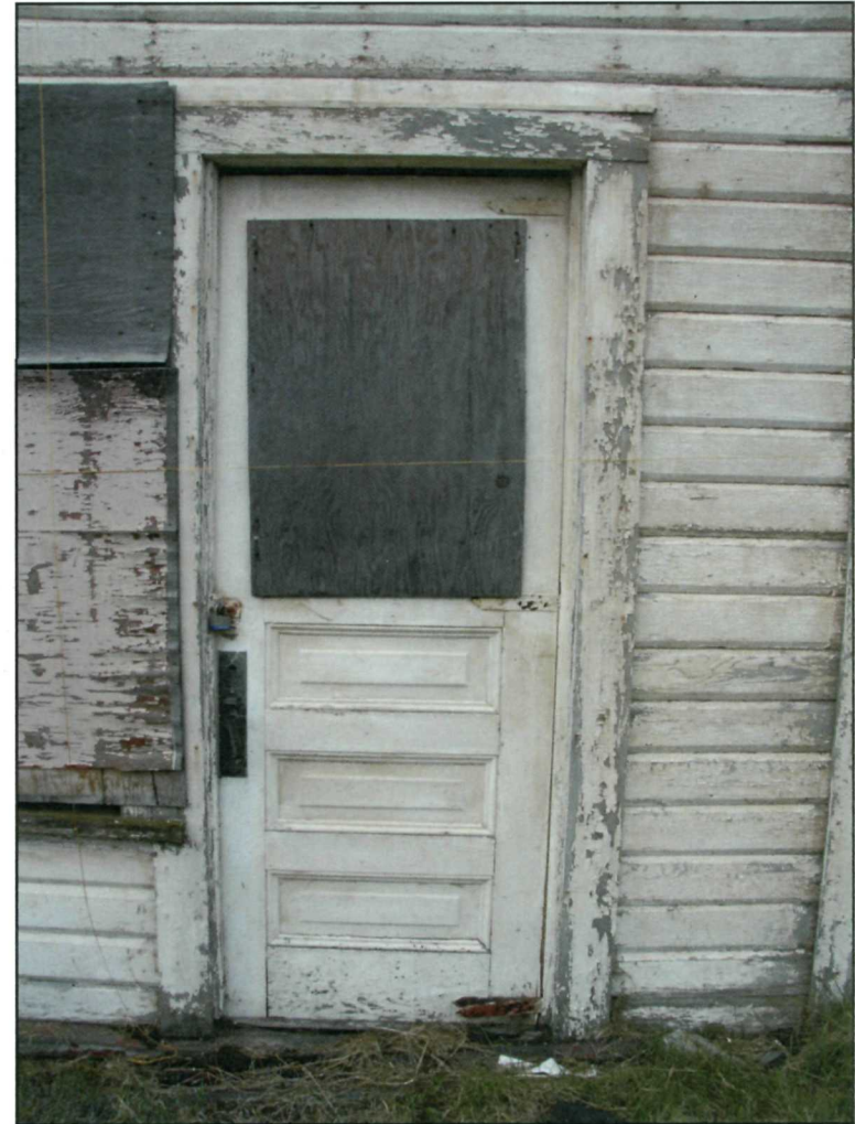
Figure 113: Windows and main doorway on north elevation (NPS July 2008).
