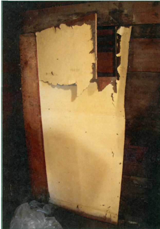
Figures 151 and 152: On the left, a current image of the opening in north wall of Room B that corresponds with the doorway in Figures 136 and 137. On the right, a close-up view behind the piece of wood covering the opening. Note the horizontal boards covering the exterior of the opening (NPS July 2009).
