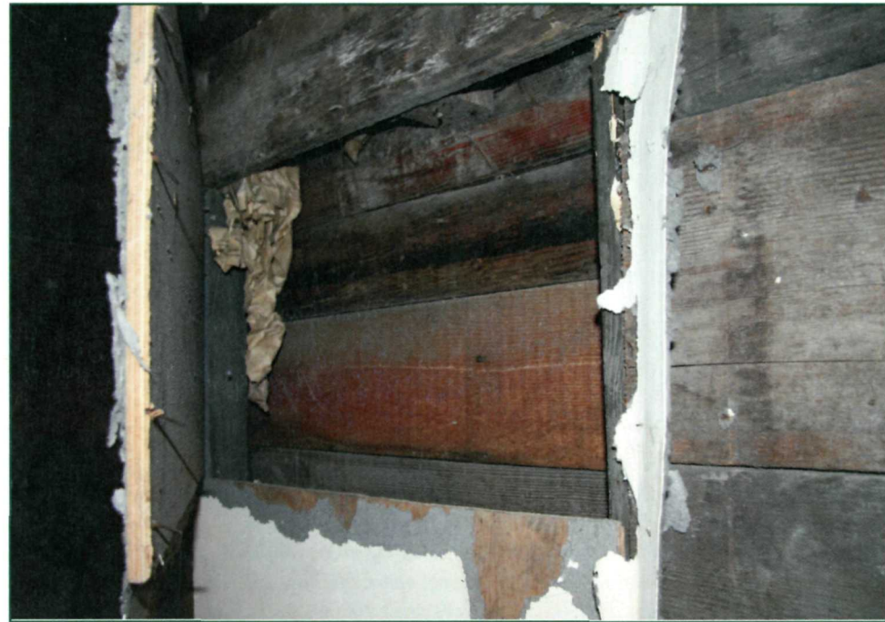
Figures 151 and 152: On the left, a current image of the opening in north wall of Room B that corresponds with the doorway in Figures 136 and 137. On the right, a close-up view behind the piece of wood covering the opening. Note the horizontal boards covering the exterior of the opening (NPS July 2009).
