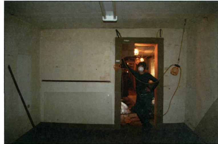
Figure 100: North wall of Room B and doorway from Room A-2, walls have since been stripped to bare wooden beams. Haruna Madono in doorway. (NPS July 2008).
