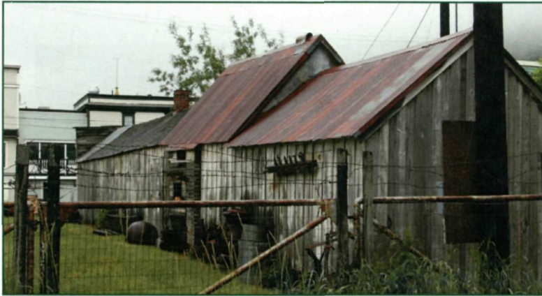
Figure 86: Parlor museum roof, view from southwest (NPS July 2008).
