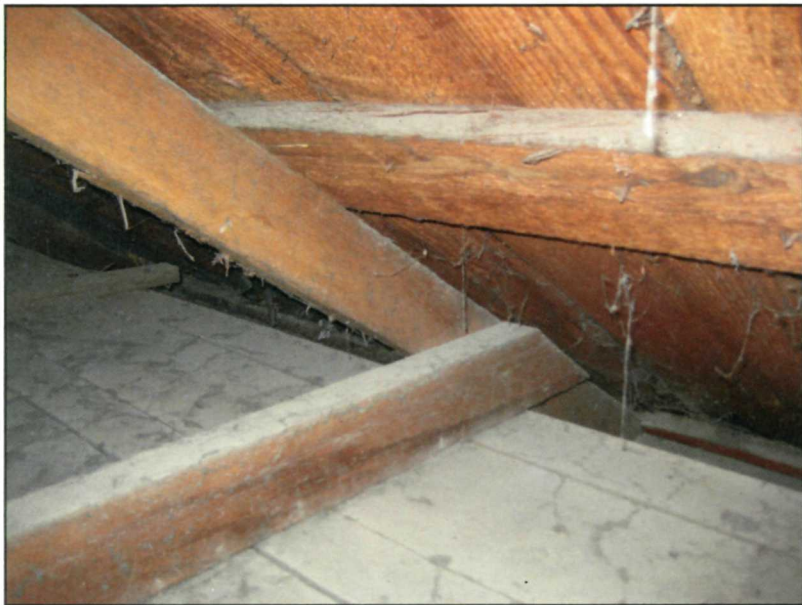
Figure 122: Attic C rafters and collar ties (NPS July 2008).
