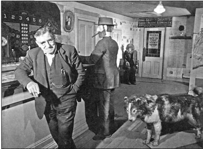
Figure 30: Interior of Jeff. Smiths Parlor Museum, ca. 1940s. Jack Greisbach is pictured in the foreground, Soapy manikin at center and the Dangerous Dan manikin in the rear corner. (George and Edna Rapuzzi Collection, Rasmuson Foundation, KLGO, print inventory #00080).
