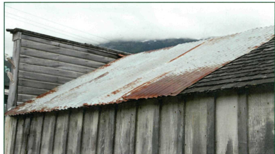
Figure 117: Metal gable roof with cedar shingles, section A northwest elevation (NPS July 2009).
