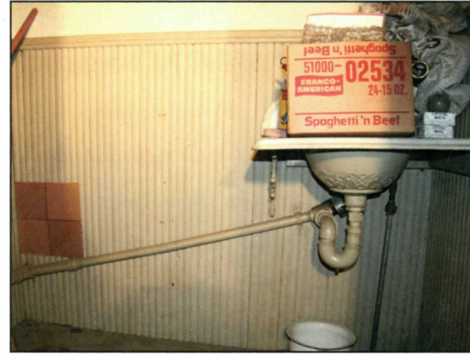
Figure 140: Sink and plumbing in bathroom (NPS July 2008).
