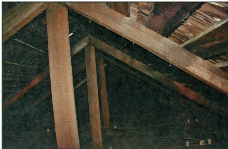
Figure 119: Attic A-1 rafters and skip sheathing (NPS July 2008).
