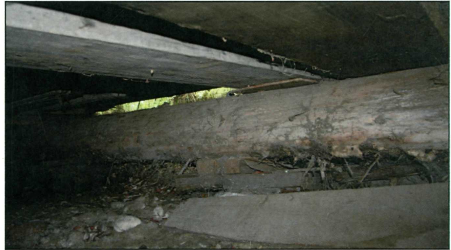
Figure 109: Log foundation along east wall of section A-1 (NPS July 2008).
