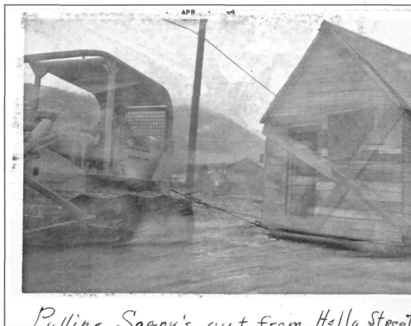
Figure 150: The rear portion of the Jeff. Smiths Parlor Museum building (Rooms B and C). Note the clearly altered eave (in the upper right hand corner of the photo) that would accommodate connection to the front half parlor museum. This photograph shows the building being dragged from 6th Avenue to its current location on 2nd Avenue (George and Edna Rapuzzi Collection, Rasmuson Foundation, KLGO, inventory print #00081.029).
