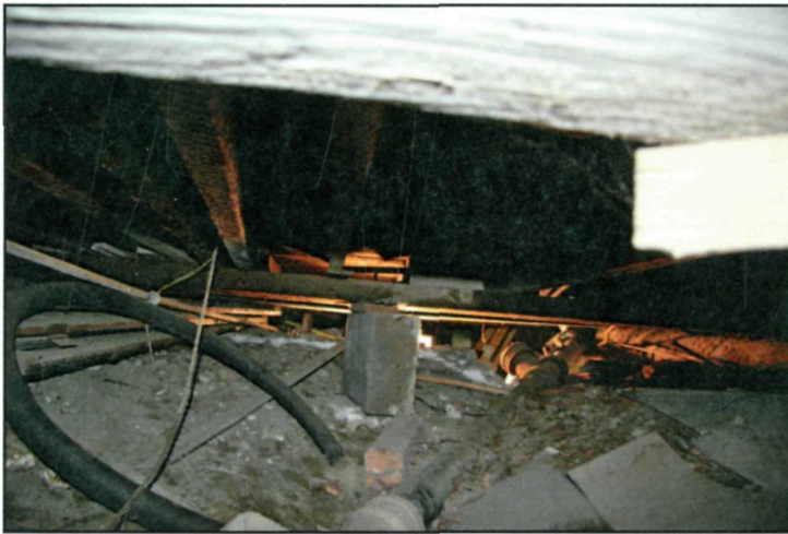
Figure 75: Crawl Space A, section A-1 looking south toward Crawl A section A-2 (NPS July 2008).
