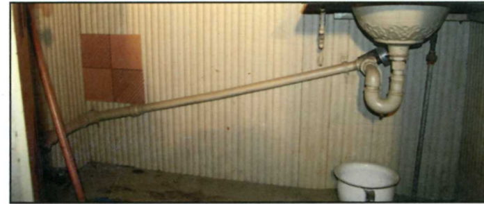
Figure 96: Painted beadboard and porcelain sink in bathroom (NPS July 2008).
