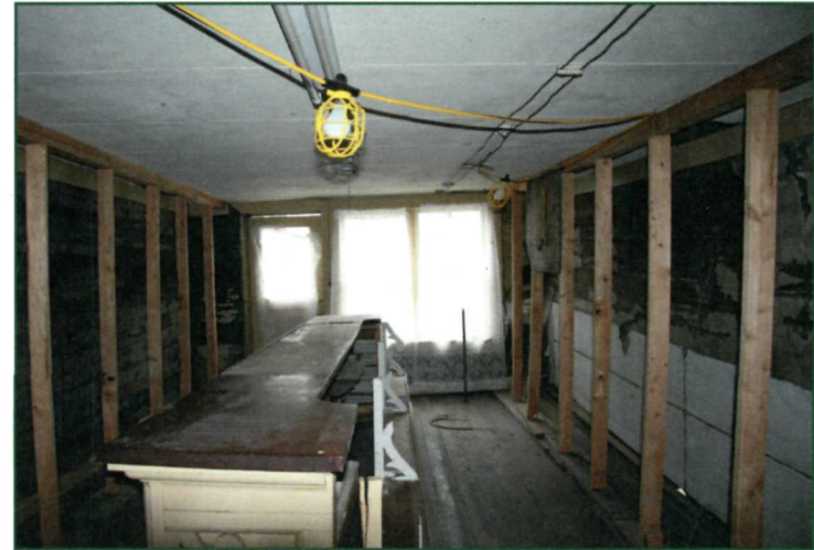
Figure 136: Bar in Room A-1, view to the north (NPS July 2009).
