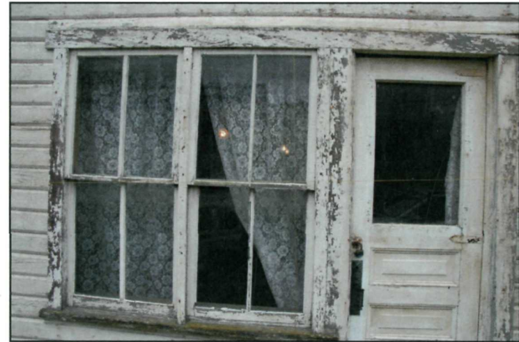
Figure 77: North elevation windows and door (NPS July 2008).
