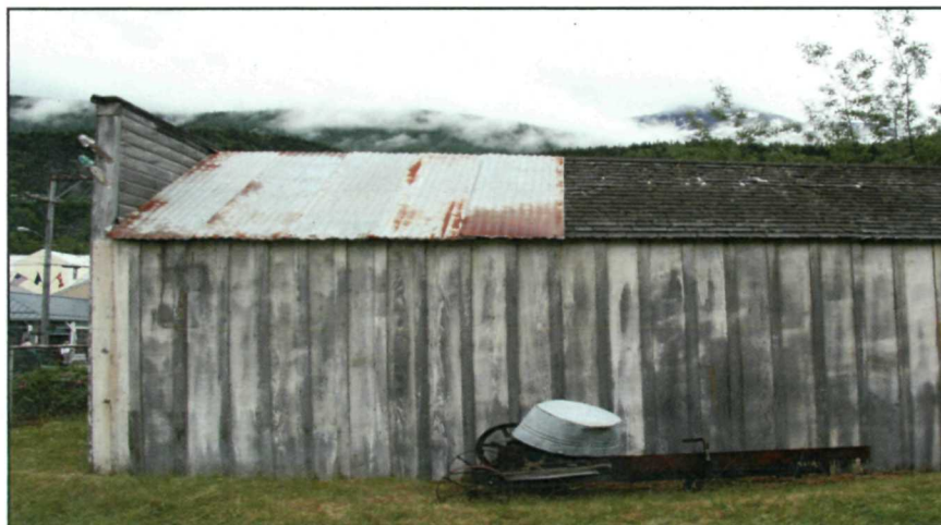
Figure 112: West facade with vertical board and batten siding (NPS July 2008).
