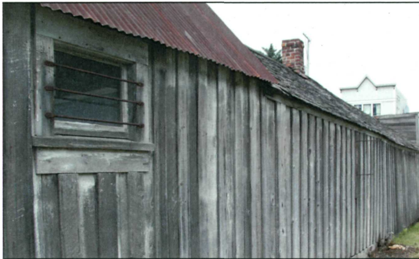
Figure 115: Window with metal bars on east elevation (NPS July 2009).
