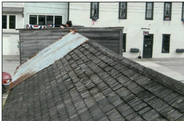
Figure 92: View of roof looking north toward back of false front, Haruna Madono looking over the false front. (NPS July 2008).
