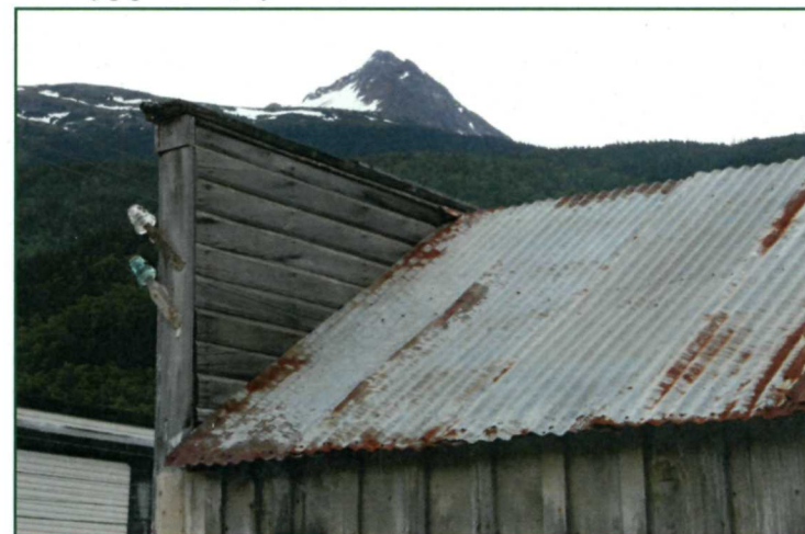
Figure 93: Northwest end of roof section A and back of false front (NPS July 2008).
