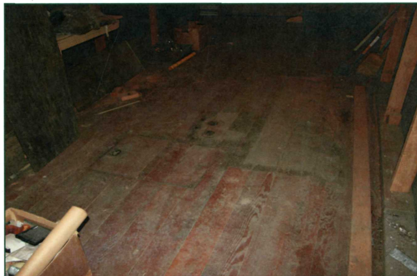
Figure 124: Tongue and groove flooring in Room A-1 with view of flush mounted trap door (NPS July 2008).
