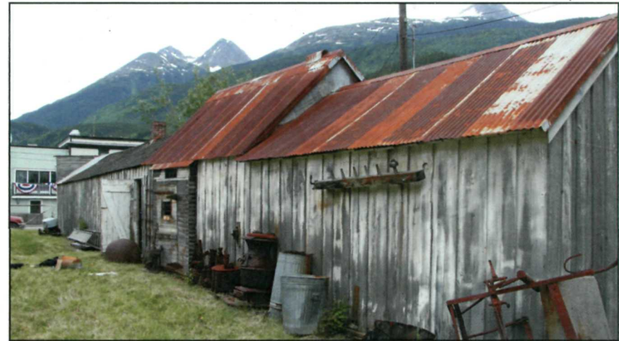
Figure 116: Metal gable roof of section B and C southwest elevation (NPS July 2008).
