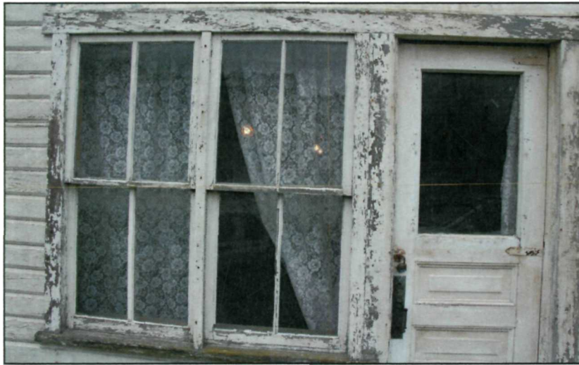
Figure 114: Windows and main doorway on north elevation (NPS July 2008).
