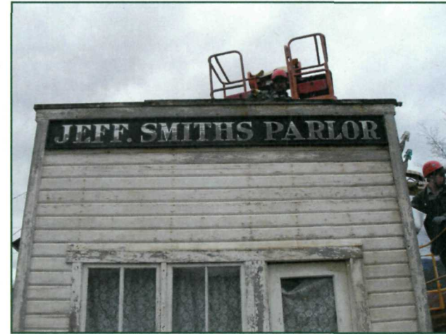
Figure 52: Jeff. Smiths Parlor Museum building, False-front, north elevation, Park Maintenance Staff installing temporary roof. Samuel Boggs, left, Cody Lewis, right. (NPS October 2009).
