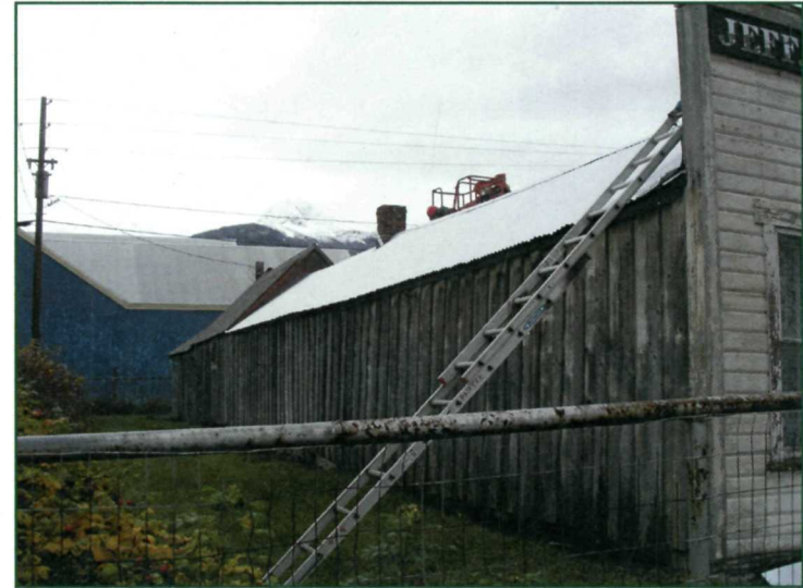
Figure 89: Temporary roof being installed (NPS October 2009)
