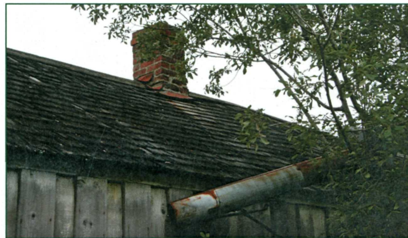
Figure 91: East slope of roof section A, masonry chimney and detached chimney pipe (NPS July 2008).
