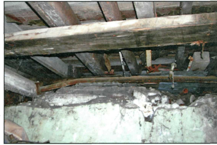
Figure 76: Crawl Space A, section A-2 cellar south wall looking toward Crawl B (NPS July 2008).
