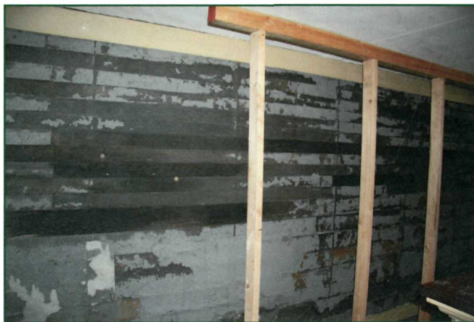
Figure 129: Same west wall of A-1 after museum curators stripped wall (NPS July 2009).
