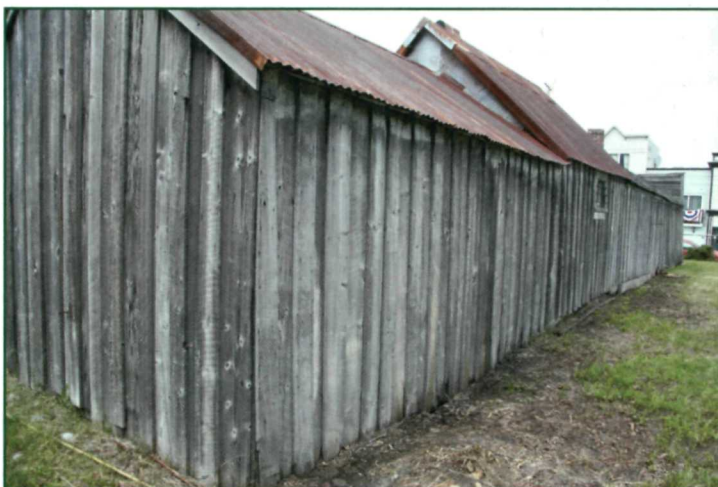
Figure 70: Jeff. Smiths Parlor Museum southeast corner, bushes removed (NPS October 2009).
