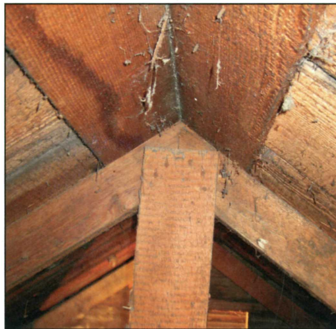
Figure 123: Attic C ridge line, rafters and collar ties (NPS July 2008).
