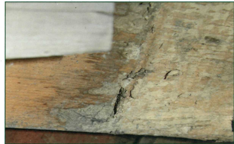
Figure 127: Sub-flooring in small section of A-1 with spaced out, newer 5" boards (NPS July 2009).
