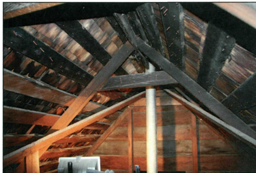
Figure 121: Attic B ridge board, rafters and collar ties (NPS July 2008).
