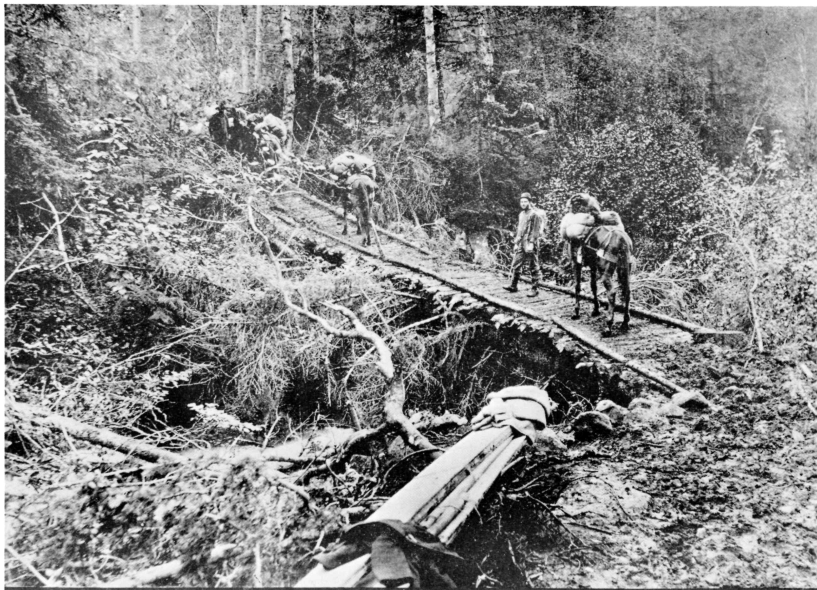
2070. Bridge over Porcupine Creek, Skaguay Trail.
