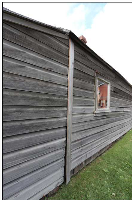
Figure 2: Alaska Street Crib, showing siding, 2019
