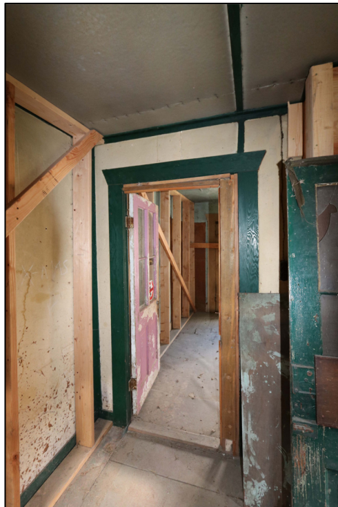
Figure 14: Alaska Street Crib, back chamber showing typical framing design, 2019 Source: Field Photograph by John Wachtel, Historical Architect, AKRO, HABS fieldwork, NPS, KLGO, IMG_6696.
