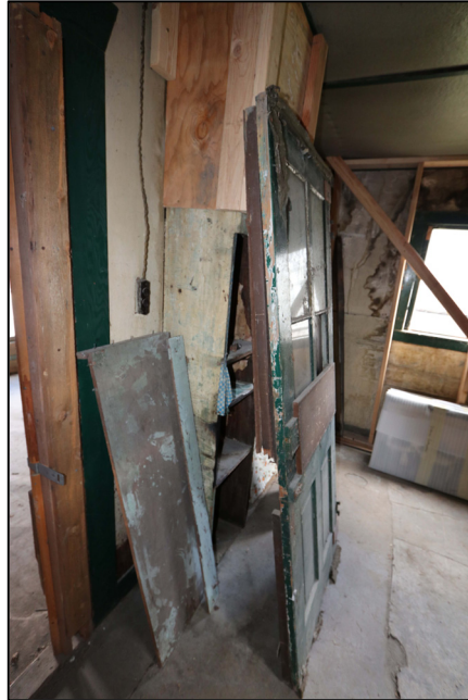
Figure 13: Alaska Street Crib, back chamber showing shelving support for chimney, 2019 Source: Field Photograph by John Wachtel, Historic American Buildings Survey fieldwork, National Park Service, Klondike Gold Rush National Historical Park, IMG_6692.
