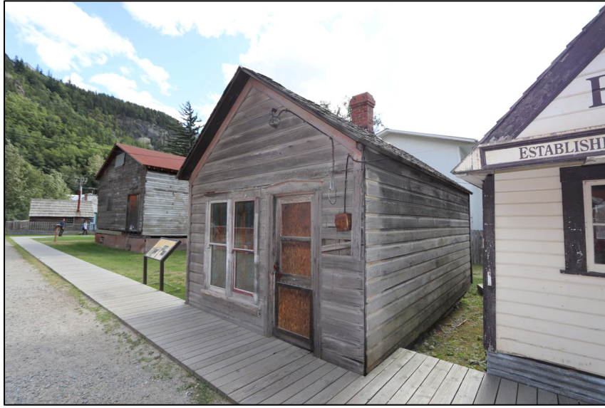
Figure 3: Alaska Street Crib, north elevation, 2019
