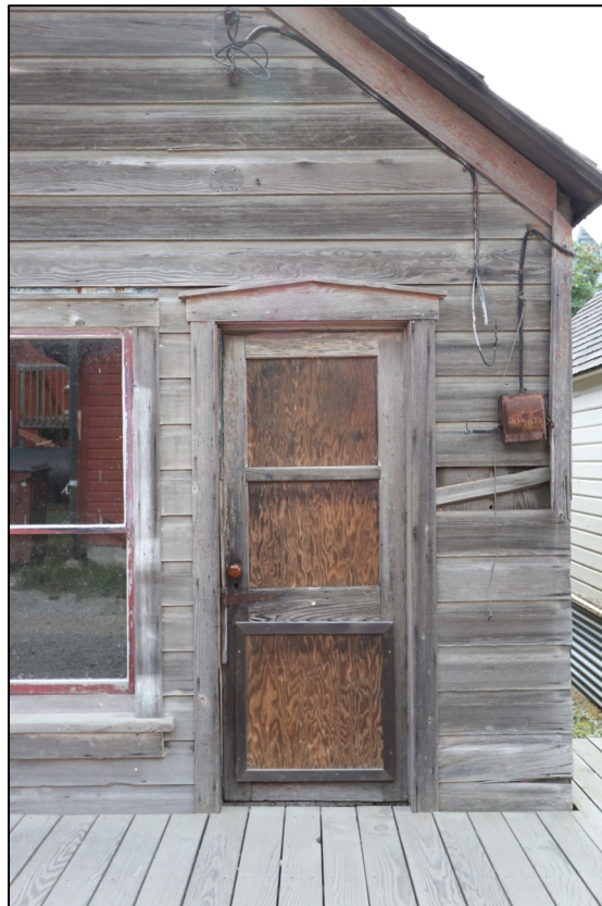
Figure 4: Alaska Street Crib, north elevation door detail, 2019
