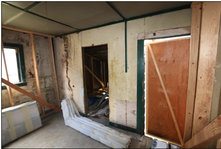
Figure 12: Alaska Street Crib, back Chamber to shed addition showing green trim, 2019 Source: Field Photograph by John Wachtel, Historical Architect, AKRO, HABS fieldwork, NPS, KLGO, IMG_6687.
