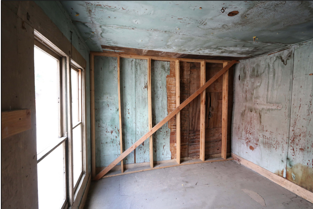
Figure 9: Alaska Street Crib, front chamber looking east, 2019 Source: Field Photograph by John Wachtel, Historical Architect, AKRO, HABS fieldwork, NPS, KLGO, IMG_6700.
