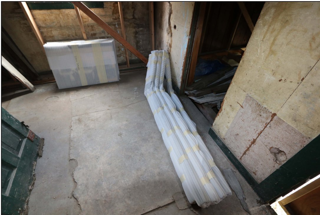
Figure 10: Alaska Street Crib, back chamber floor, 2019 Source: Field Photograph by John Wachtel, Historical Architect, AKRO, HABS fieldwork, NPS, KLGO, IMG_6689.
