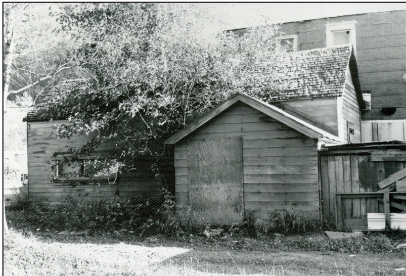
Figure 4: Goldberg Cigar Store and Confectionery on Block 1, Lot 2, in 1979. Image shows gable roof addition.
