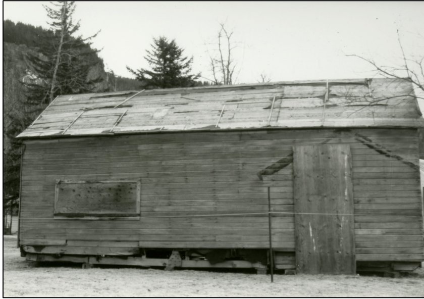
Figure 5: Ghost of gable roof addition, March 1990.
