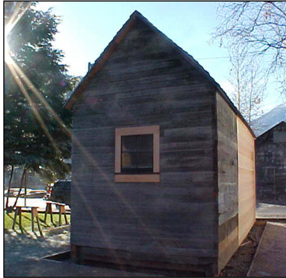
Figure 3: Rear elevation of Goldberg Cigar Store and Confectionery taken after completion of NPS 2002 stabilization work. Of note, at this time the building was located on the north side of Fifth Avenue east of Broadway.
