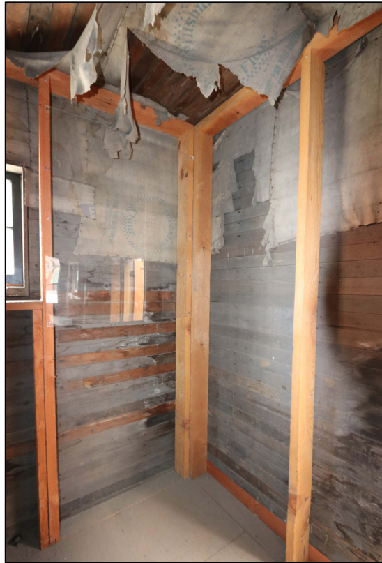
Figure 7: Pillsbury flour sacks on interior walls.
