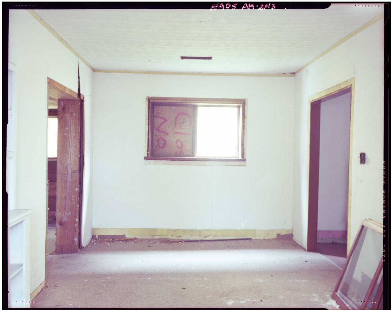
Fig. 4. Dining room looking southeast. (Photographer: Robert Lyon, 2015)
