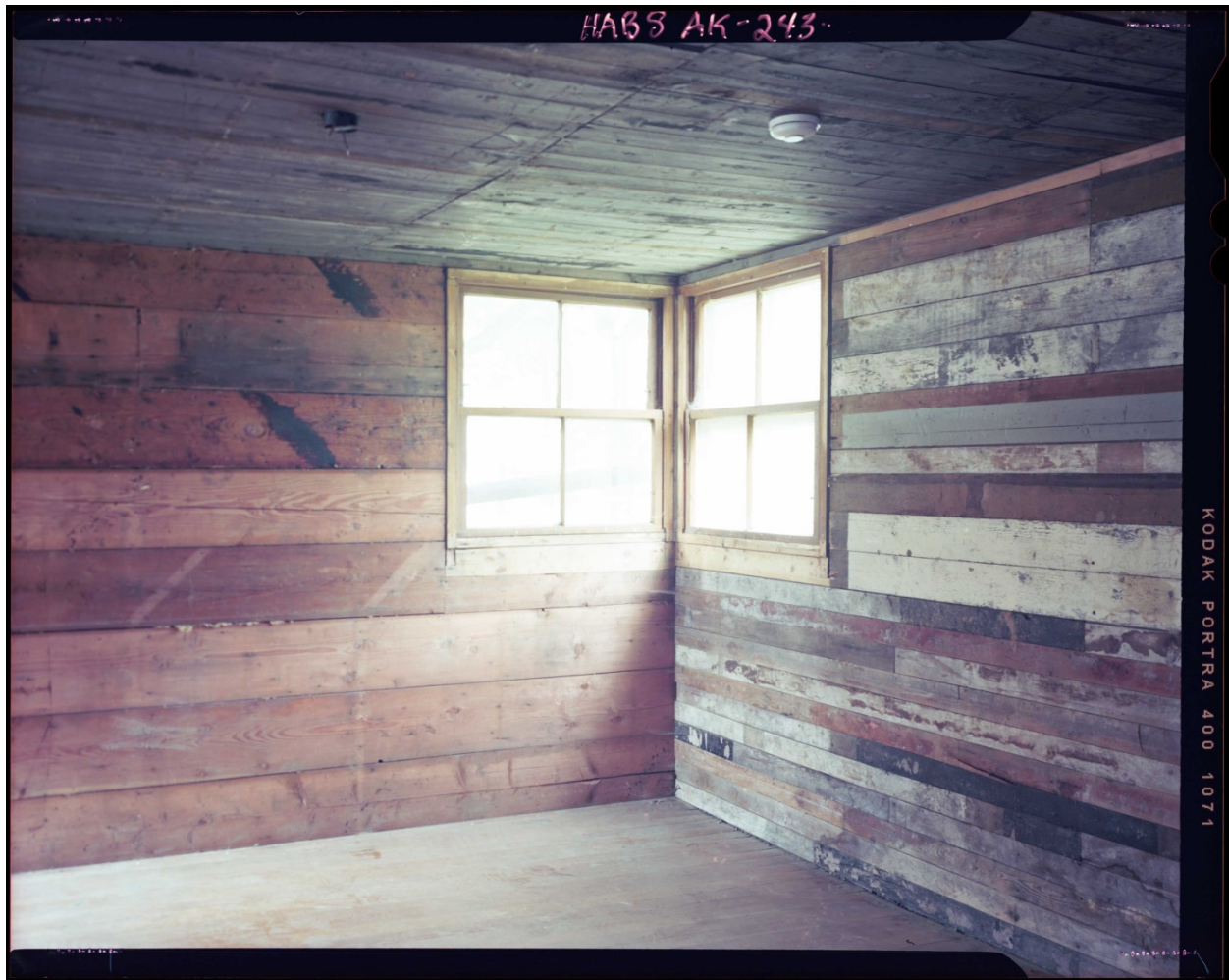
Fig. 7. North corner windows in bedroom. (Photographer: Robert Lyon, 2015)
