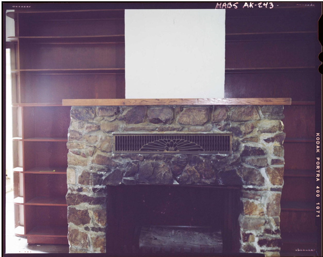
Fig. 3. Detail of fireplace grille. (Photographer: Robert Lyon, 2015)
