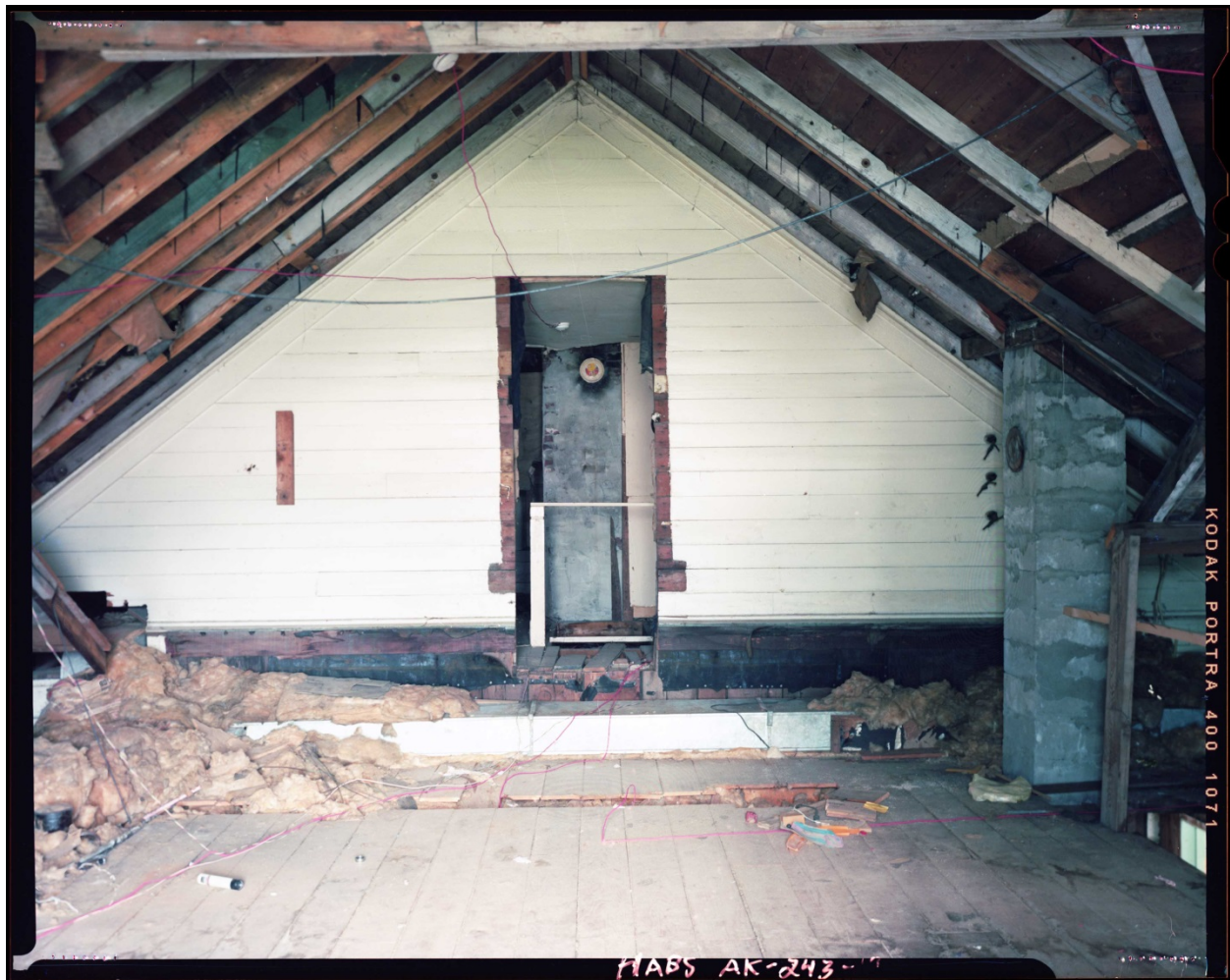
Fig. 8. Rear attic space looking southwest to gable end of original building. Original window cut to door opening. (Photographer: Robert Lyon, 2015)
