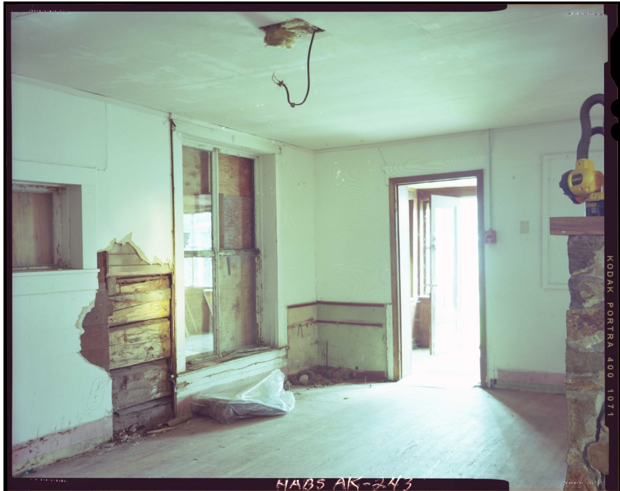
Fig. 1. Living room looking east to entry porch. Interior wall finish exposed to show heavy log construction. (Photographer: Robert Lyon, 2015)
