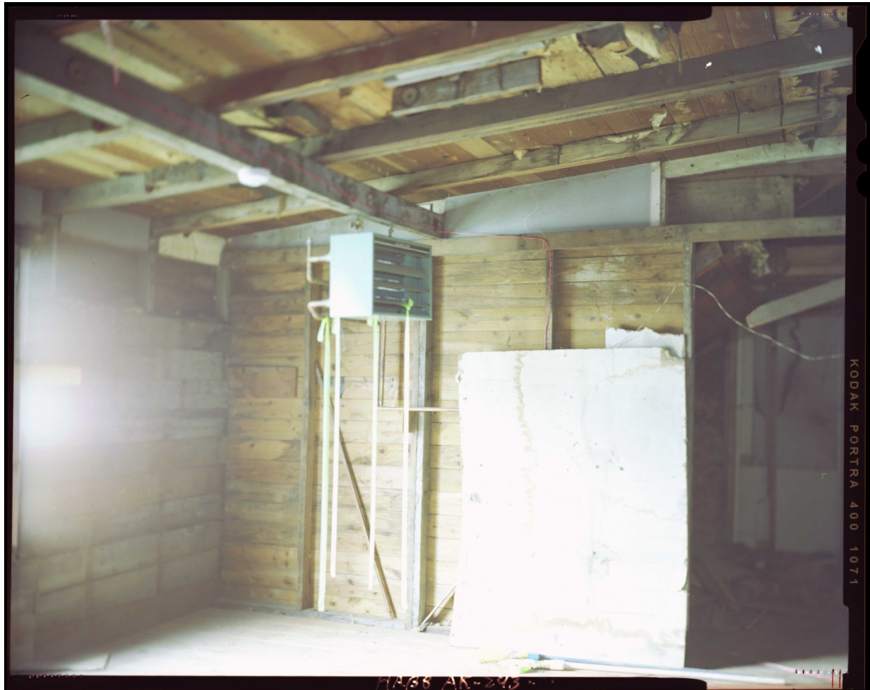
Fig. 9. Rear attic space looking east. (Photographer: Robert Lyon, 2015)
