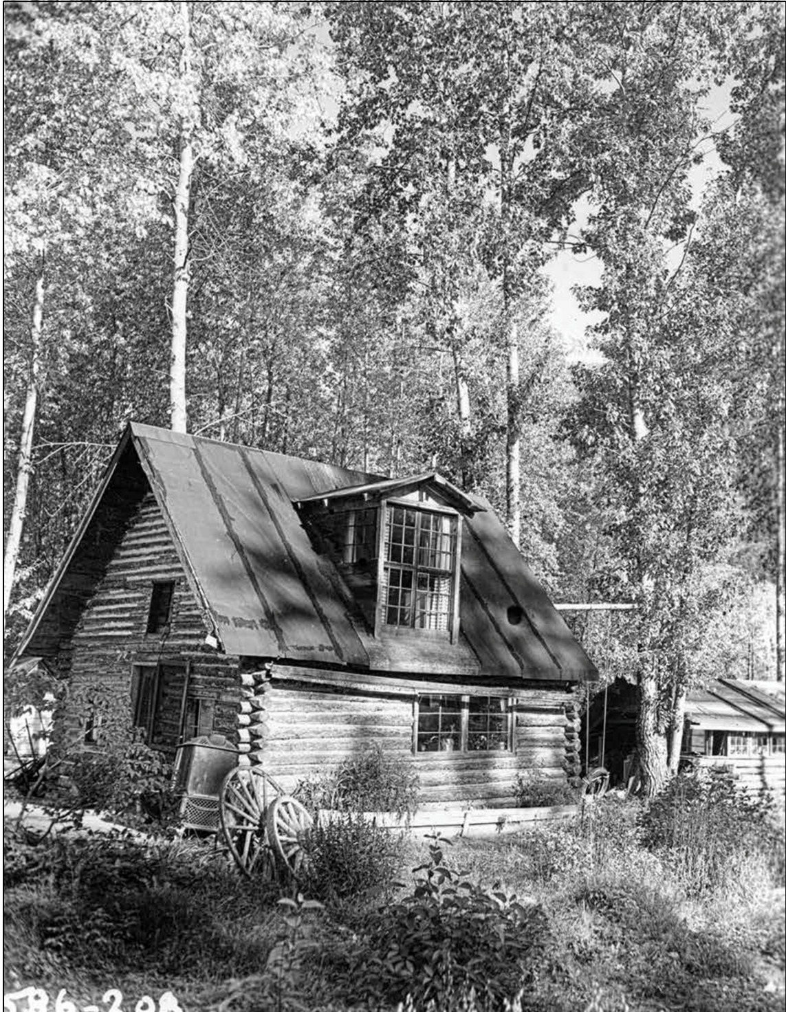
Figure 3: Patterson-McDermott Cabin showing Patterson era gambled dormer Source: Patterson Cabin, north and west elevations (586-208), photograph by Hunter Gruening, September 1952, National Park Service (NPS), KLGO Digital Library, Courtesy of Steve Hites Collection
