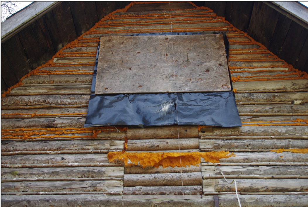
Figure 5: Gable peak of north elevation showing barked and peeled logs Source: Field photograph by Kathleen Wackrow, NPS, April 2016, NPS, AKRO, Historic Architecture, Patterson Cabin Digital Files IMGP6021
