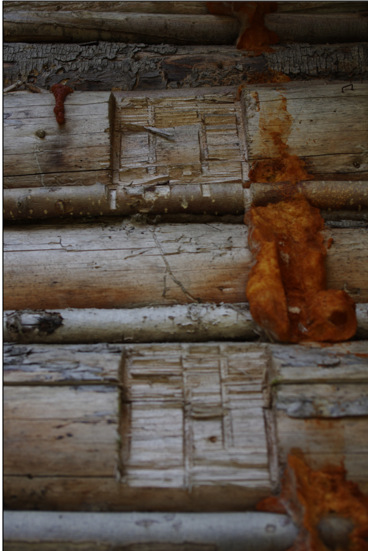
Figure 6: Signs of former shed-roofed kitchen addition from McDermott era along north elevation
