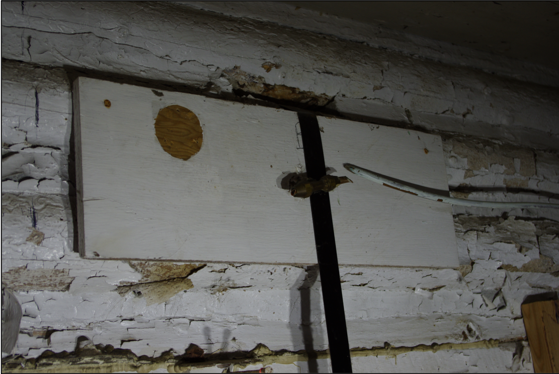
Figure 16: Rough-sawn wood board affixed to the east wall above the window. The circular marking on the left end of the board indicates where the base of a propane lantern was once attached
