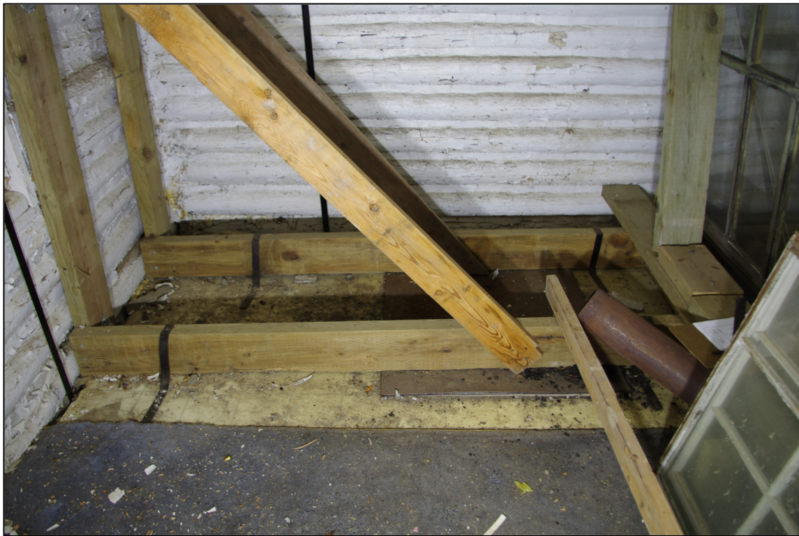
Figure 13: Interior southeast corner of first floor showing blue carpet, linoleum, and stove pad Source: Field photograph by Kathleen Wackrow, NPS, April 2016, NPS, AKRO, Historic Architecture, Patterson Cabin Digital Files IMGP6176
