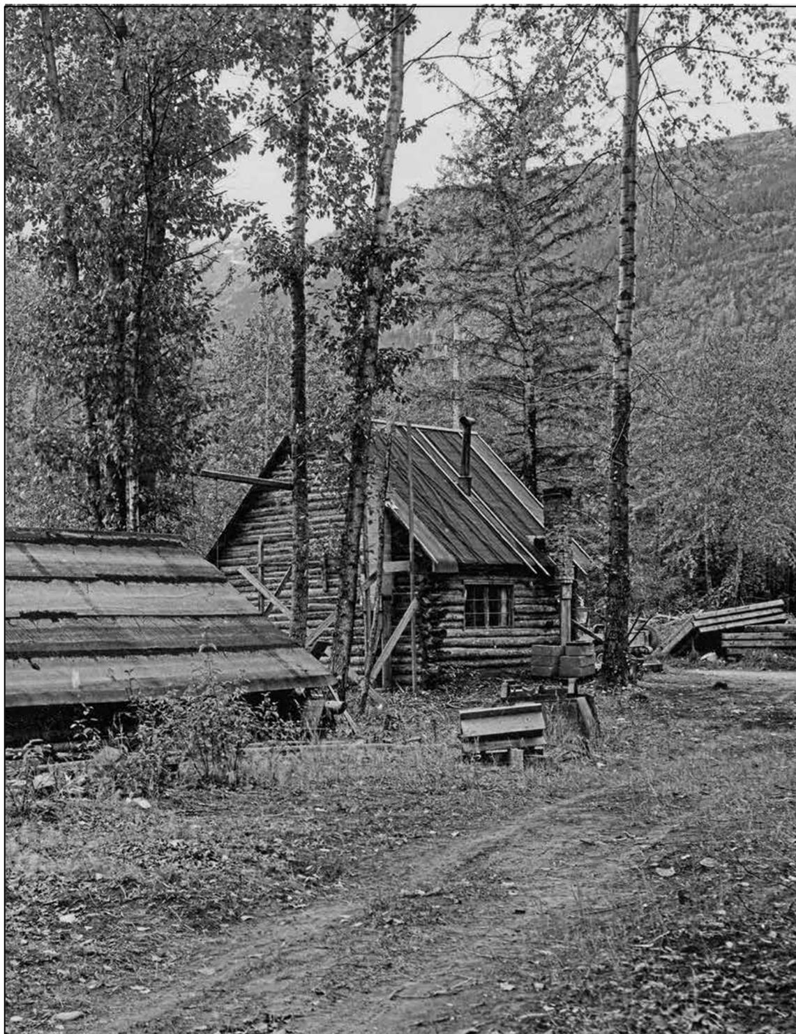
Figure 9: South and east elevations of Patterson-McDermott Cabin, showing no longer extant chimney
