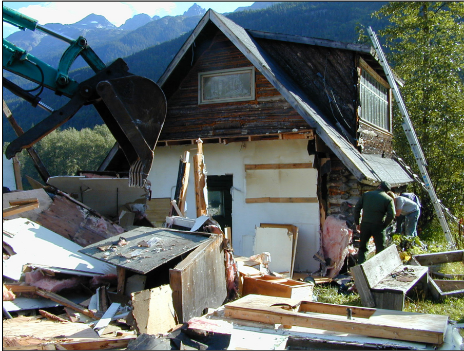
Figure 4: Patterson-McDermott Cabin relocation showing removal of kitchen addition Source: Unknown Photographer, NPS Staff Photo, September 2002, NPS, Alaska Regional Office (AKRO), Historic Architecture, Patterson Cabin Digital Files
