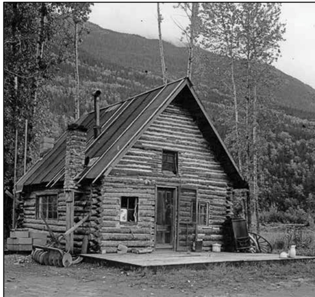
Figure 8: North and east elevations of Patterson-McDermott Cabin, showing no longer extant chimney
