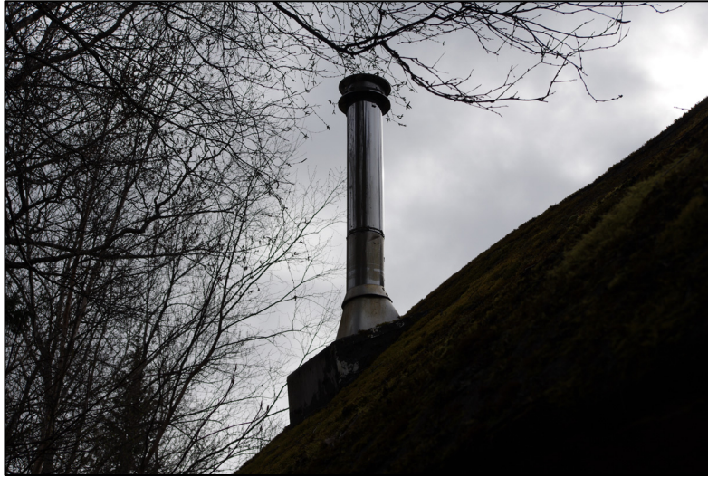
Figure 7: Insulated metal stove pipe from McDermott era Source: Field photograph by Kathleen Wackrow, NPS, April 2016, NPS, AKRO, Historic Architecture, Patterson Cabin Digital Files IMGP6068
