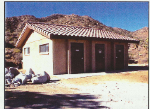
Completed Black Rock Campground Restroom
