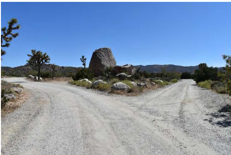
Intersection of the main (at left) and secondary loop roads (at right), facing southwest (North Wind 2020). The staging area is visible to the left of the boulder in the center of the photograph and the secondary loop road is visible at right.
