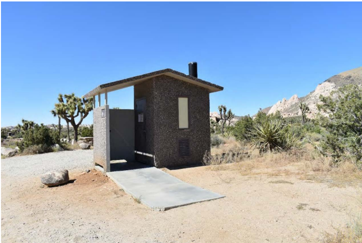
Typical one-vault toilet at Ryan Campground, facing northeast (North Wind 2020).
