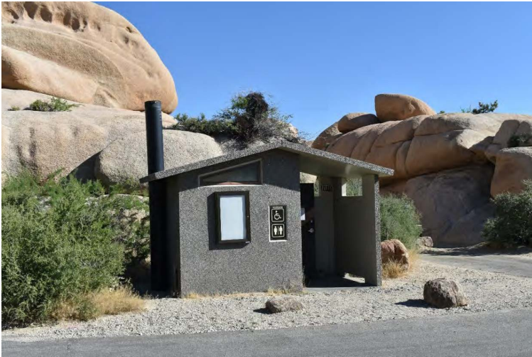
JR10, a single vault toilet at Jumbo Rocks Campground, facing north. Note the bulletin board in a locked case on the building's front (south) façade (North Wind 2020).
