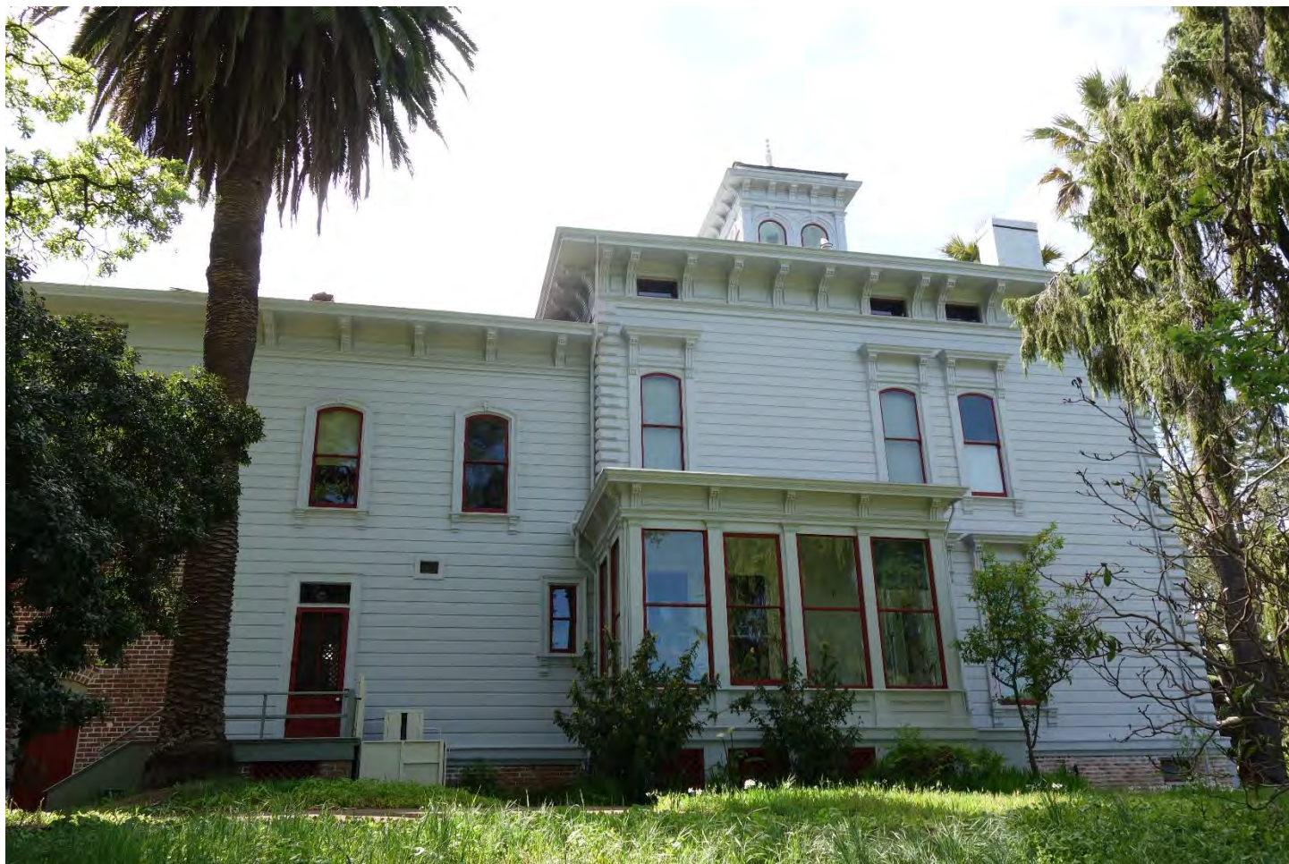
Photo 2: Strentzel-Muir House, east elevation. Camera facing west. Christopher E. Johnson, April 9, 2018.
