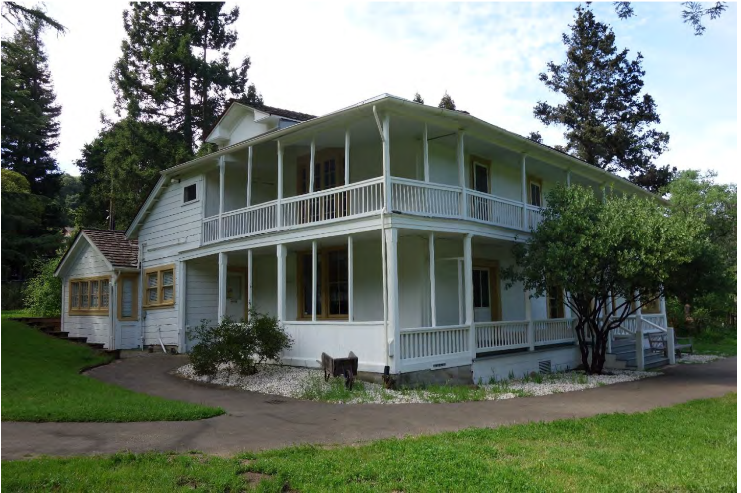
Photo 19: Martinez Adobe, east (front) and south elevations. Note the rear additions and the wrap-around two-story veranda. Camera facing northwest. Christopher E. Johnson, April 9, 2018.
