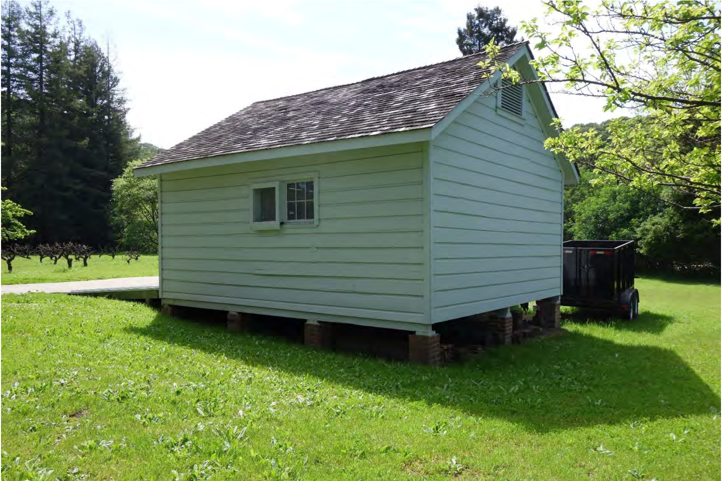
Photo 13: Carriage House, north (rear) and east elevations. Note the brick pier foundation. Camera facing west southwest. Christopher E. Johnson, April 9, 2018.
