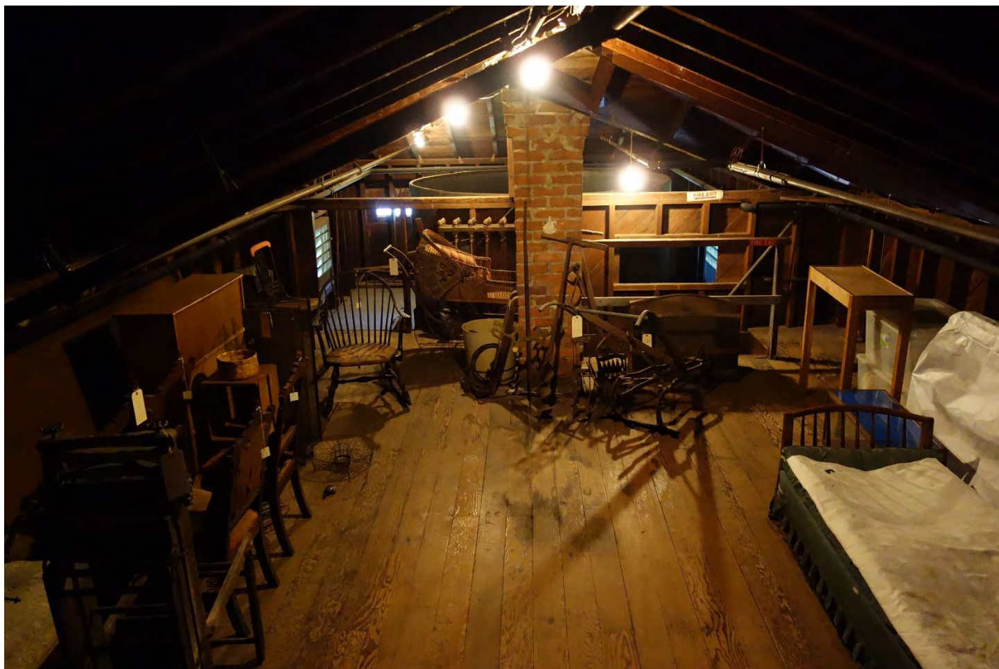
Photo 8: Water tank in the attic addition constructed by John Muir in 1890, camera facing south. Christopher E. Johnson, April 9, 2018.
