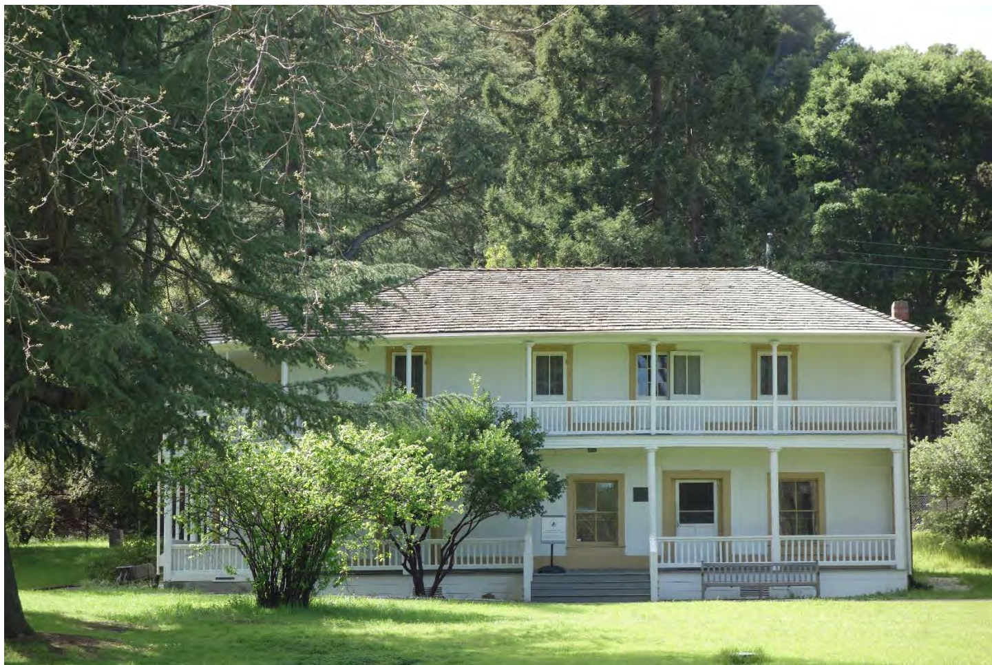
Photo 18: Martinez Adobe, east (front) elevation, camera facing west. Christopher E. Johnson, April 9, 2018.
