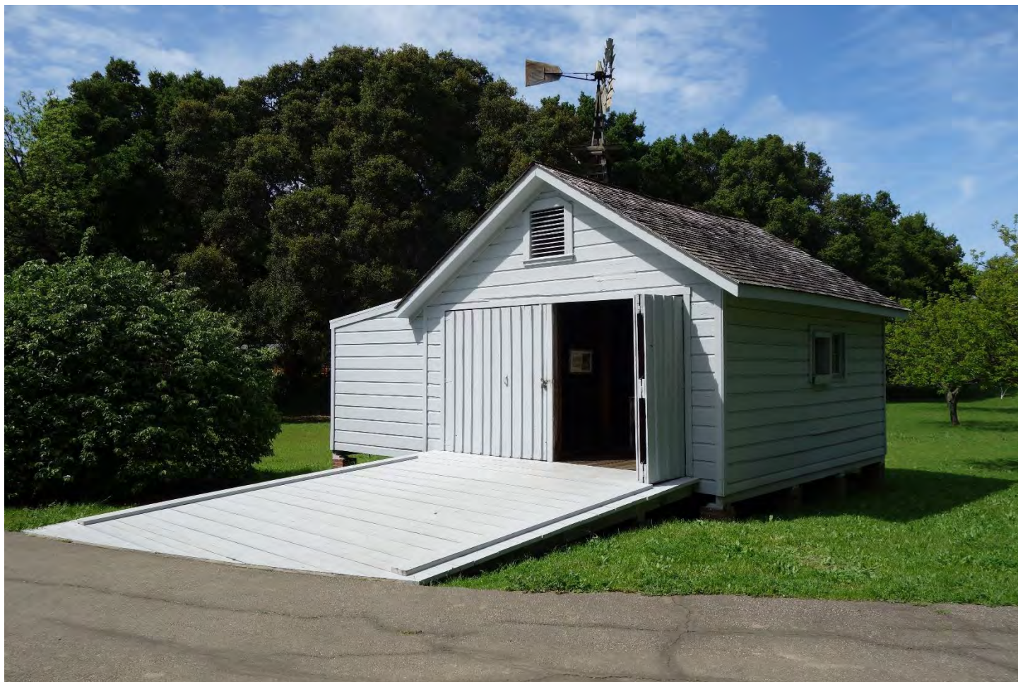
Photo 12: Carriage House, south (front) and east elevations, camera facing northwest. Christopher E. Johnson, April 9, 2018.
