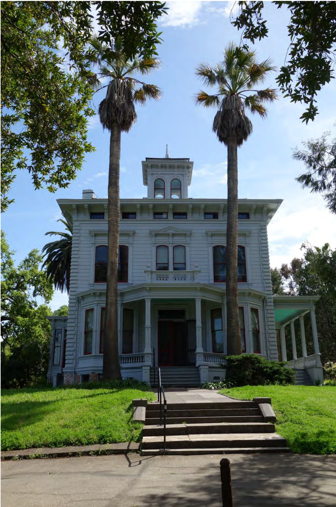
Photo 1: Strentzel-Muir House, front (north) elevation. Note the two California fan palms framing the entrance. Camera facing south. Christopher E. Johnson, April 9, 2018.
