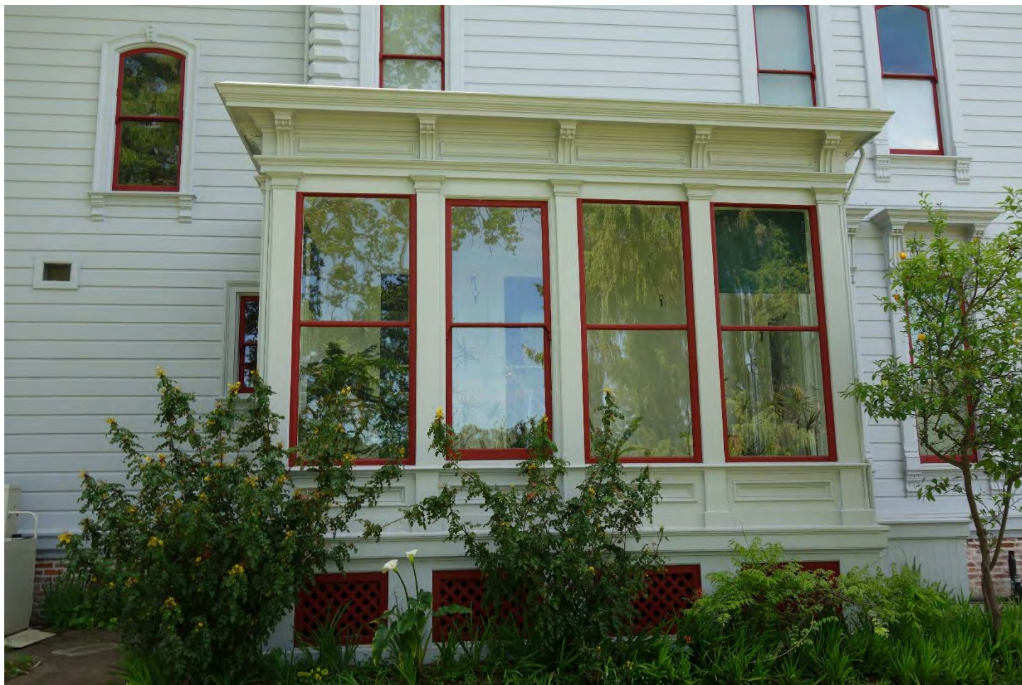
Photo 4: Strentzel-Muir House conservatory, camera facing west. Christopher E. Johnson, April 9, 2018.
