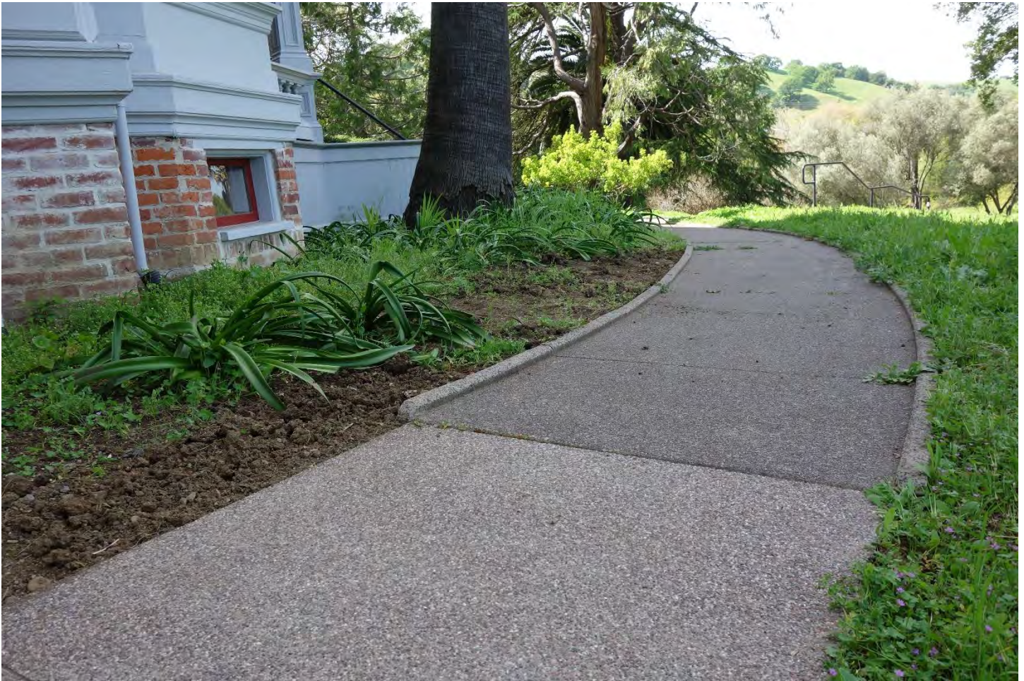
Photo 9: Strentzel-Muir House walkway with curbs on the northeast corner of the house, camera facing northwest. Christopher E. Johnson, April 9, 2018.
